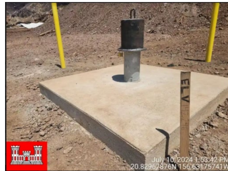
Figure 3. Groundwater monitoring well MW-02.
