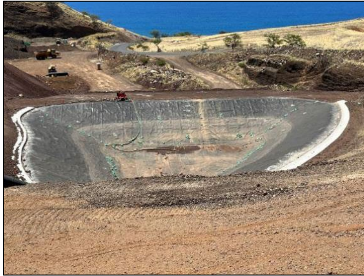
Figure 5 — Leachate Basin Adjacent to Ash and Debris Storage Area
