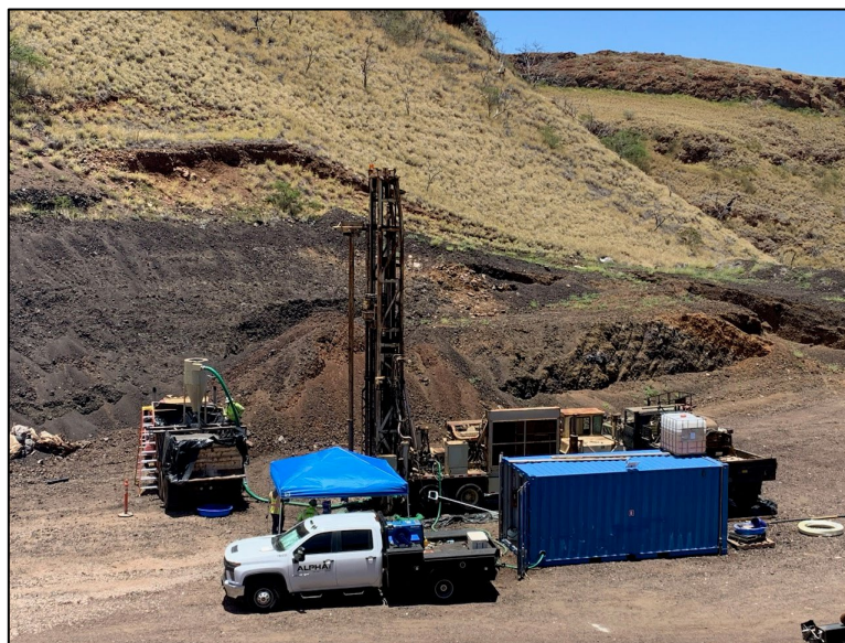
Figure 7 — Drill Rig Installing Groundwater Monitoring Well at TDS Site
