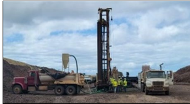
Figure 3. Groundwater monitoring well installation.
