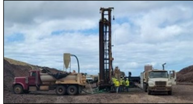
Figure 3. Groundwater monitoring well installation.
