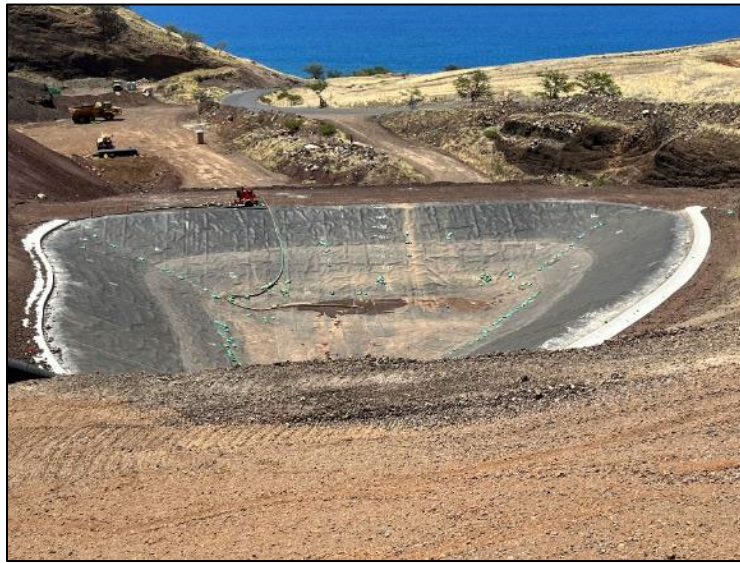
Figure 7 — Leachate Basin Adjacent to Ash and Debris Storage Area
