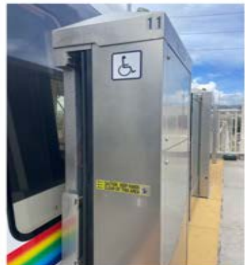
Signage at gates with tactile warning strips on ground
