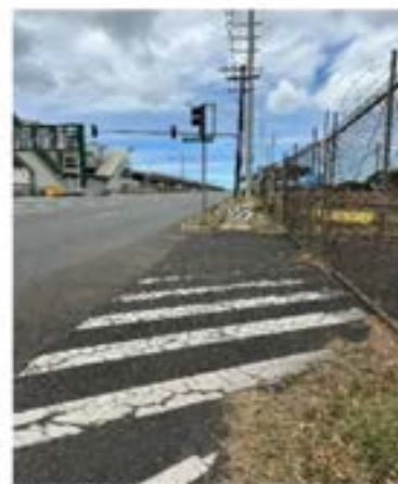
Uneven cracked sidewalk (Kalauao Station)
