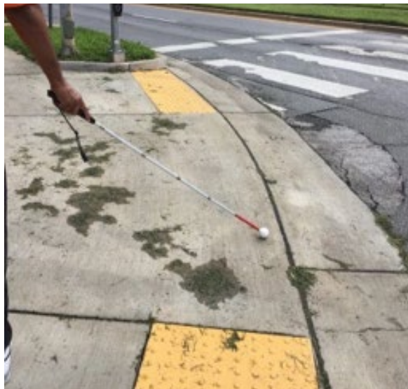
Figure 37: Example of curb ramp that is not aligned with crosswalk.
