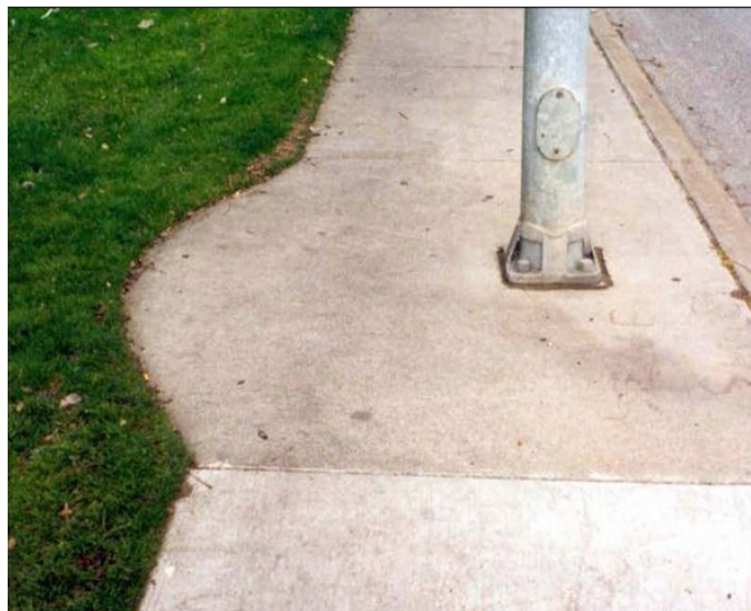
Figure 21: A shared use path splits around a utility pole. The wedge of grass provided is a non-prepared surface that may help people with vision disabilities navigate around the obstacle. Retroreflective edge lines could also be used to help define the correct path in this context.
