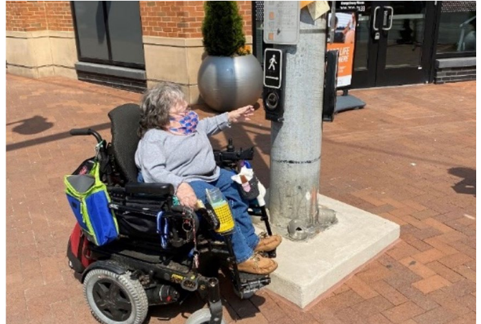
Figure 49: Person in wheelchair can't reach pedestrian push button due to large concrete base.
