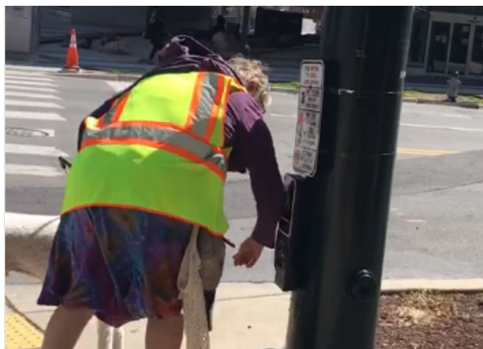
Figure 48: Person with guide dog having difficulty reaching a pedestrian push button that is too low
