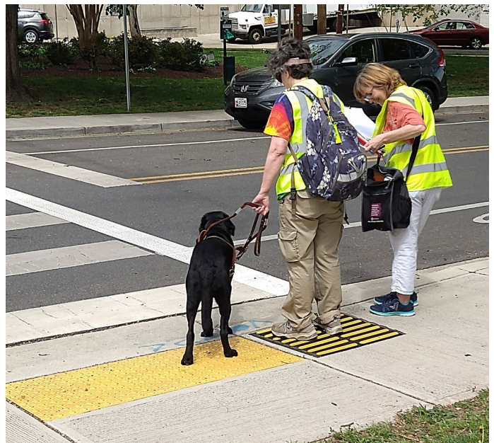
Figure 14: Alignment TDIs (shown at right of DWS) were tested as part of a pilot in downtown Silver Spring
