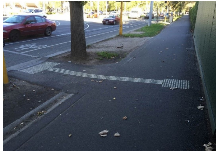
Figure 32: Example of tactile direction indicator used to guide pedestrians with vision disabilities to a midblock crosswalk in Melbourne, Australia. Note that the bars are not oriented as specified in this guide for sidewalk alert TDIs.
