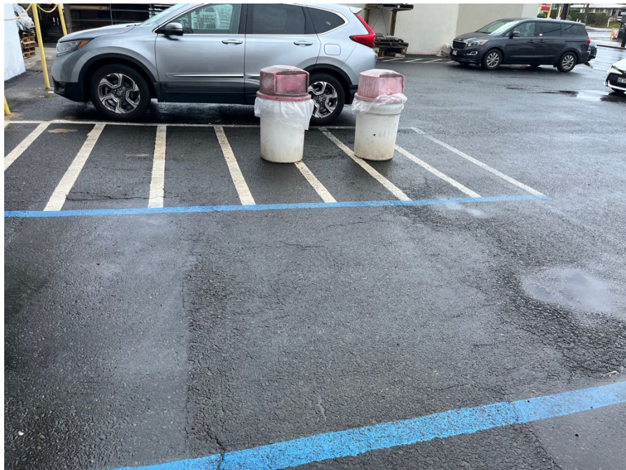
(Obstructions in access aisle)
