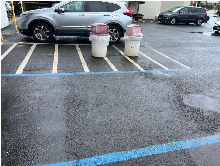
(Obstructions in access aisle)
