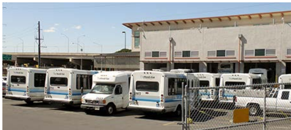
The Handi-Van base and maintenance yard on Middle Street has an estimated capacity to handle between 185-195 paratransit vehicles. The facility is nearing capacity with the current fleet of 181 Handi-Vans, with no room to expand.
