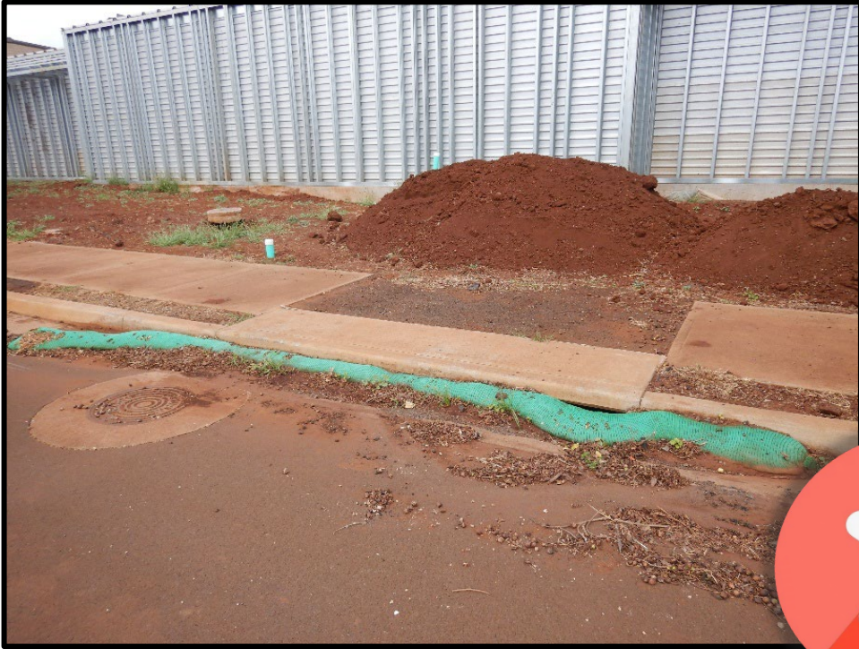
STORM DRAIN PROTECTION
