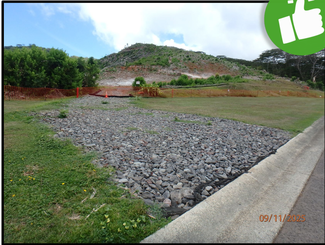
TRACK OUT CONTROL MEASURE
