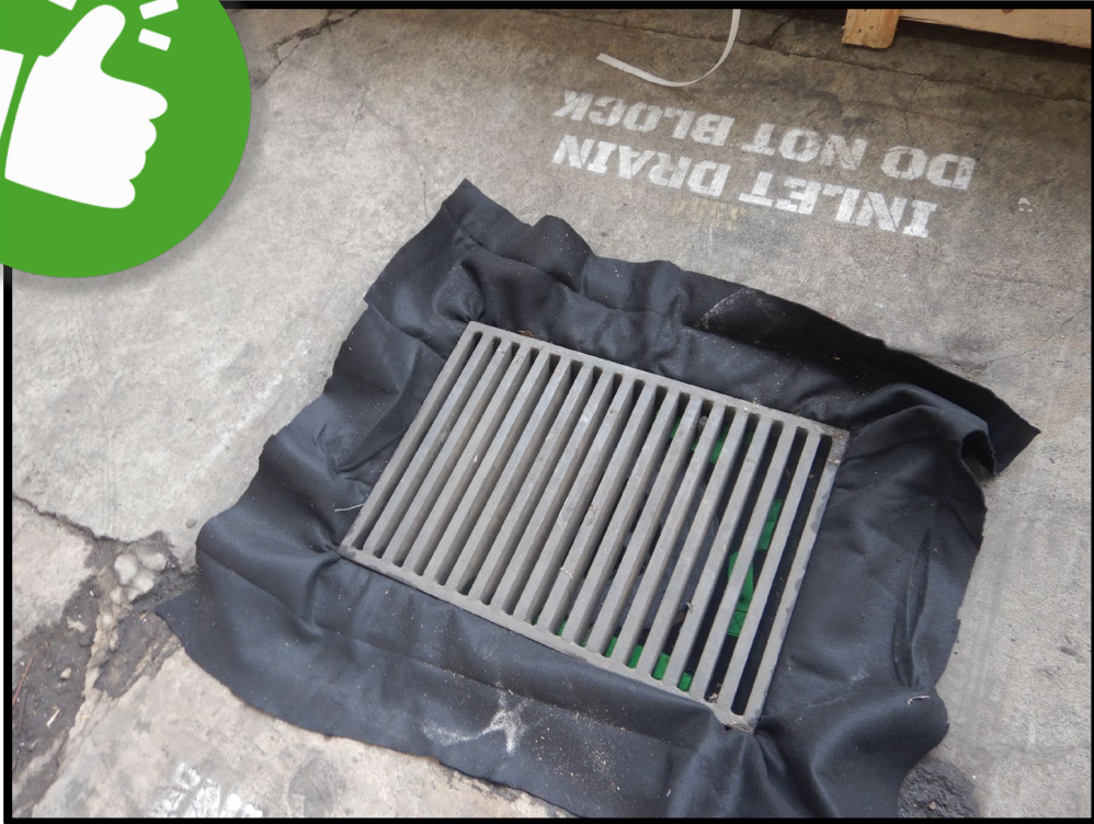
DRAIN INLET PROTECTION
