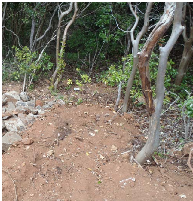
Figure 5.1 Road Push Pile on Side of Stream Bank
