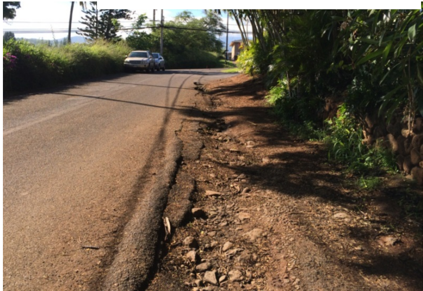
Figure 6.15 Lower Honoapiʻilani Road Shoulder Erosion
