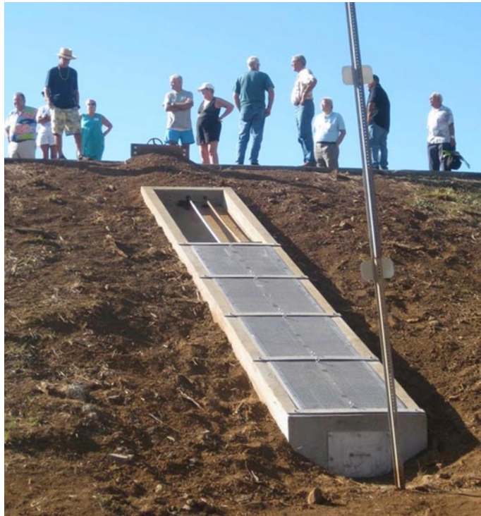
Figure 4.24 Nearly Completed Nāpili 4-5 Dam Outlet Valve
