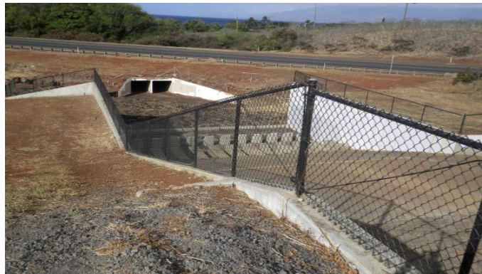
Figure 4.22 Ka'ōpala Desilting Basin Spillway Downstream Channel and Culverts
