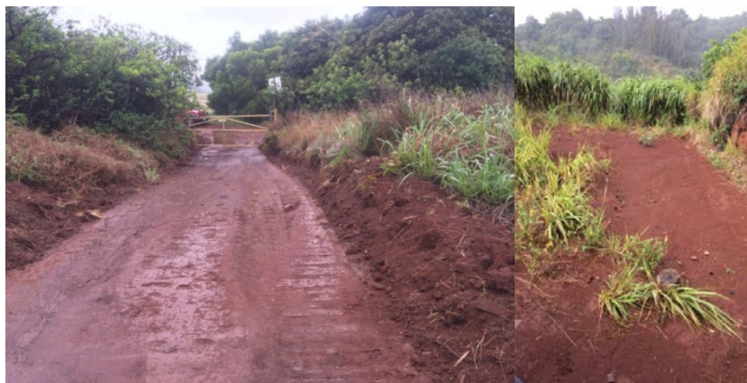
Figure 6.5 Maintained Road with Sediment Kickouts (Kahana Watershed – Zipline Access Road)
