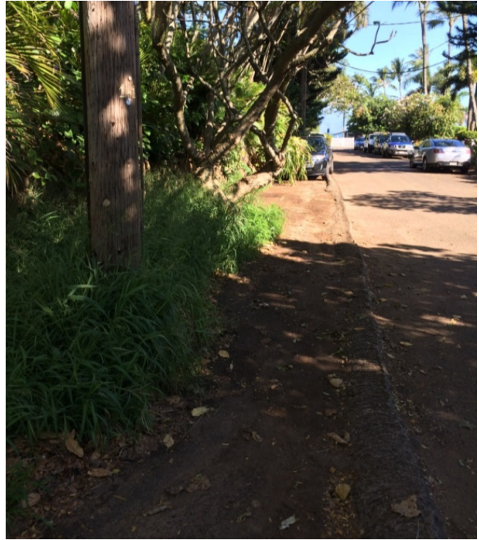
Figure 6.14 Nāpili Place Road Shoulder Erosion
