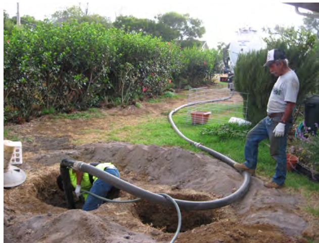
Pumping Septic Tank
