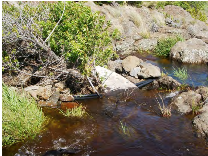
Diversion intake in Keanu‘i‘omanō Stream
