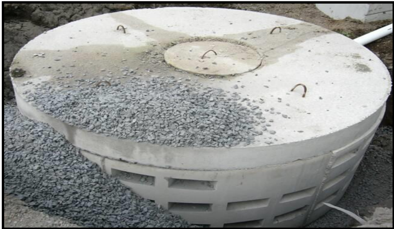
Figure 40. Stormwater Infiltration Well
