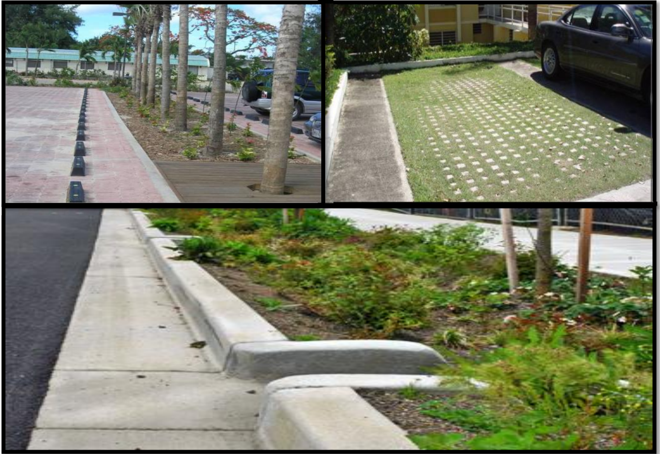
Figure 39. Examples of Low Impact Design Stormwater Treatment in Parking Lots
