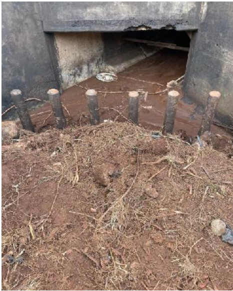
Soil and debris captured at bollards just mauka of the box culvert
