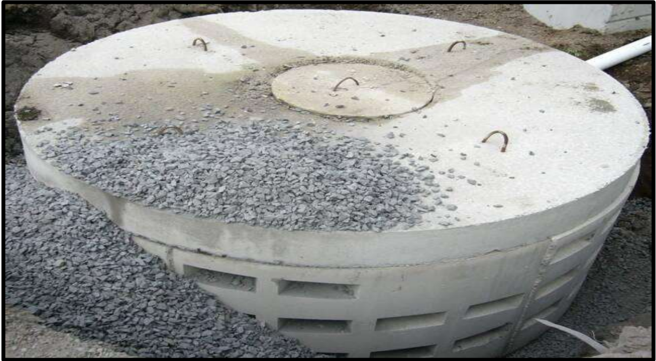
Figure 43. Stormwater Infiltration Well
