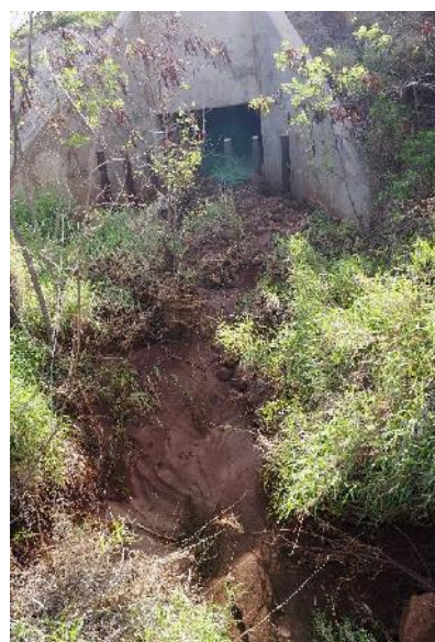
Evidence of sediment laden stormwater
