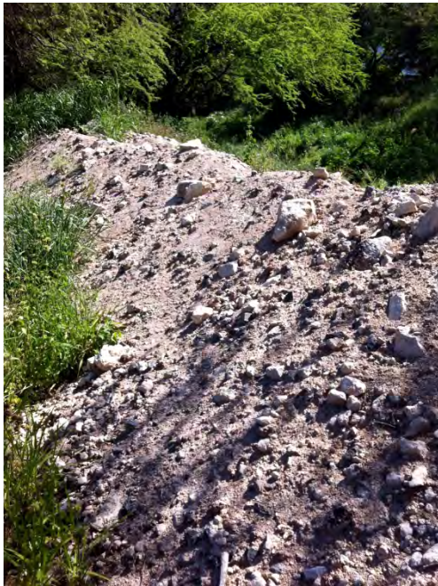
Photo 47. Berm protecting property makai of stream. Berm has failed in the past causing flooding.
