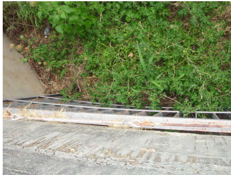
Photo 25. Grate covering makai side of bridge. Most likely for security purposes.
