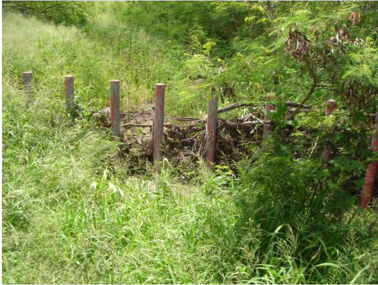
Photo 23. Upstream of a large bridge on Fence Rd. This is a debris catching fence.
