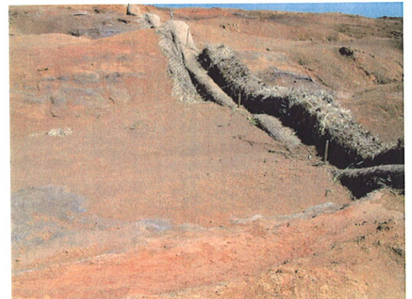
Figure 28. Pili roll and pili grass bales capturing sediment.
