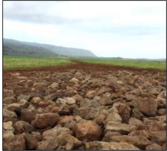
A strip of boulders at the entry/exit point of a field road on the Waialua DuPont-Pioneer property removes excess soil from the tires of field machinery
