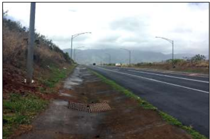
A portion of the State's MS4 along Joseph P. Leong Highway
