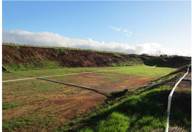
A sediment basin is designed to retain runoff, capturing significant amounts of sediment.
