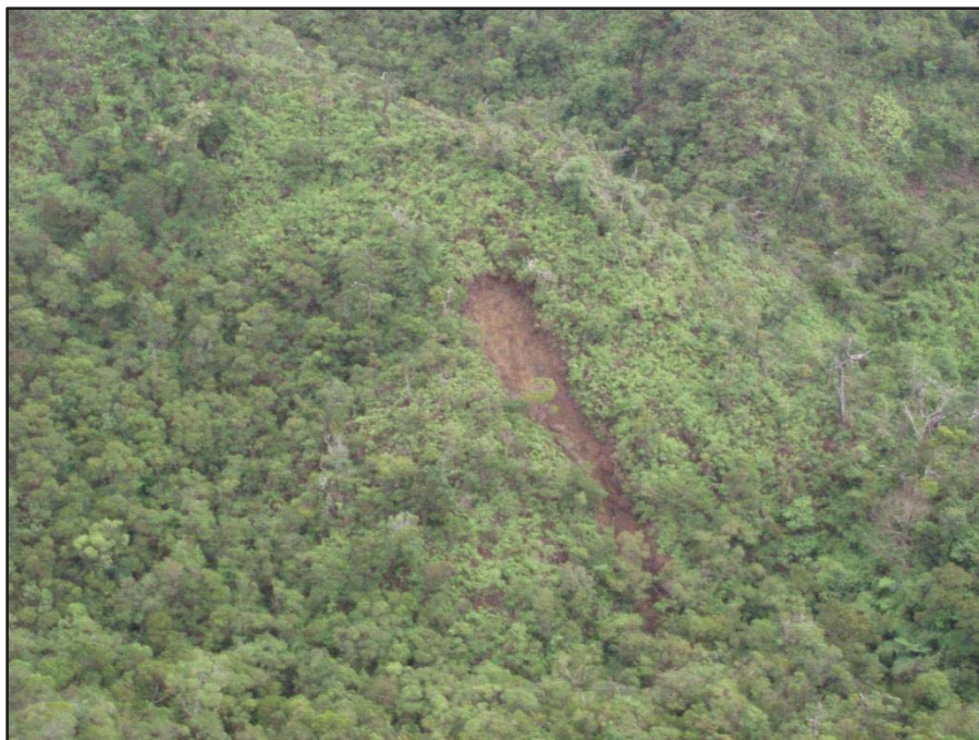
Photo B9: View of open slope debris slide in upper Kipapa Watershed.
