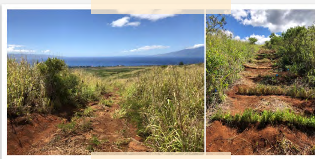
Restoration location before restoration began (on the left). Note the steep slopes and heavily gullied road. Photo on the right shows the road after it was cleared, prepped and BMPs were installed.
