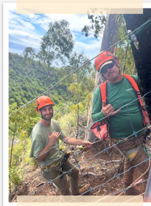
Crews use ropes to unroll and attach black mesh on the side slopes of Hanakao'o Valley.
