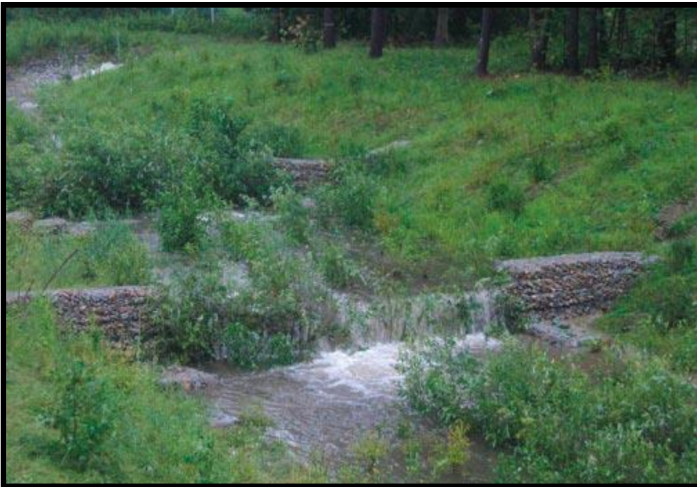
Figure 65. Image of Gabion Weirs in Series
