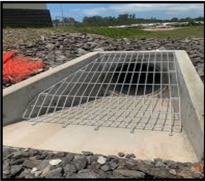
Figure 72. Culvert Protection from Debris
