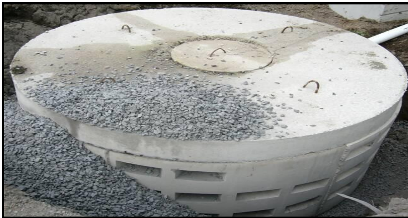
Figure 76. Stormwater Infiltration Well
