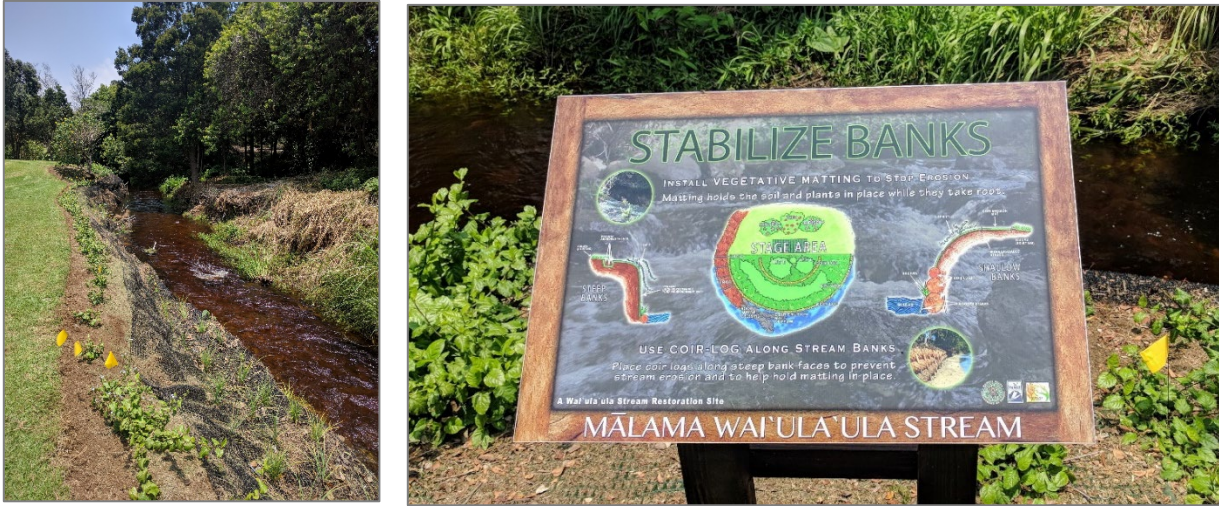
Figure 7. Streambank restoration in progress (left) and educational sign (right) funded as part of a Section 319-funded project, "Implementation of Best Management Practices in the Wai'ula'ula Watershed" (2014-2018), which was implemented by Hawai'i Sea Grant
