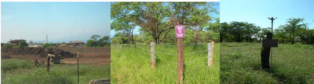
From left to right: Kibei Wastewater Reclamation Facility, Reclaimed Water sign; sprinkler head
