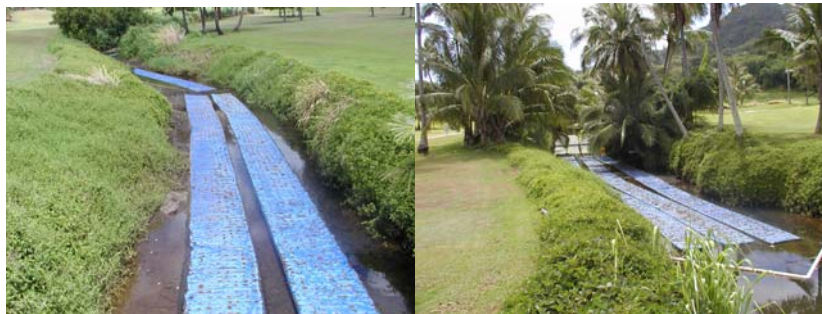
Photos of the platforms before the October storm event.
