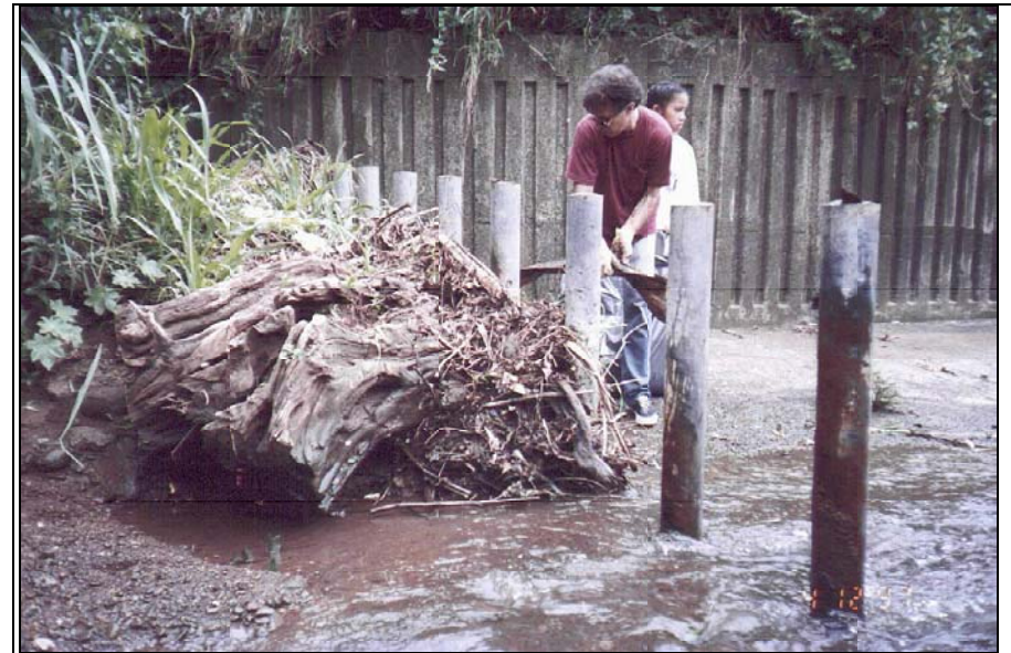
Figure 44. Large Stump Blocking Waiomao Stream (April 12, 1997). In 1996, City crews cleaned the channel (right side of photo) up to the debris barrier (posts), but did not remove the stump (left side of photo). It appeared to have been there a long time and has trapped sediment and debris. This channel-blockage may cause accelerated stream flows and erosion of the opposite stream bank. See next Figure also.
