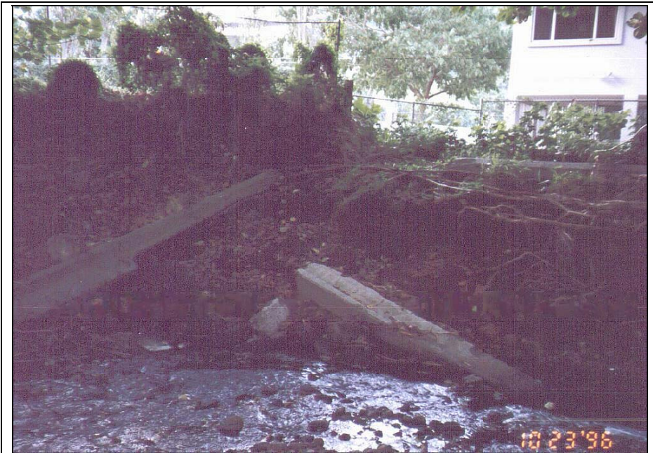
Figure 47. Failed Attempt at Stream Bank Erosion Control by Residents at Manoa Stream. Concrete foundation pile remnants about 16 inches in diameter and several feet long were used here as a retaining wall. They now appear to be in the floodway. This is the site of the proposed gabion retaining structures.
