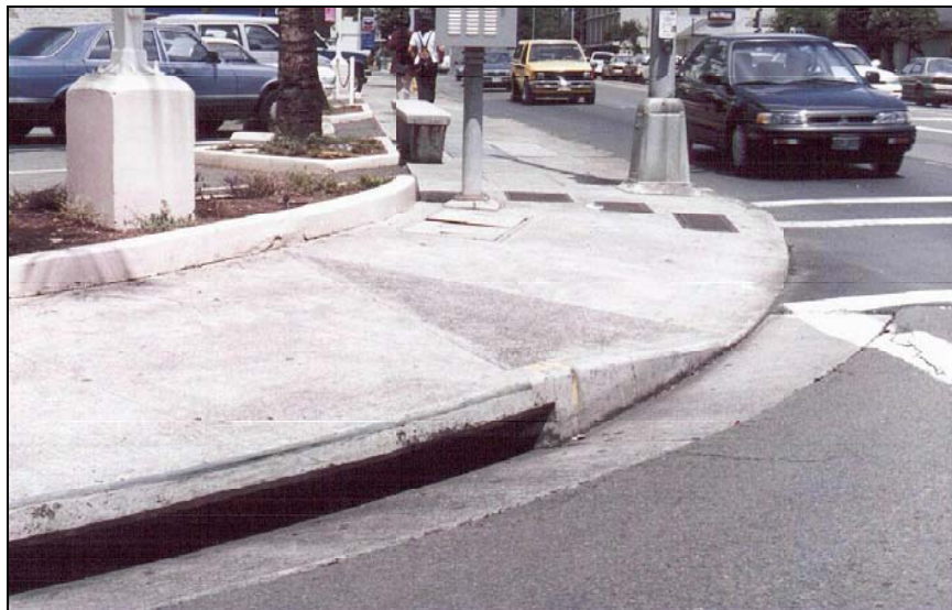
Figure 28. Storm Drain Inlet From Street to Catch Basin. Rain washes rubbish and contaminants from streets. Rubbish and contaminants collect in catch basins. From catch basins, storm water flows via pipes or culverts to streams and then to the Ala Wai Canal.
