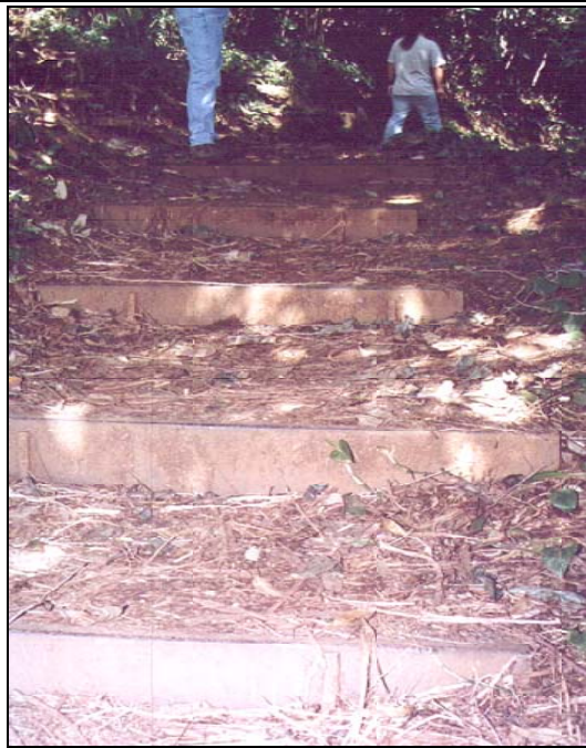
Figure 6. Erosion Control (1997) Using Recycled Plastic Planks, Manoa Falls Trail.
