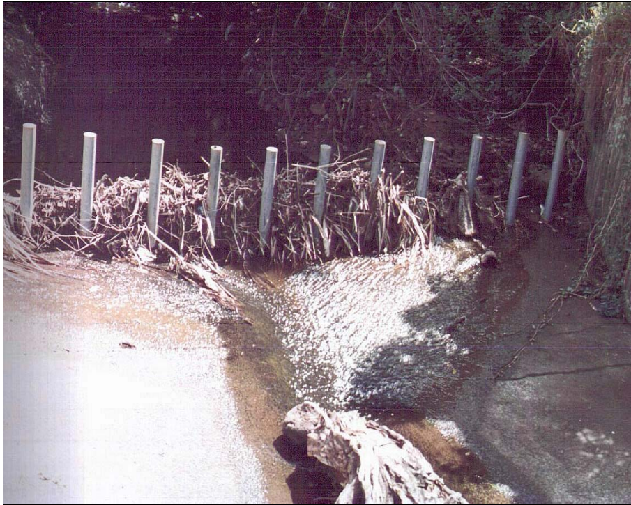
Figure 46. Stump Has Moved. In the previous Figure, the stump was on the other side, the upstream side, of the debris barrier. In this photo, the stump is on the down stream side. The stump was moved by high stream flows which occurred on October 11, 1997 and floated the stump up and over the debris barrier. DPW has been notified about this situation.
