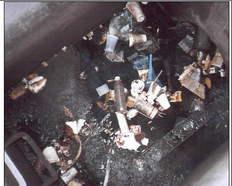
Figure 29. Typical Amount of Litter in Bottom of Storm Drain Catch Basin Under Kapahulu Avenue. Ladder rungs allow climbing down from manhole cover to remove rubbish shown in lower left corner of photo.
