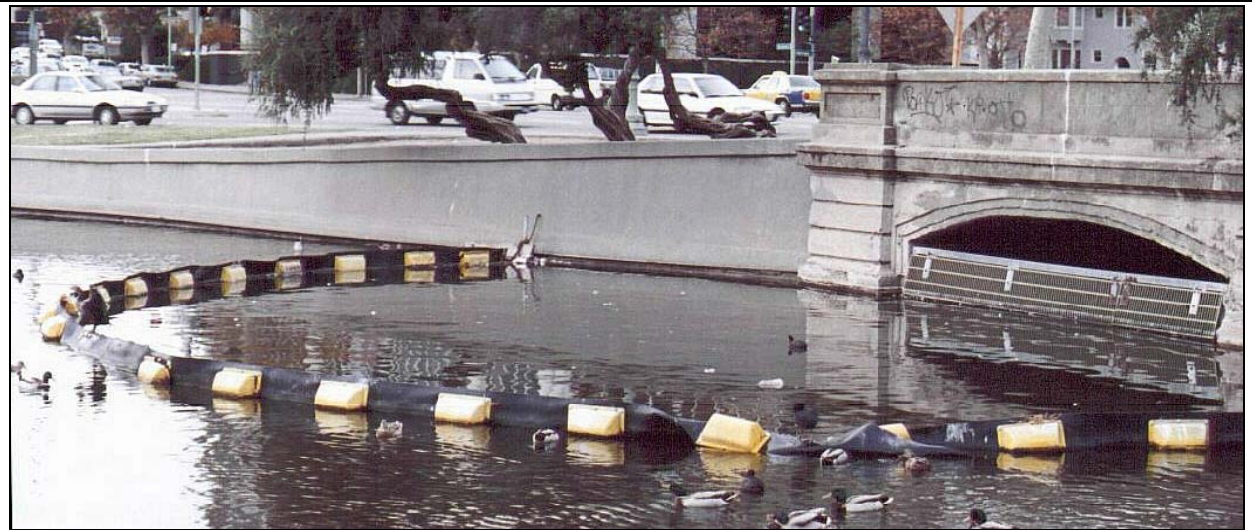
Figure 32. Debris-Catching Boom in Lake Merritt, Oakland, California. The boom captures debris originating on the land and transported via the storm drain outlet (right of photo) into the Lake.
