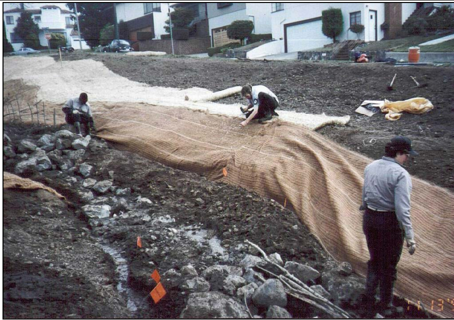
Figure 9. Stream Restoration in El Cerrito, Calif. This stream was in a pipe and paved over. The pipe was recently broken open so that the stream could be restored as an open waterway.
