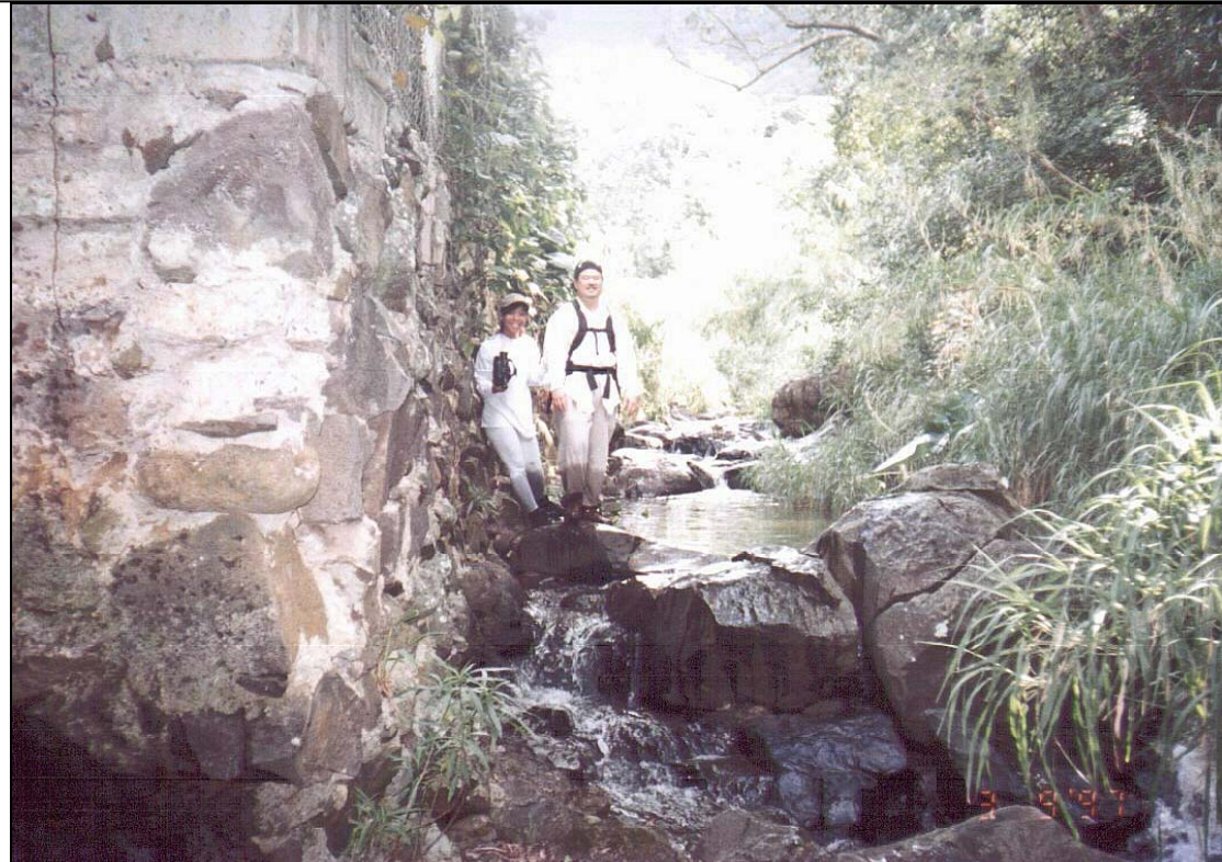
Figure 41. Retaining Wall. One of Several Retaining Walls in Pukele Stream, Adjacent to State Property (Anuenue School). Walls like this force higher stream flow levels and velocities which cause erosion of the banks on the opposite side of the stream. In this case, public historic properties (taro terraces - lo \square l) are endangered. Part of the problem is that stream ownership is split down the middle between property owners on either bank. In this case, government owns one half the stream. Where private property is owned on both sides of the stream, government has no property rights. Agencies need to develop policies to guide compliance because in such cases streams are not kept clean, nor will government maintain the privately held areas.
