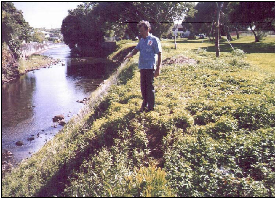
Figure 10. Manoa Playfield at Manoa Recreation Center. The entire length of stream bank along Manoa Stream adjacent to the recreation center is badly eroding. It should be cut back, landscaped and trees planted. A stream should be a key feature of parks. Instead, streams are treated as obstacles or problems and are fenced off from the community. Manoa Elementary School has adopted this area and is planting trees along the bank, with the help of City Parks staff. A memorandum by the Consent Decree Coordinator may have stopped the messy practice of mass herbiciding – which contributed to the erosion problem – but no action has been taken so far on stream bank restoration and erosion control.
