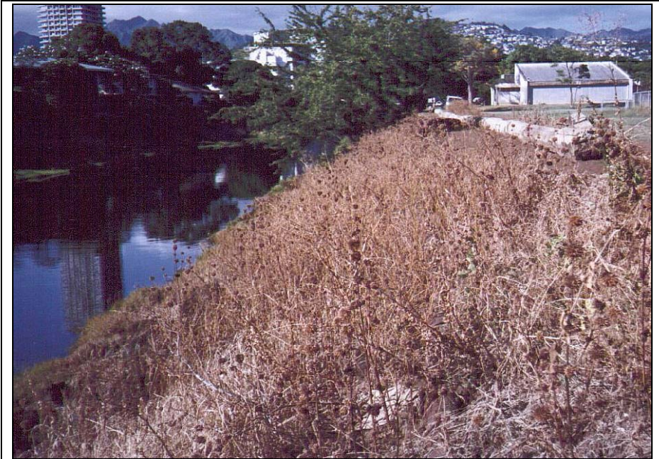
Figure 11. Kaimuki High School – Manoa-Palolo Canal. Proposed Start of Streambank Restoration and Bike Path from Date Street to Woodlawn Drive. This is the Manoa-Palolo Canal, next to Kaimuki High School. The bank should be cut back at a lesser slope, a trail/bike path cut into or on top of the bank, and trees and landscaping applied to stop soil erosion.
