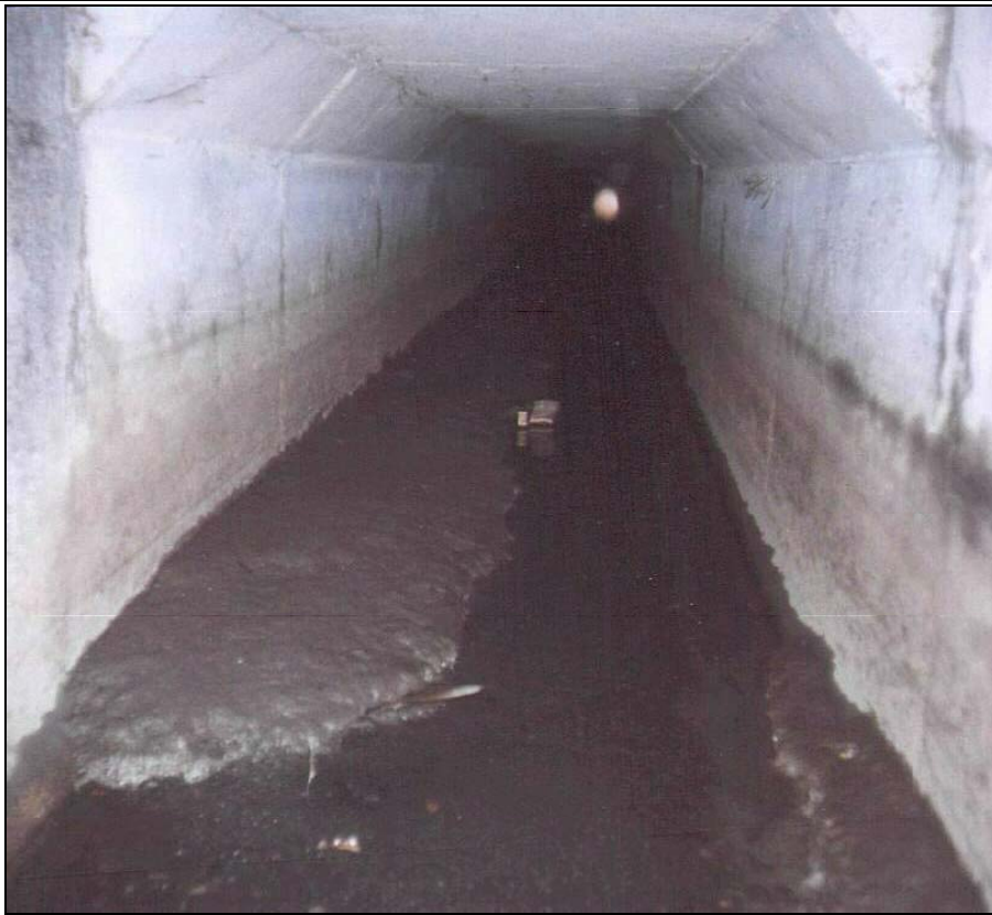
Figure 24. Accumulated Sediment in Storm Drain Under Kapahulu Ave. City Crews Remove This Material While Sliding, Face-Down, on Skateboards Because Drainpipe Is Only 2-Foot High.
