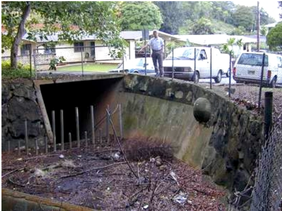
Figure 2.10: Drain inlet at the top of Lipalu Street in Pikoiloa subdivision
