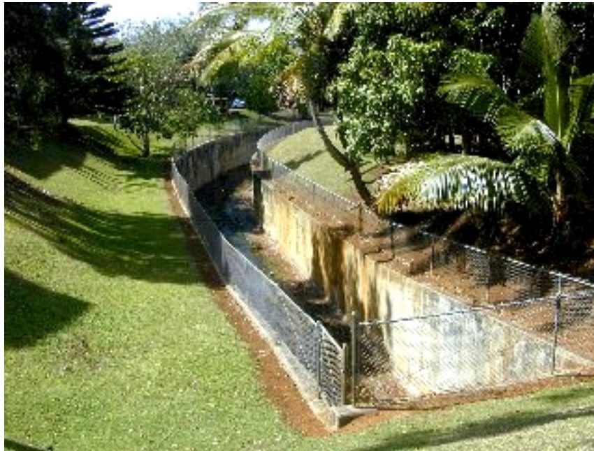
Figure 2.8: Concrete culvert along the lower portion of the Parkway subdivision
