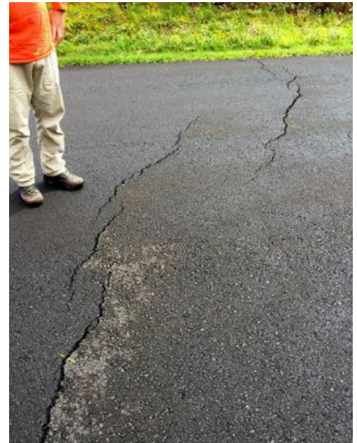
Cracks in road around Leilani Estates. Photo taken on 5/2/2018 courtesy of USGS.
