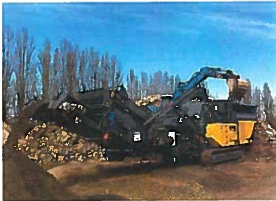
Rubble Master RM90 crusher with MS95 screen
