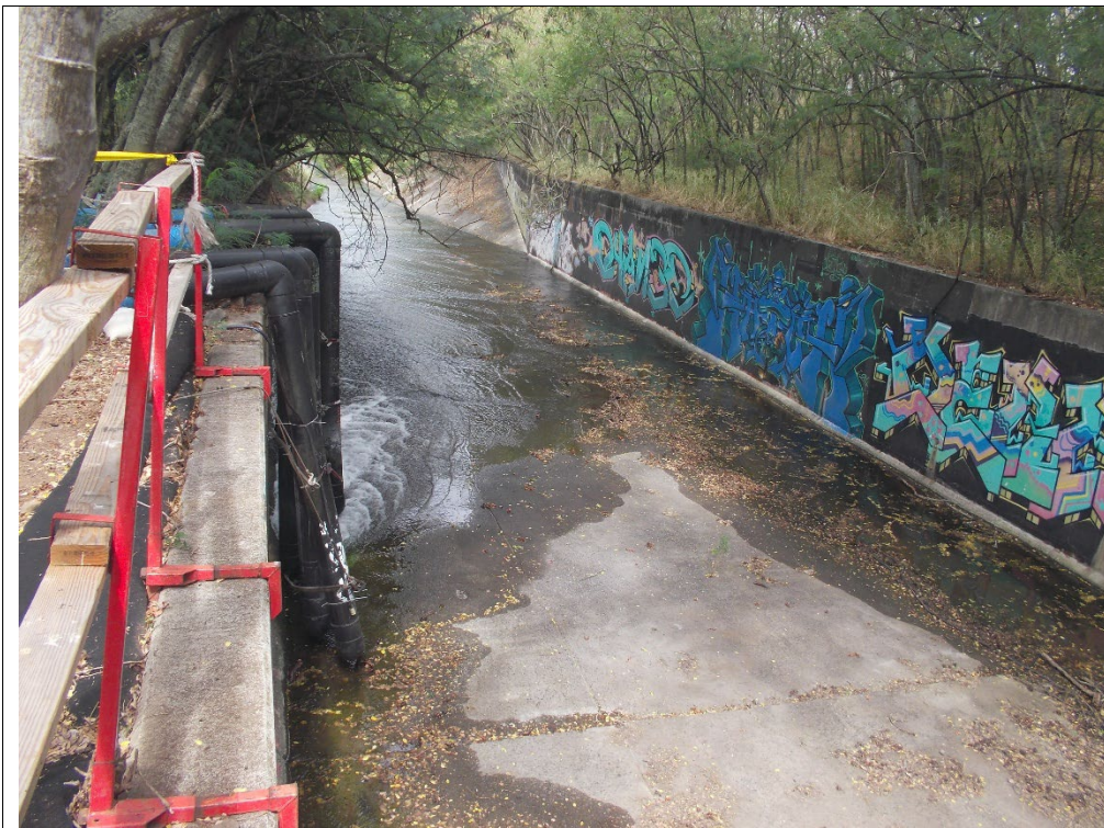
Photograph # 2: Discharge Site looking downstream.
