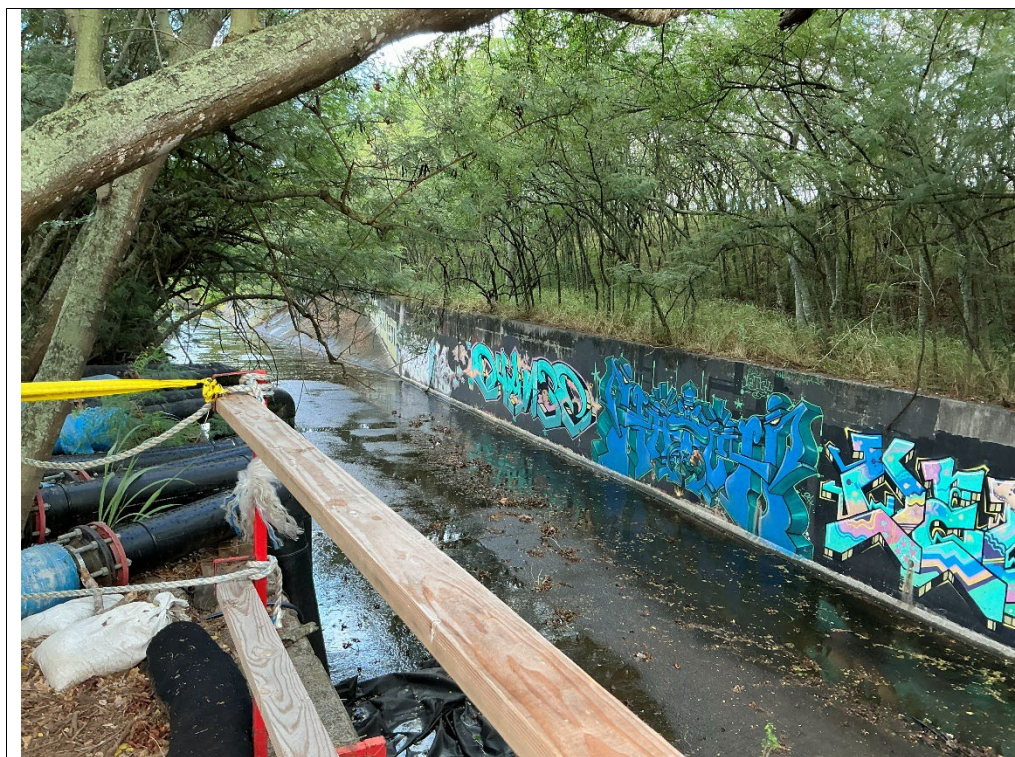
Photograph # 2: Discharge Site looking downstream.
