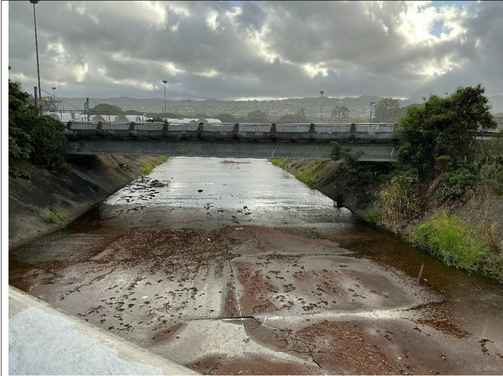
Photograph # 1: Downstream Site 1 looking upstream.
