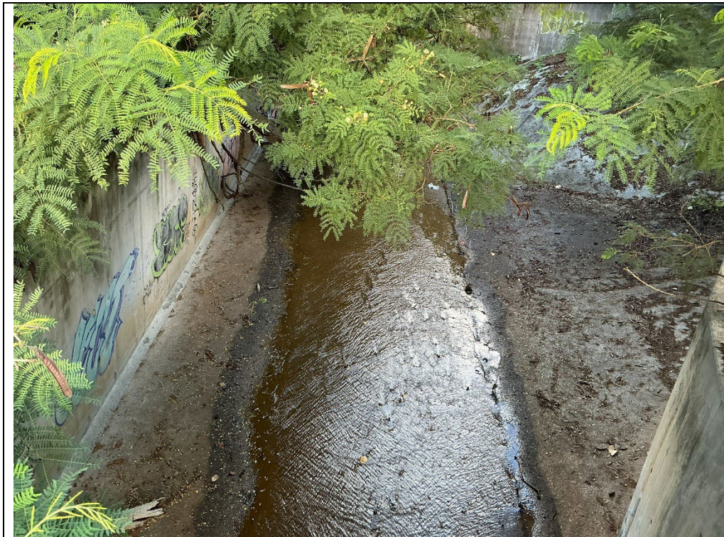
Photograph # 2: Upstream Site looking downstream.
