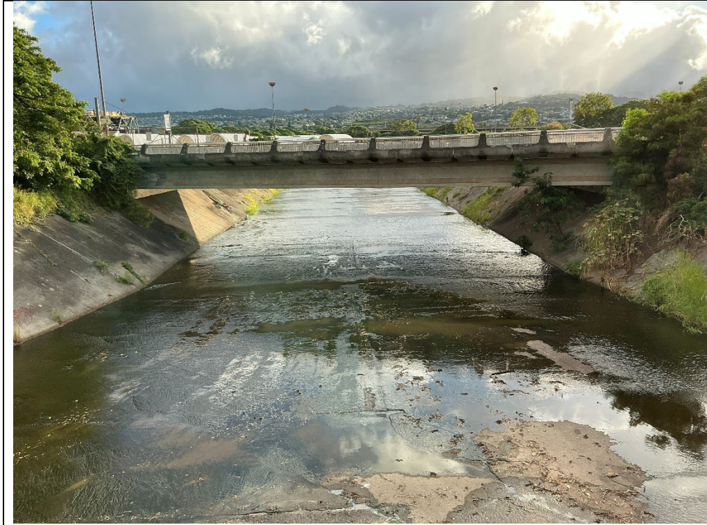
Photograph # 1: Downstream Site 1 looking upstream.
