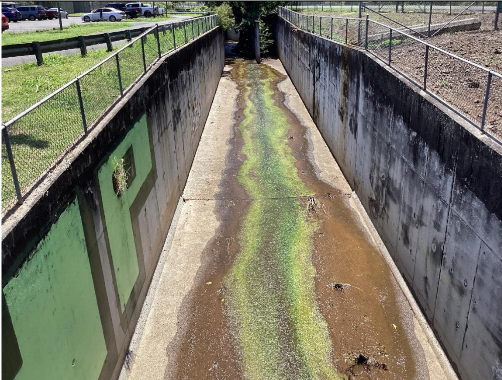
Photograph # 1: Upstream Site looking upstream.
