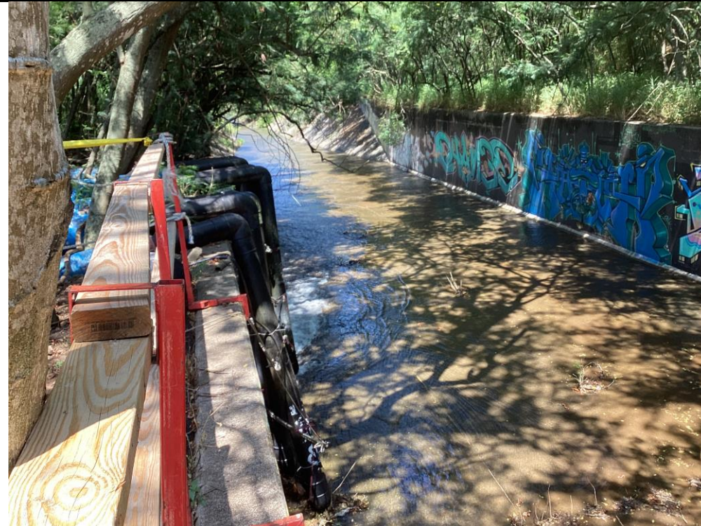
Photograph # 2: Discharge Site looking downstream.
