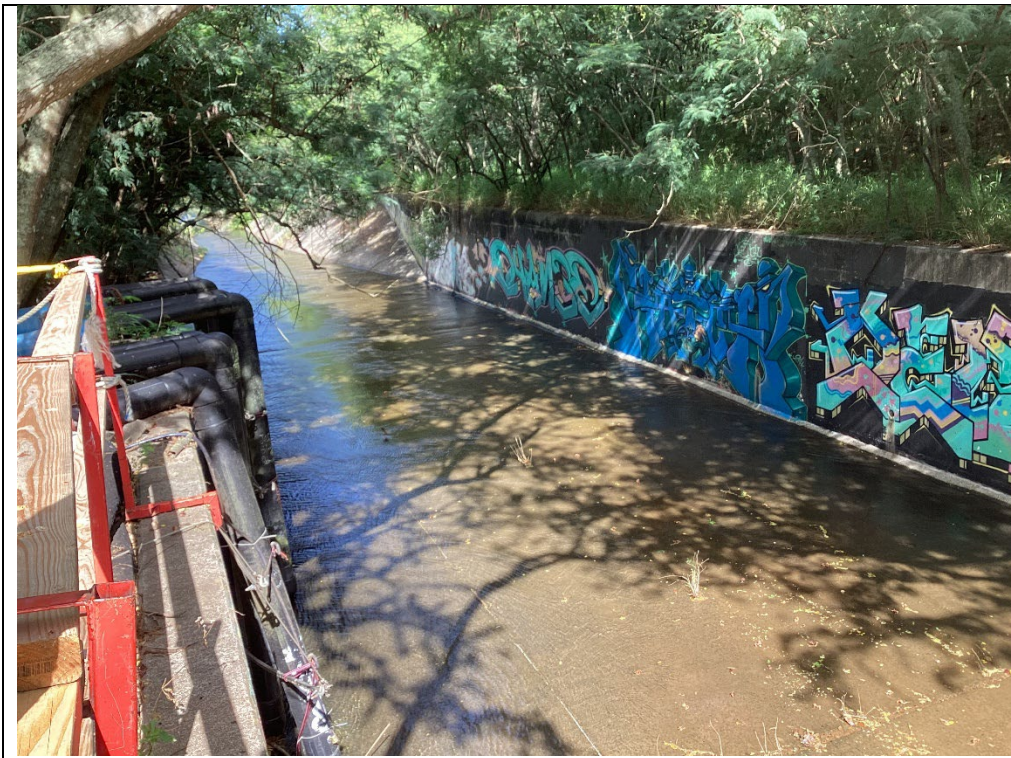
Photograph # 2: Discharge Site looking downstream.
