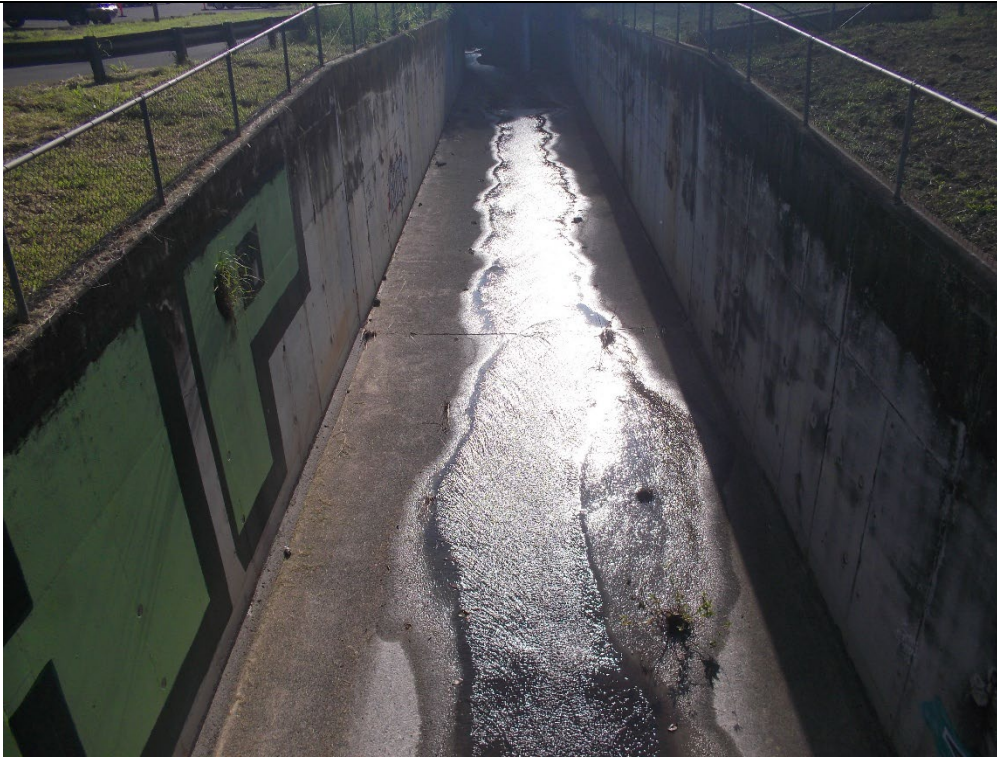
Photograph # 1: Upstream Site looking upstream.
