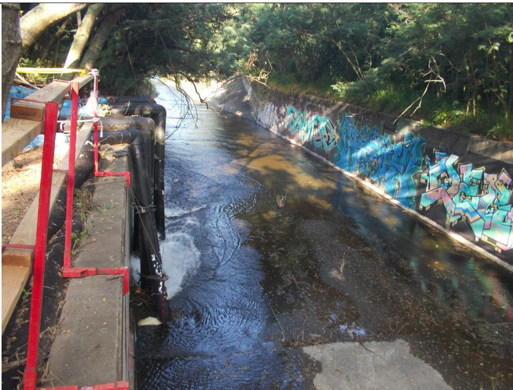
Photograph # 2: Discharge Site looking downstream.
