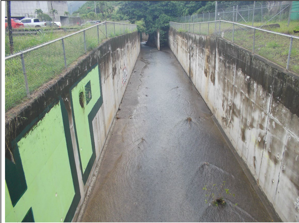
Photograph # 1: Upstream Site looking upstream.
