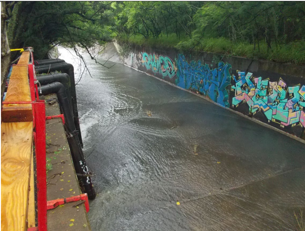
Photograph # 2: Discharge Site looking downstream.
