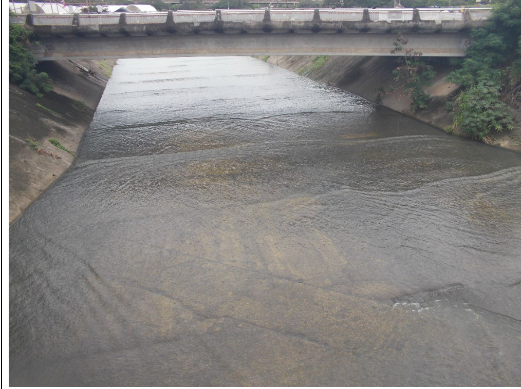
Photograph # 1: Downstream Site 1 looking upstream.
