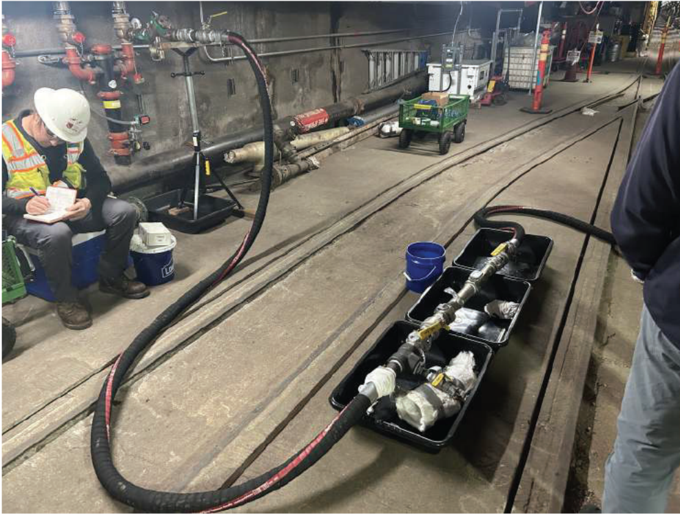
FOR line packed via fire protection water supply line at Main Sump.
