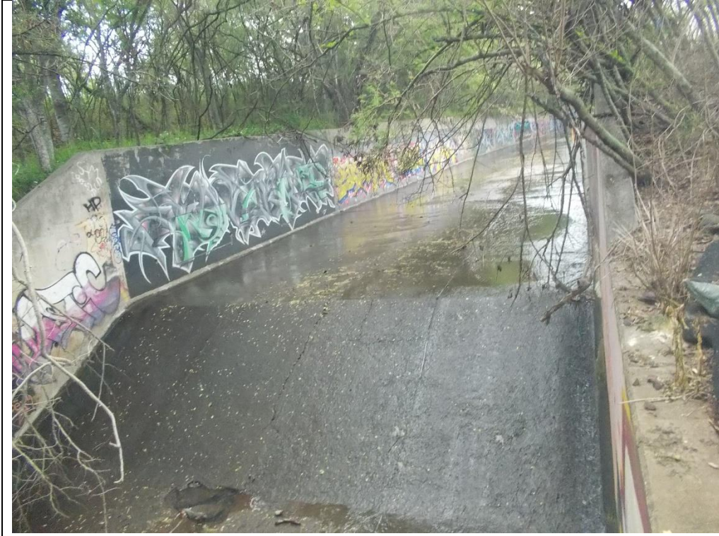
Photograph # 1: Downstream Site # 1.
