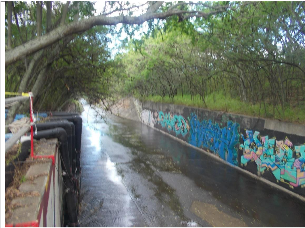
Photograph # 2: Downstream Site # 1.
