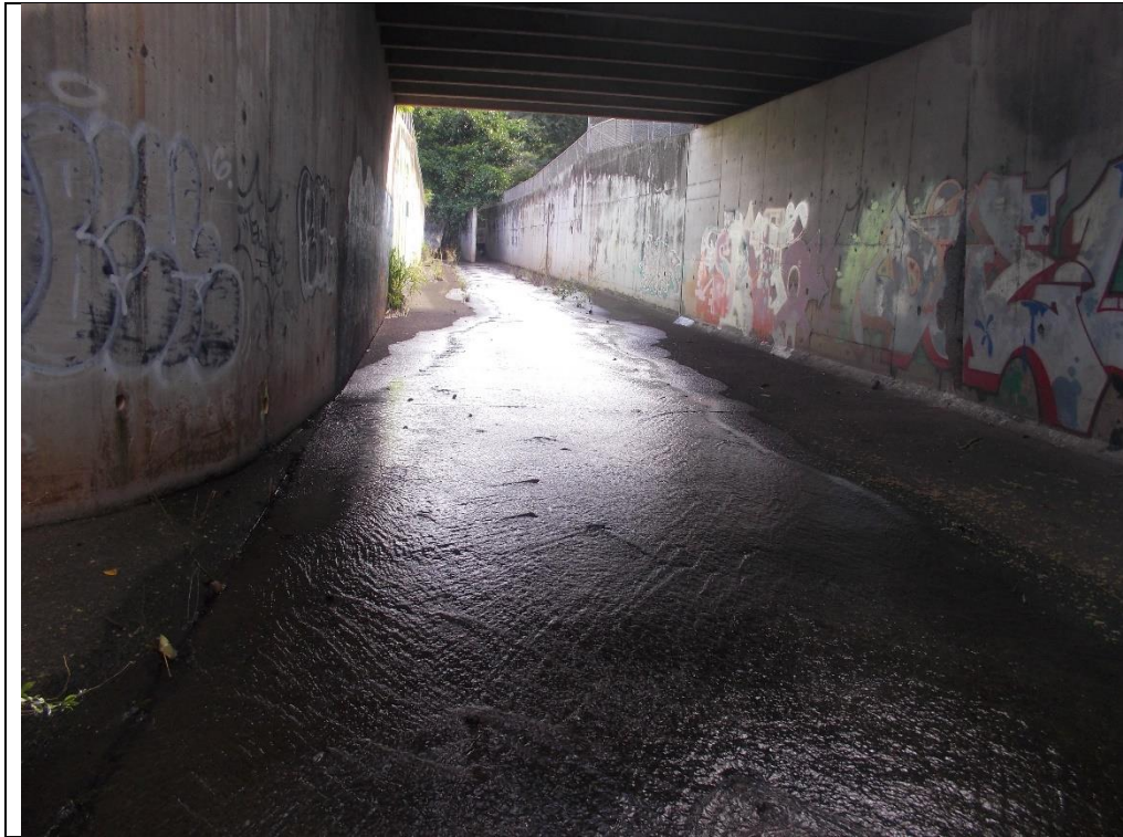
Photograph # 1: Upstream Site looking upstream.
