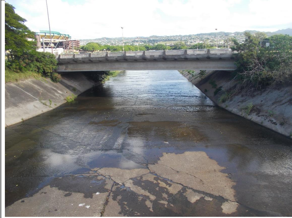
Photograph # 1: Downstream Site # 1.
