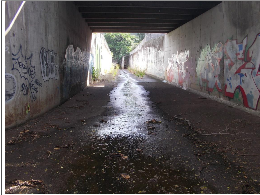
Photograph # 1: Upstream Site looking upstream.
