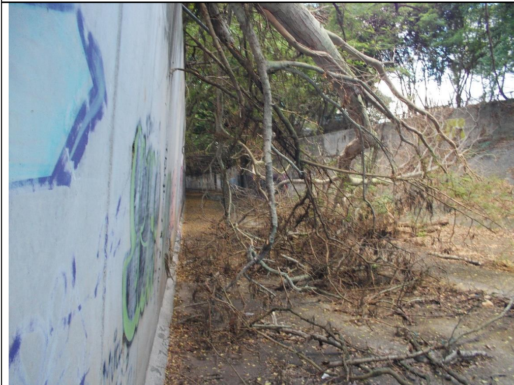
Photograph # 2: Upstream Site looking downstream.
