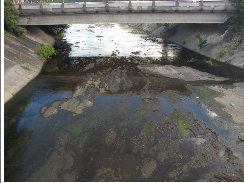
Photograph # 1: Downstream Site 1 looking upstream.
