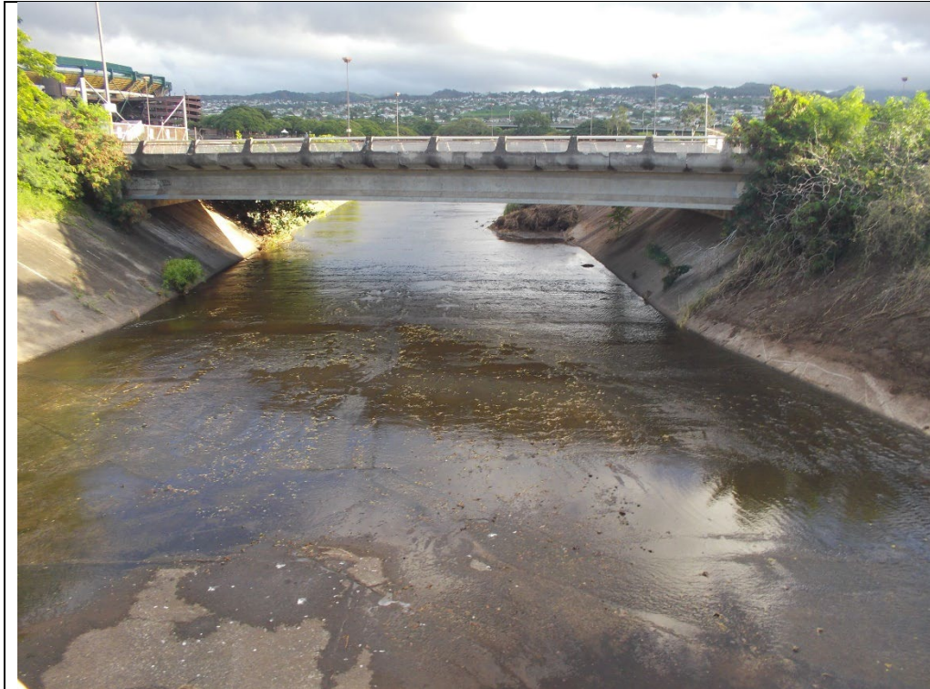
Photograph # 1: Downstream Site 1 looking upstream.
