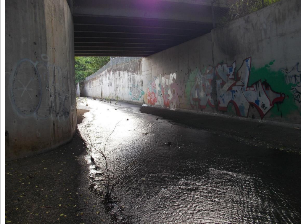
Photograph # 1: Upstream Site looking upstream.
