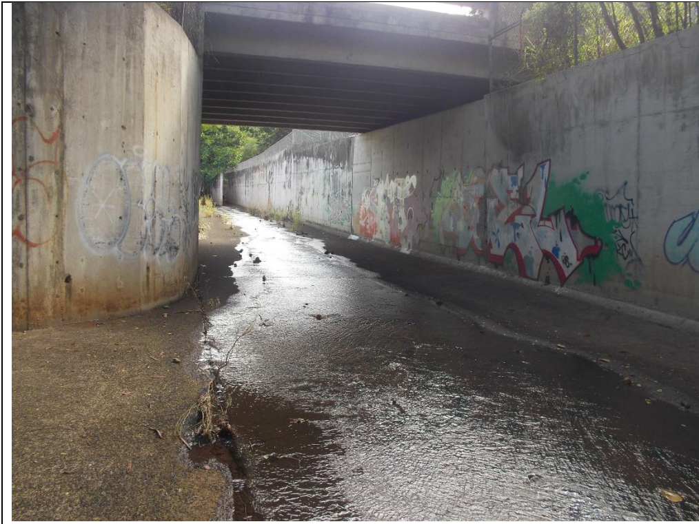
Photograph # 1: Upstream Site looking upstream.
