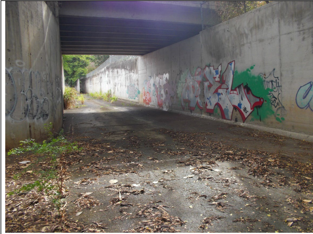
Photograph # 1: Upstream Site looking upstream.
