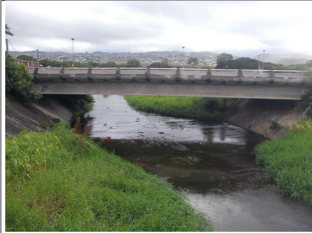
Photograph # 1: Downstream Site 1 looking upstream.
