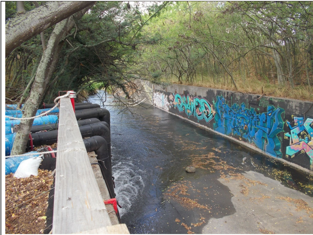
Photograph # 2: Discharge Site looking downstream.
