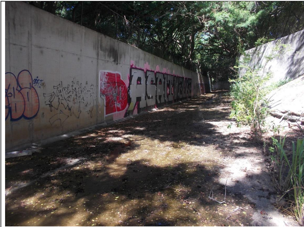
Photograph # 1: Upstream Site looking upstream.
