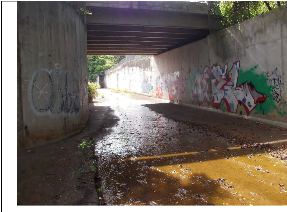
Photograph # 1: Upstream Site looking upstream.
