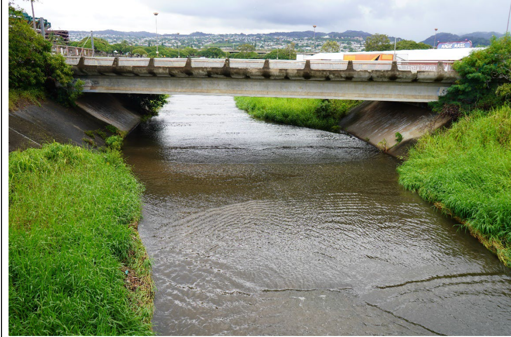
Photograph # 1: Downstream Site # 1.
