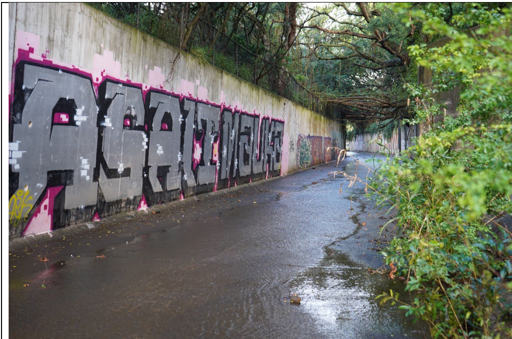
Photograph # 2: Upstream Site looking downstream.
