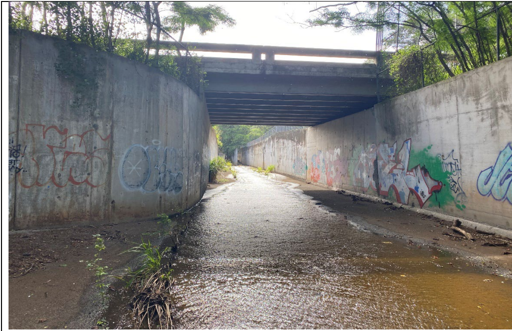
Photograph # 1: Upstream Site looking upstream.
