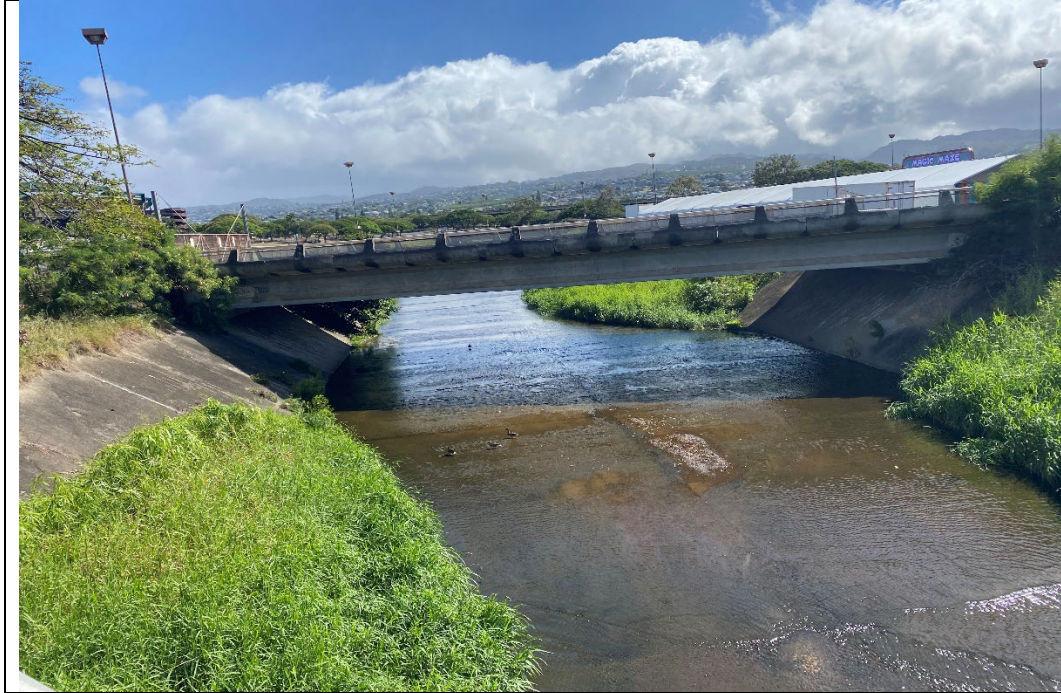
Photograph # 1: Downstream Site #1 looking upstream.
