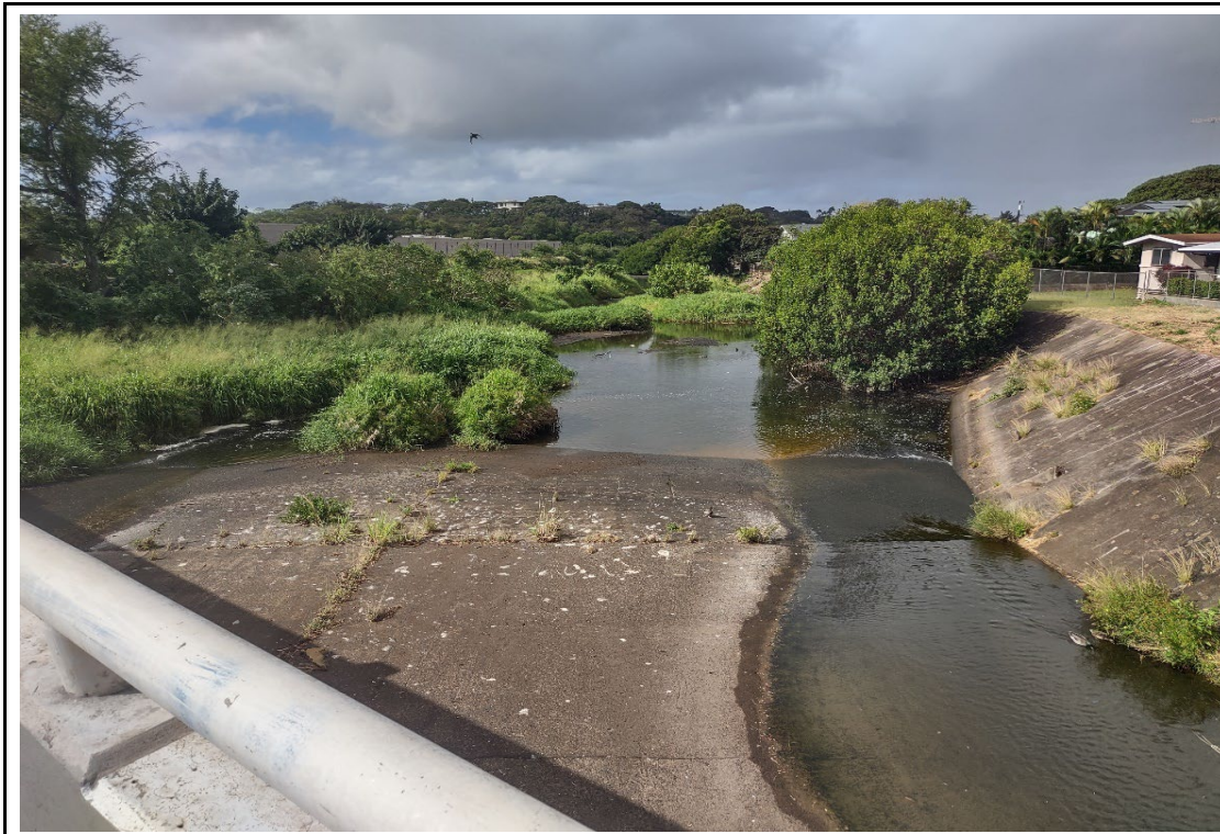
Photograph: Downstream Site #2 looking downstream.
