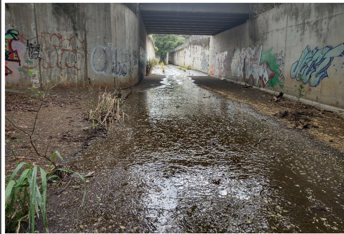
Photograph #1: Upstream Site looking upstream.
