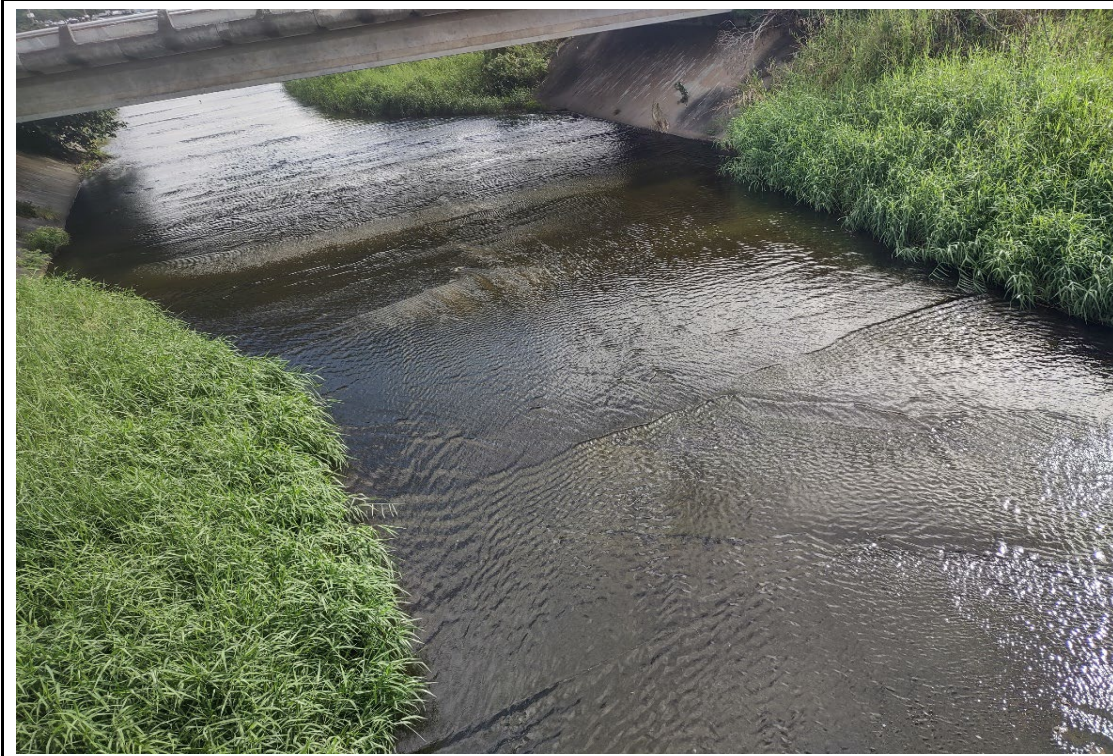
Photograph: Downstream Site #1 looking upstream.
