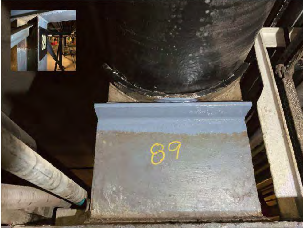
Re-seated and shimmed line at PS-89.
