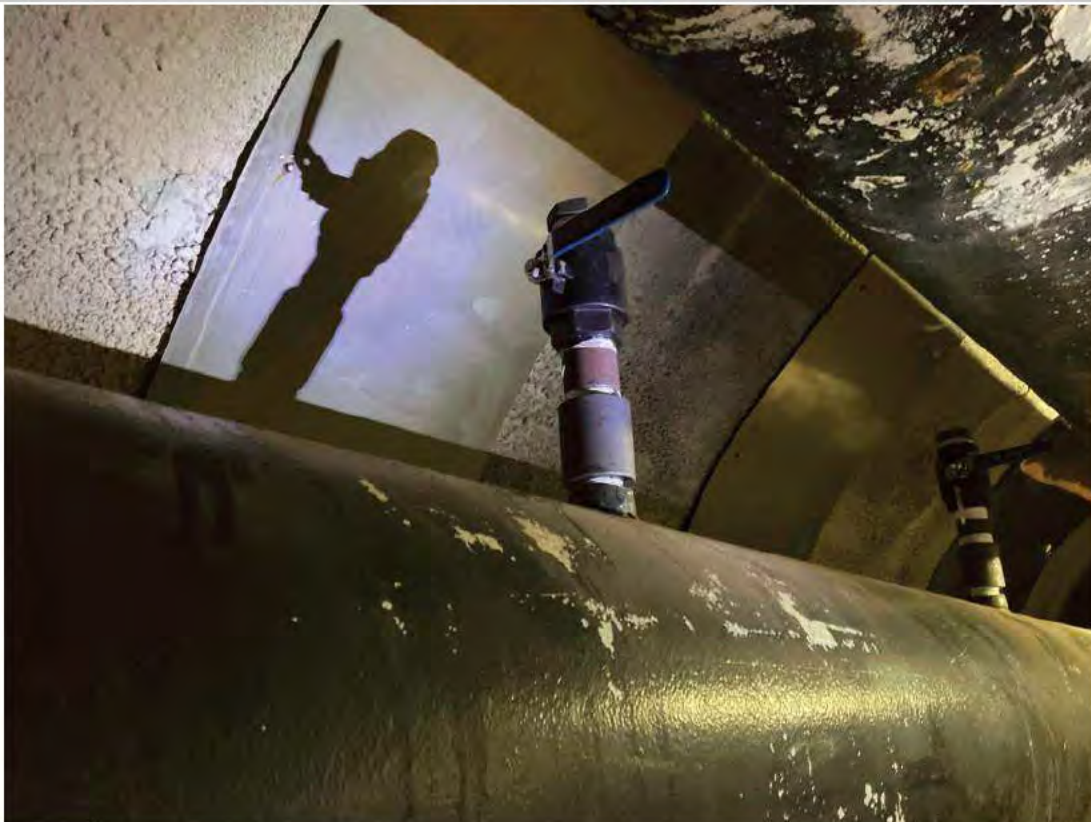
Threaded assembly replaced at PS 595 (1 of 2).
