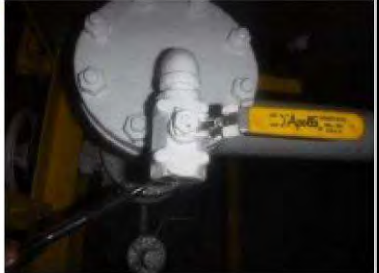
Existing condition (b) (3) (A) ball valve on FOR line without plug at Surge Tank 4.
