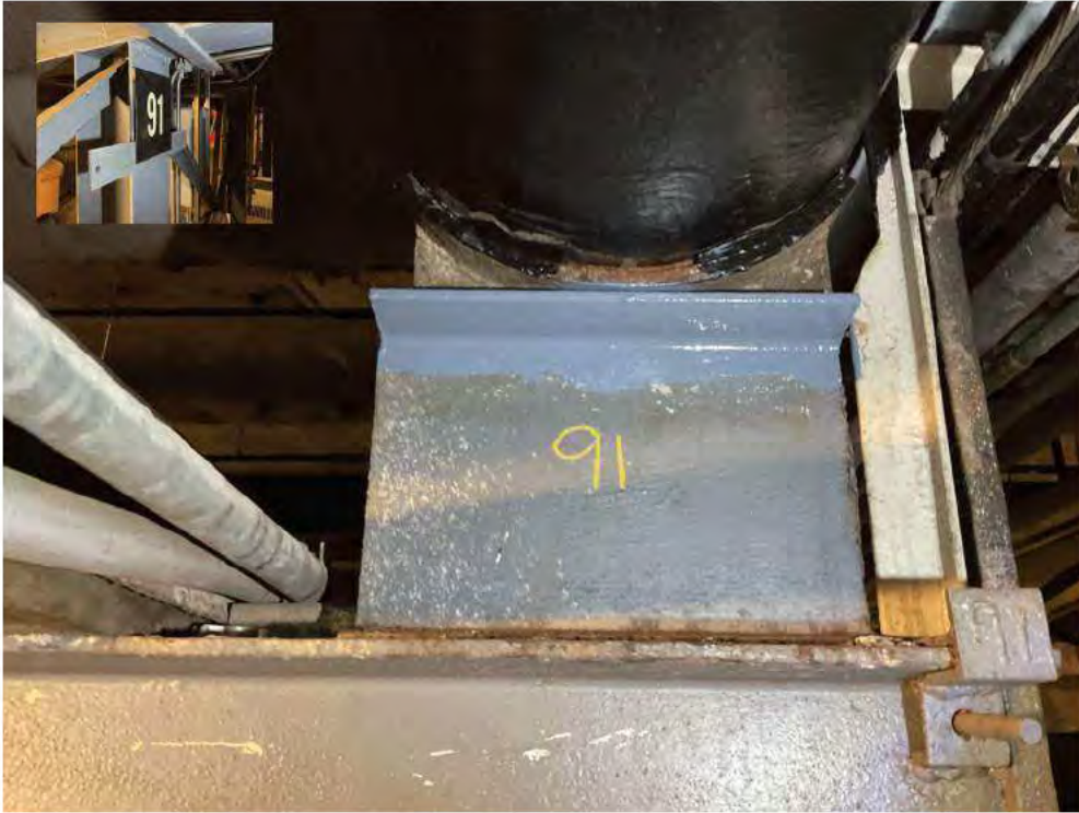
Re-seated and shimmed line at PS-91.
