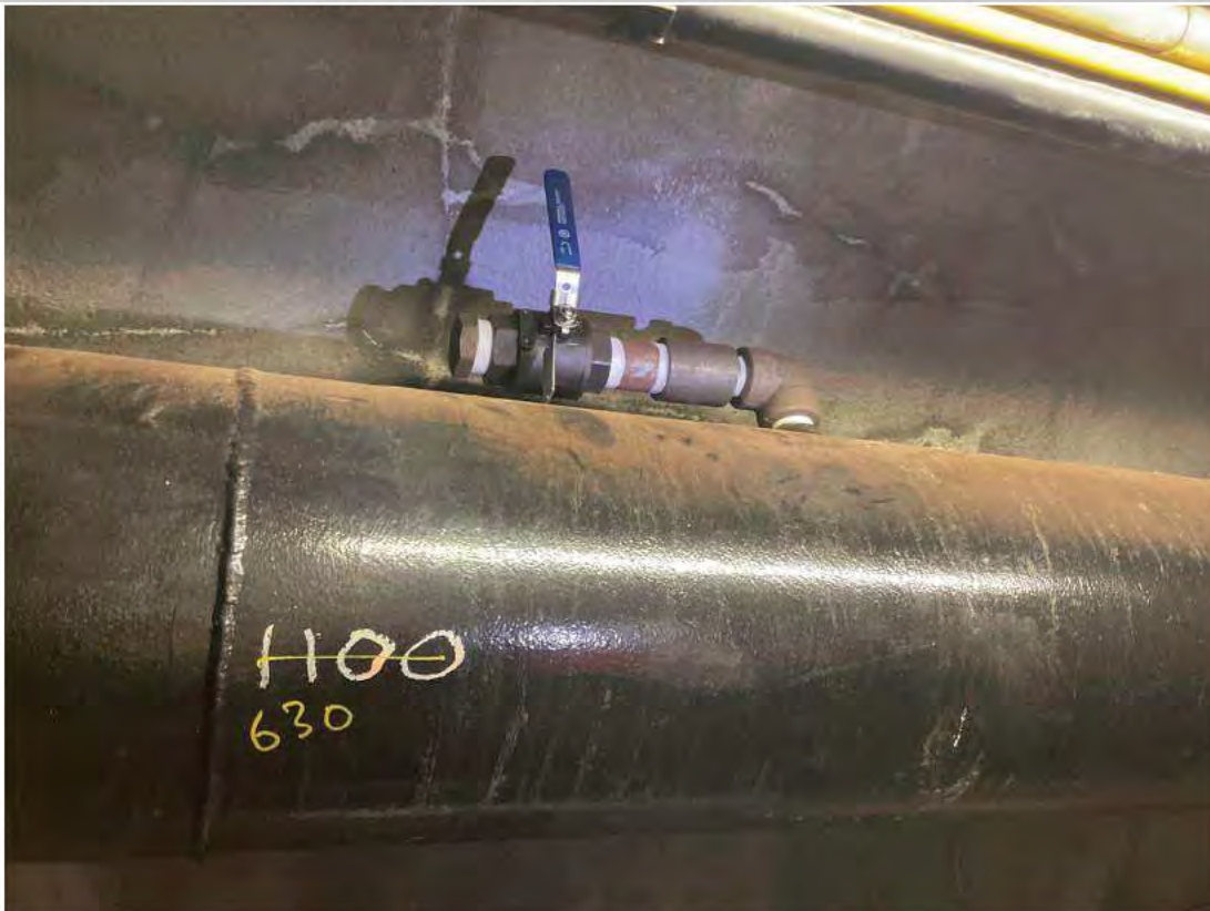
High point vent assembly replaced at PS 584.
