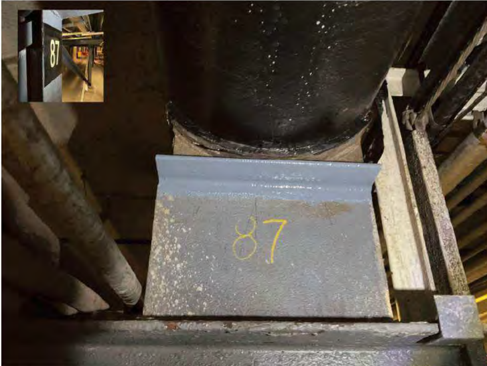
Re-seated and shimmed line at PS-87.
