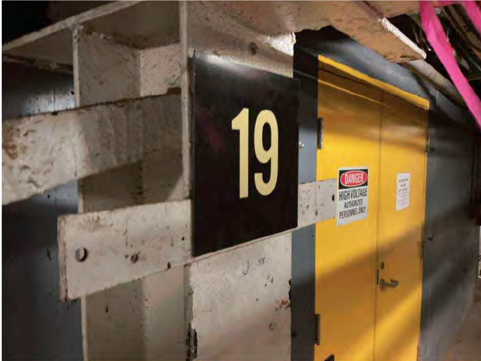
Existing Pipe Support 19.
