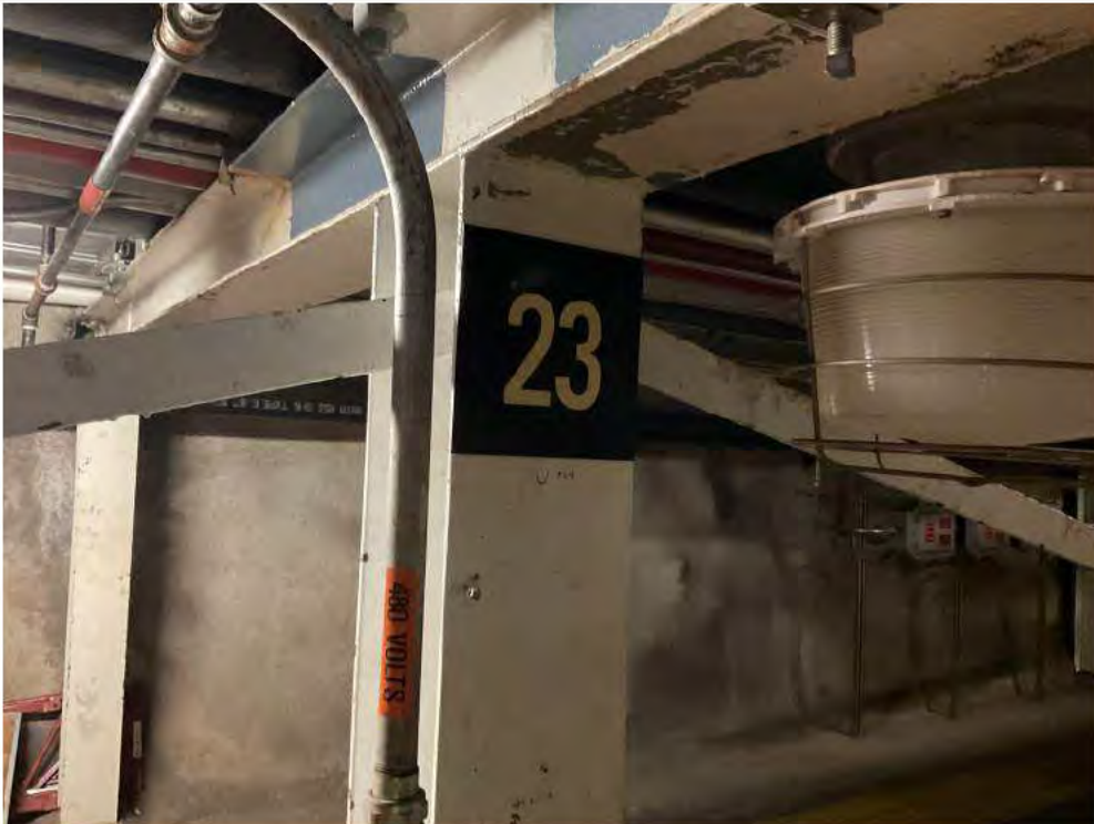
Existing Pipe Support 23.
