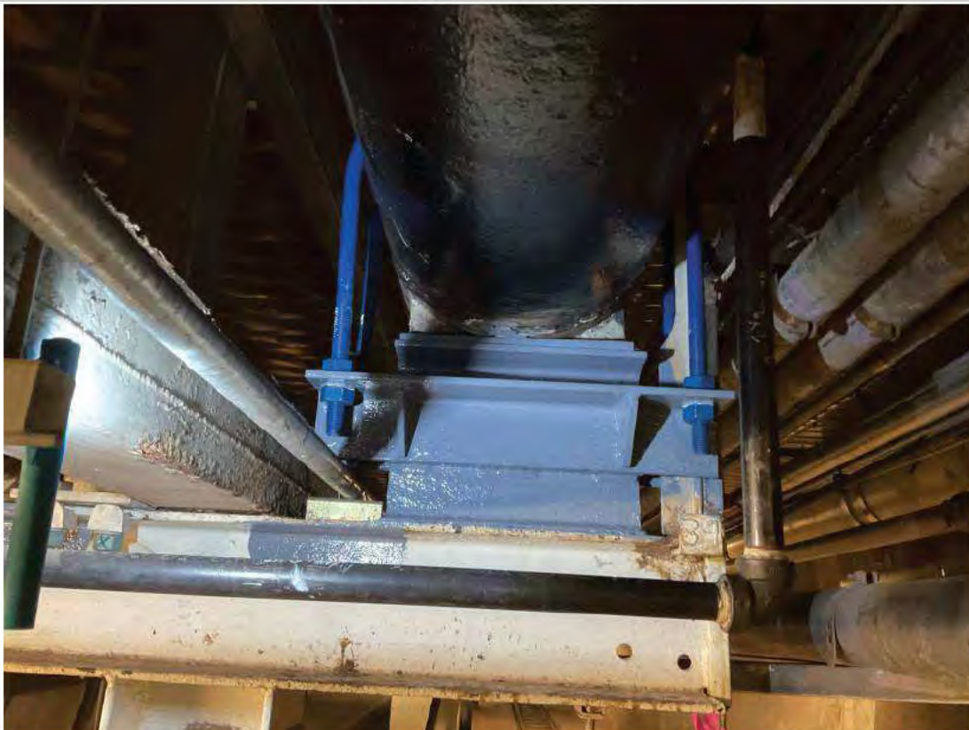
New welded bracket and U-bolt restraints existing Pipe Support 34.
