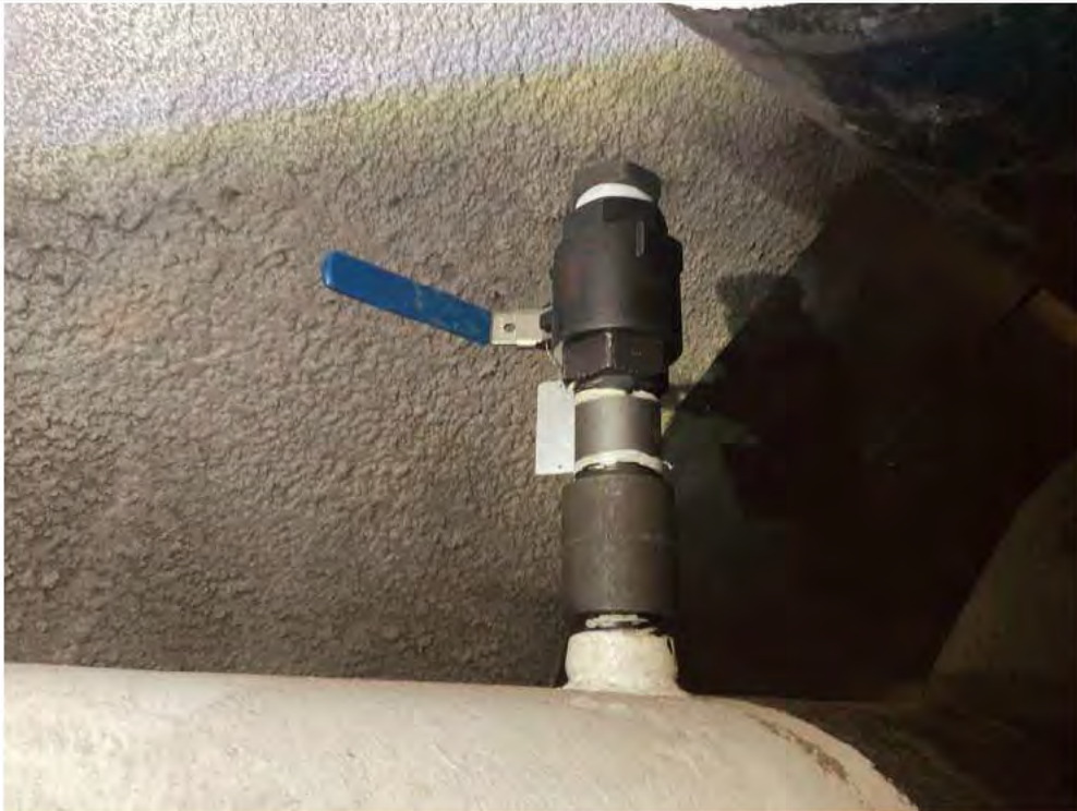
Threaded assembly replaced at PS 277.
