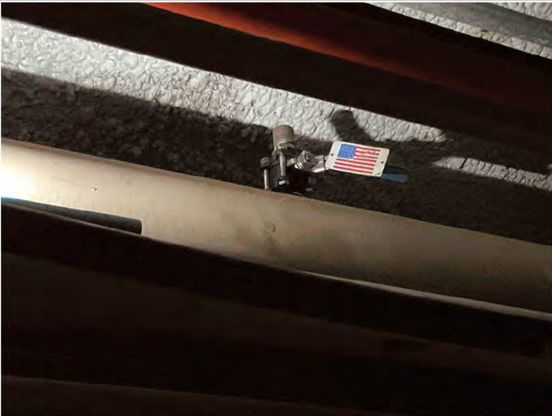
Replaced 3/4-inch threaded assembly at PS 205
