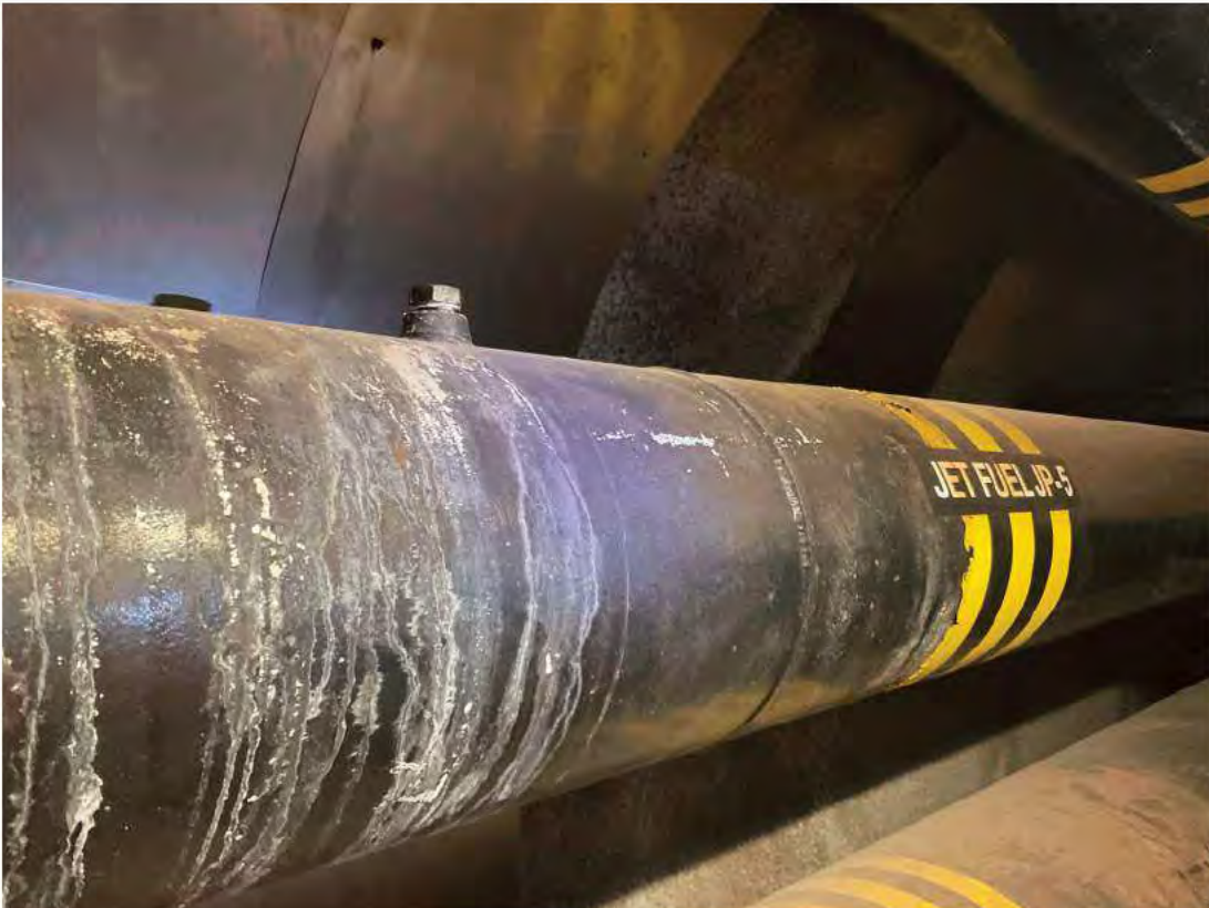
Threaded plug replaced at PS 597.
