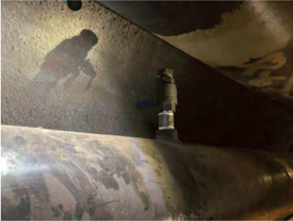
Threaded assembly replaced at PS 205.
