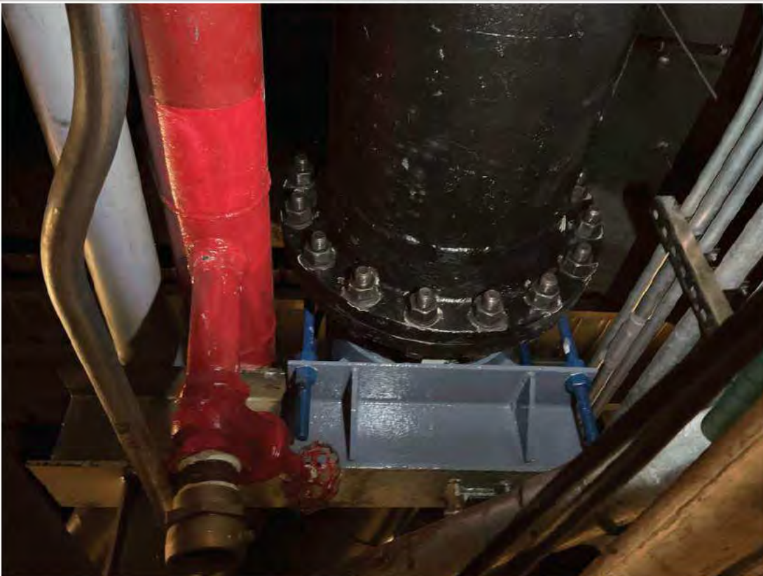
New welded bracket and U-bolt restraints existing Pipe Support 20.
