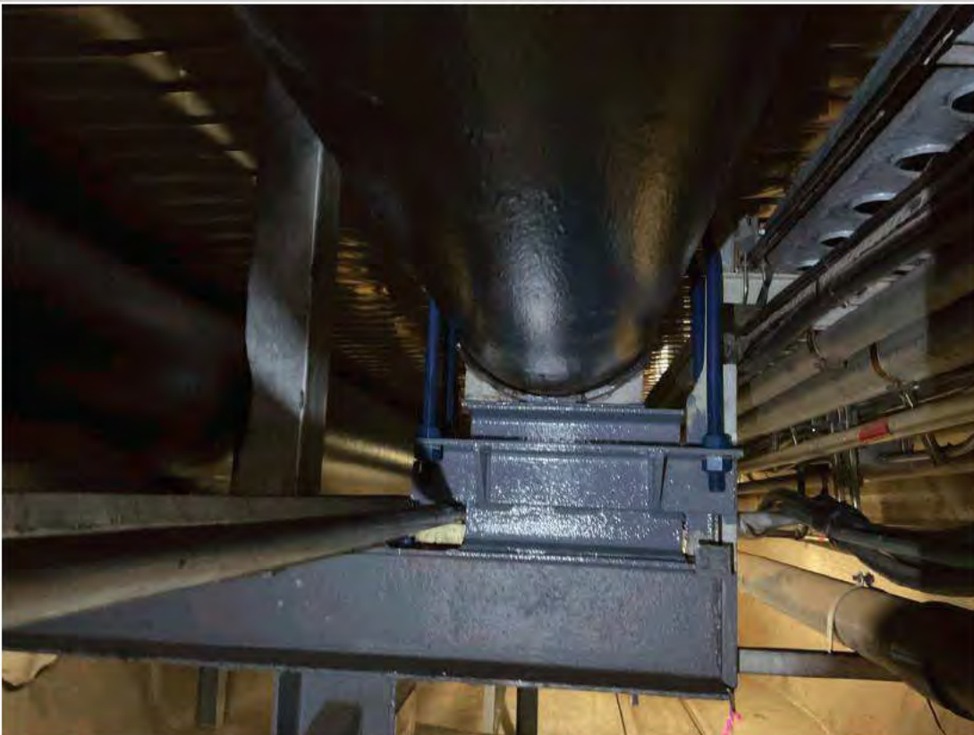
New welded bracket and U-bolt restraints at Pipe Support 53.
