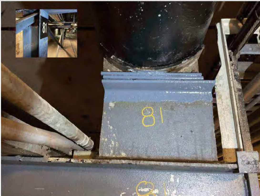
Re-seated and shimmed line at PS-81.
