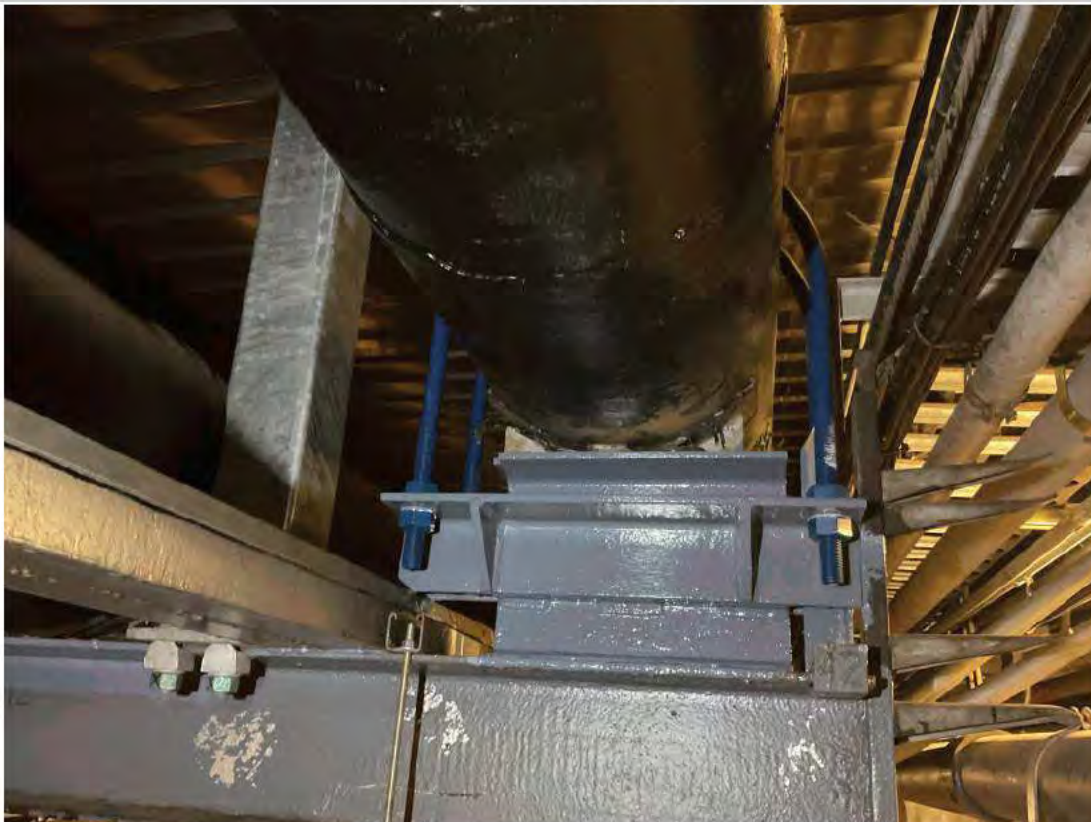
New welded bracket and U-bolt restraints existing Pipe Support 42.
