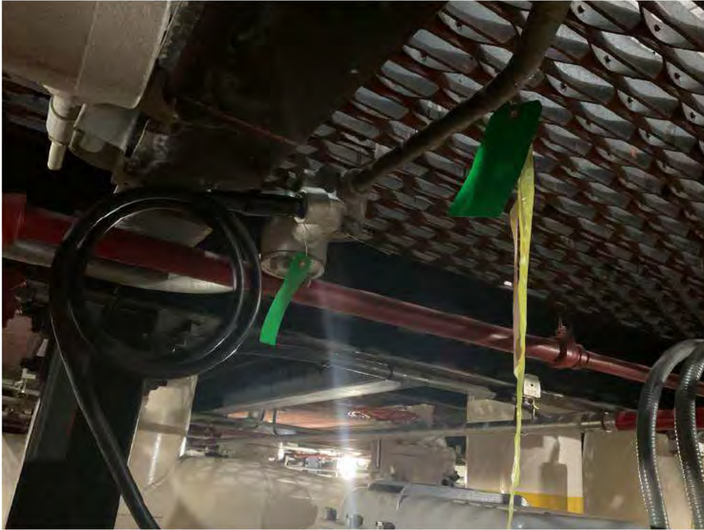
Condulet GUA Cover installation (typical) with QA tags.
