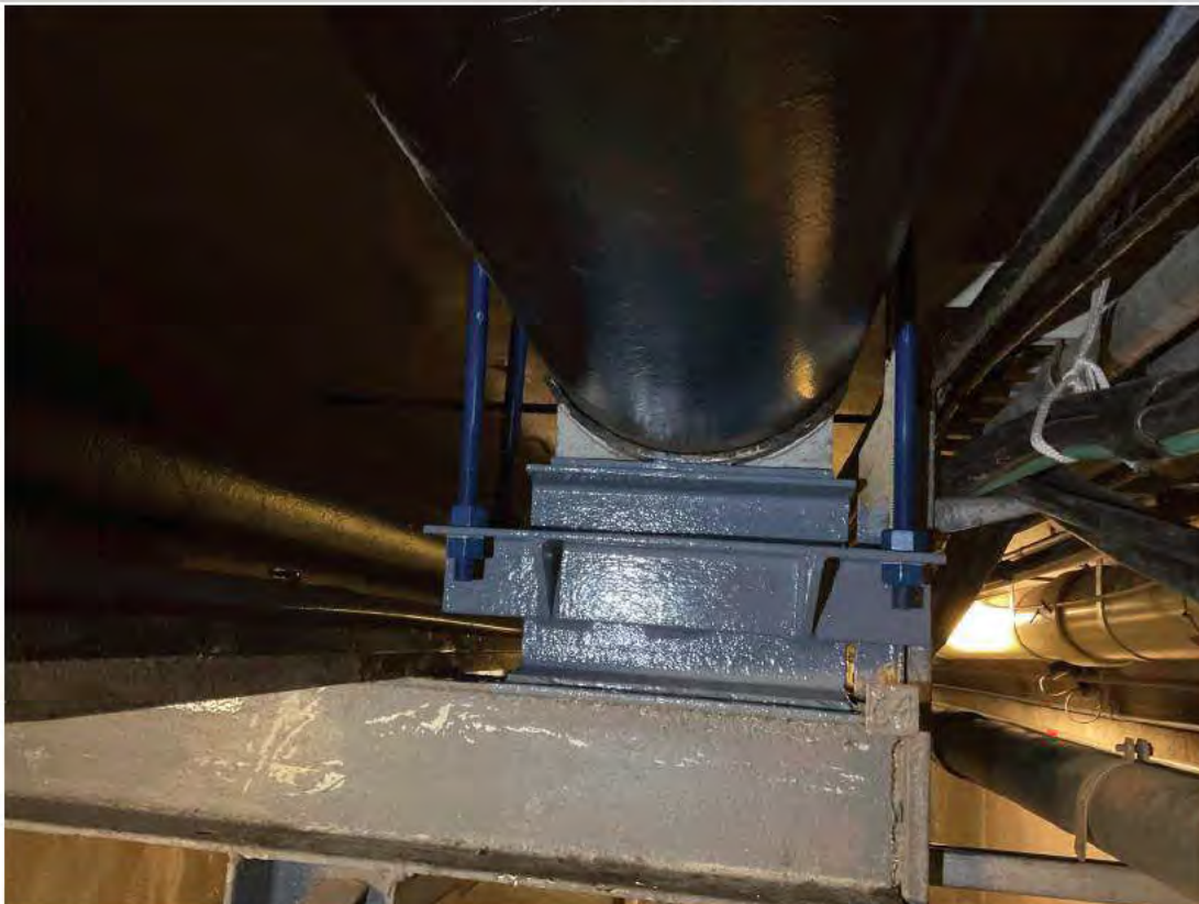
New welded bracket and U-bolt restraints at Pipe Support 64.
