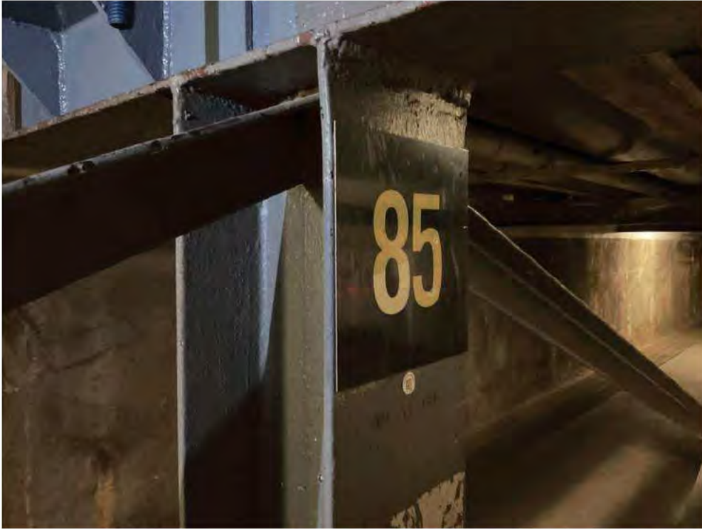
Existing Pipe Support 85.
