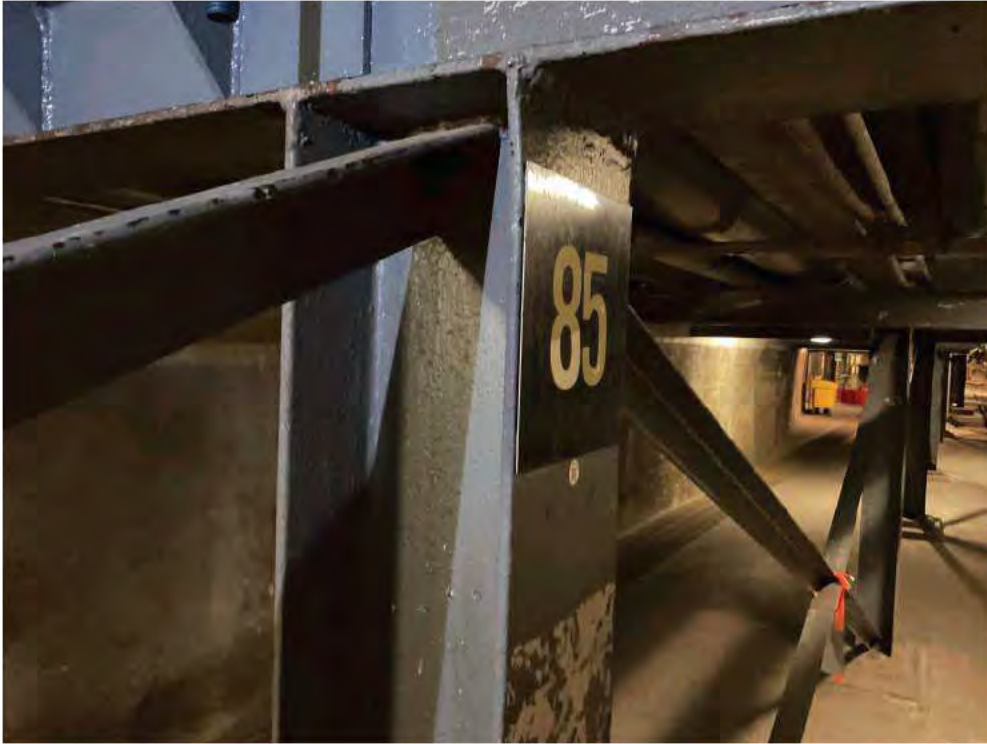
Existing Pipe Support 85.
