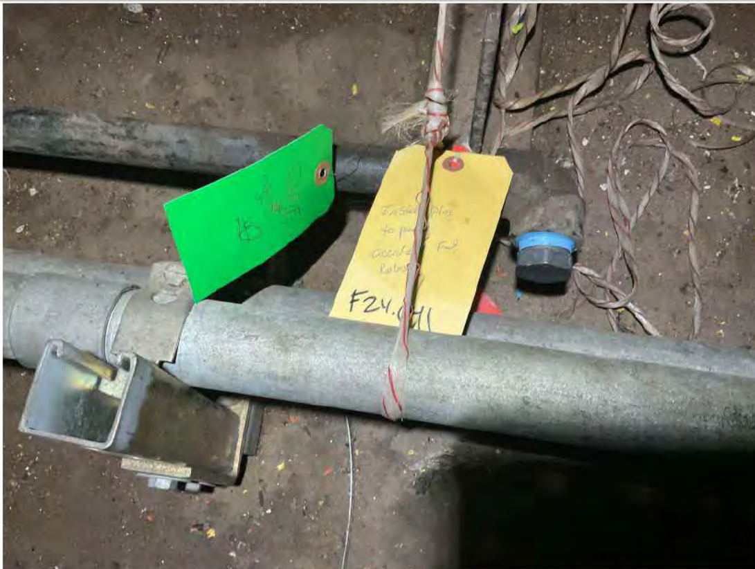
Threaded pipe (b) (3) (A) with fuel-resistant thread sealant.
