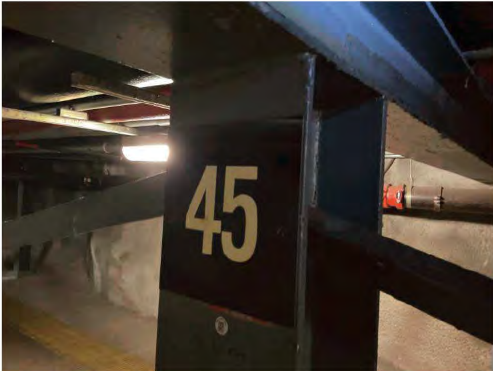
Existing Pipe Support 45.
