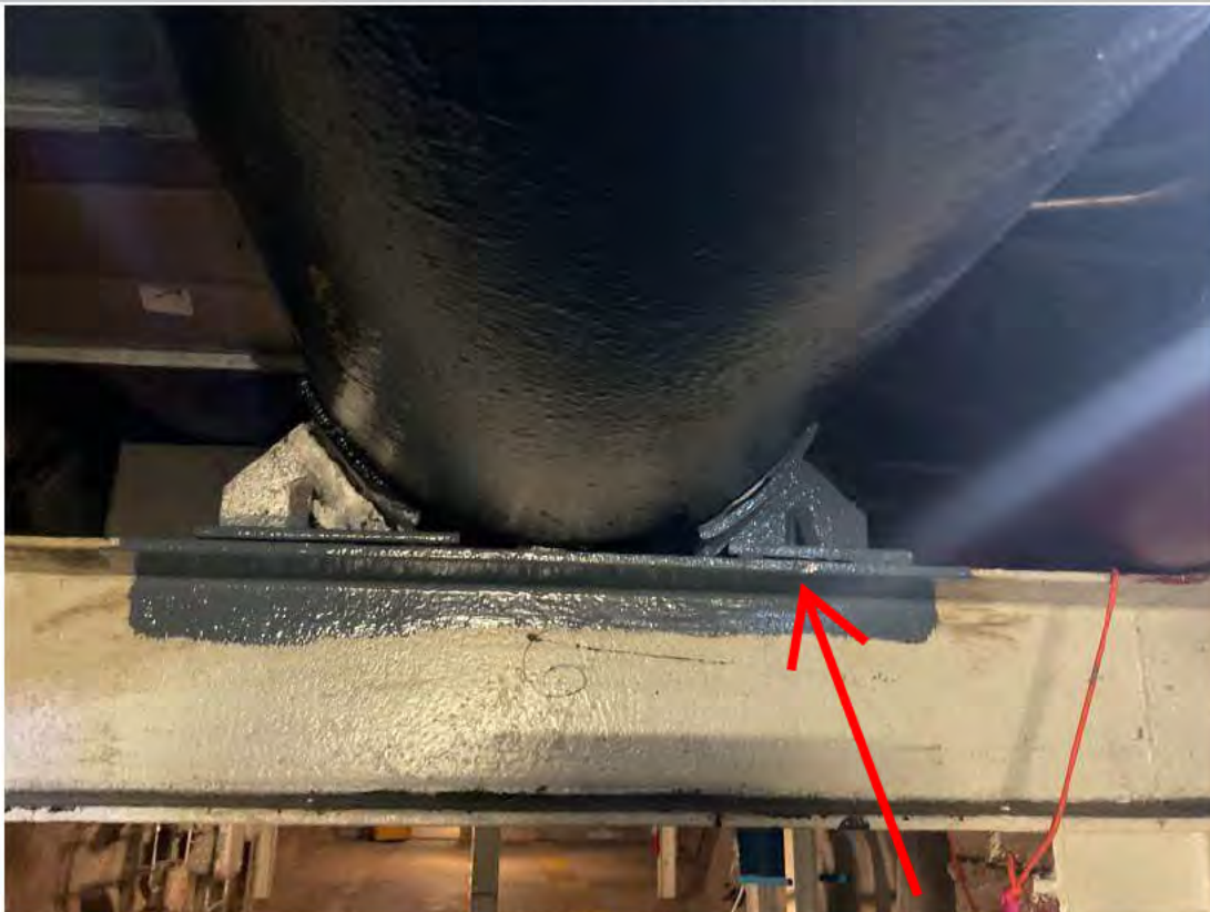
Replaced missing cradle (right) at Pipe Support 6.
