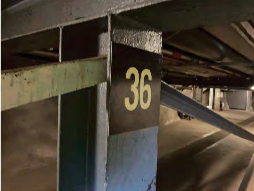
Existing Pipe Support 36.
