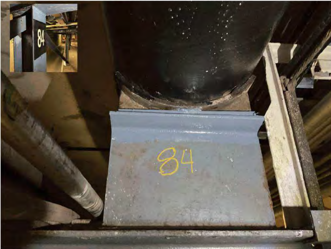
Re-seated and shimmed line at PS-84.
