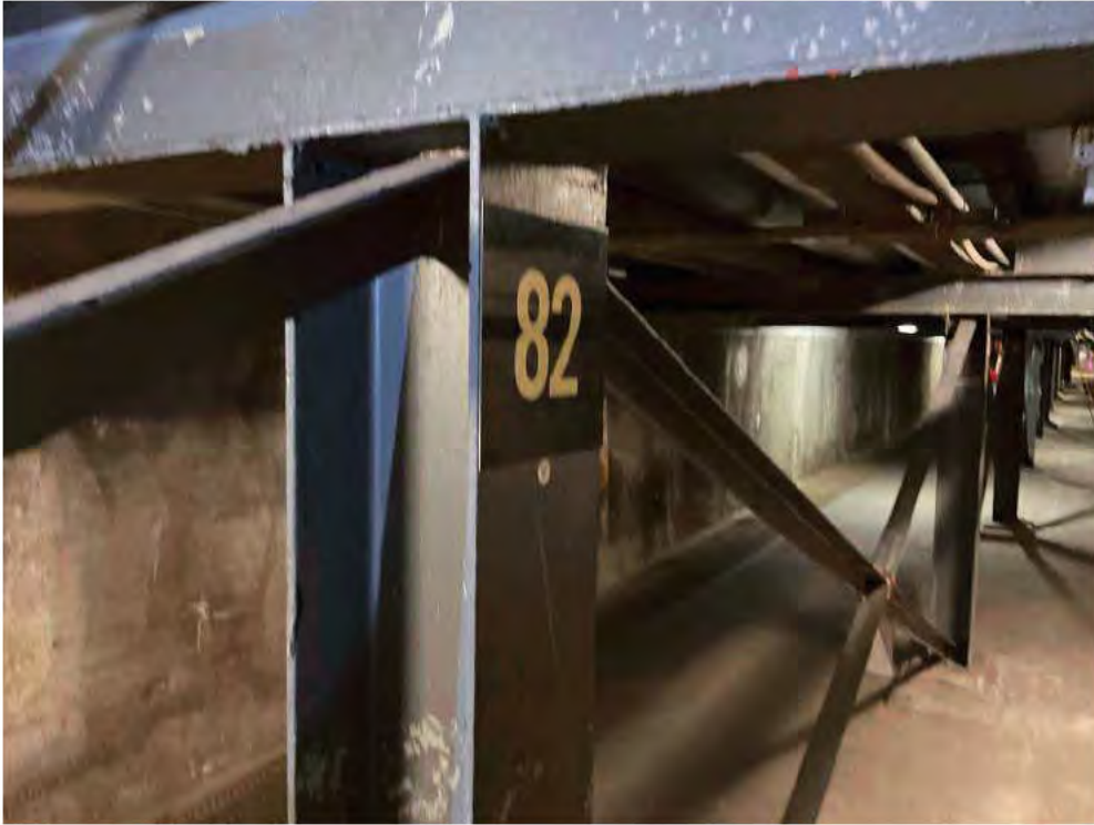
Existing Pipe Support 82.
