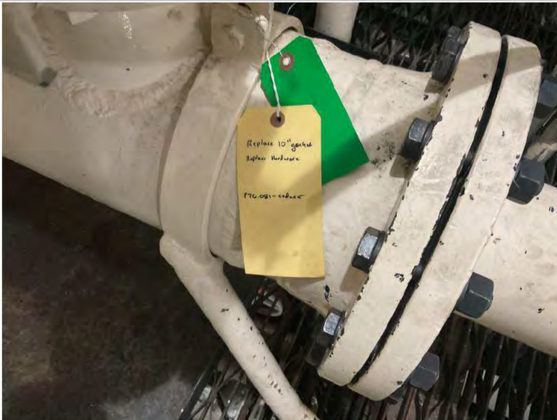
Replaced gasket and hardware on F-76 pressure relief assembly.
