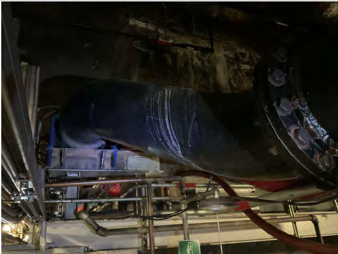
New offset spool installed at Pipe Support 4.
