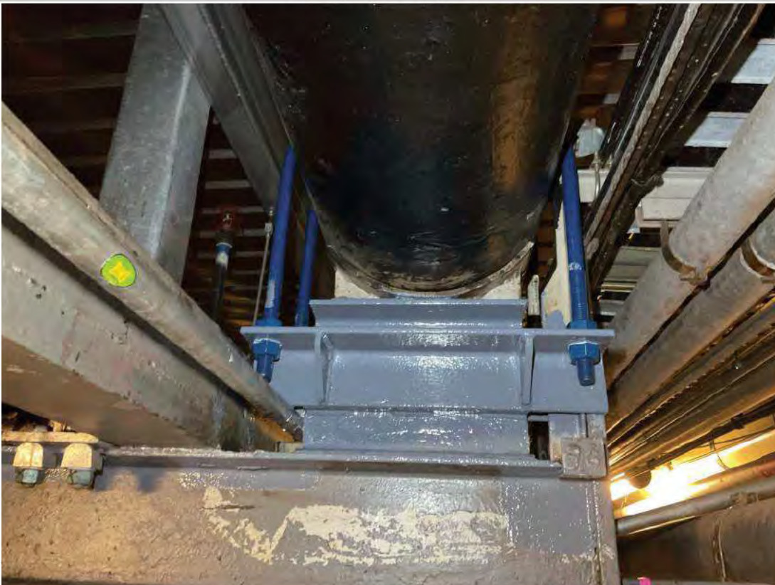
New welded bracket and U-bolt restraints existing Pipe Support 36.
