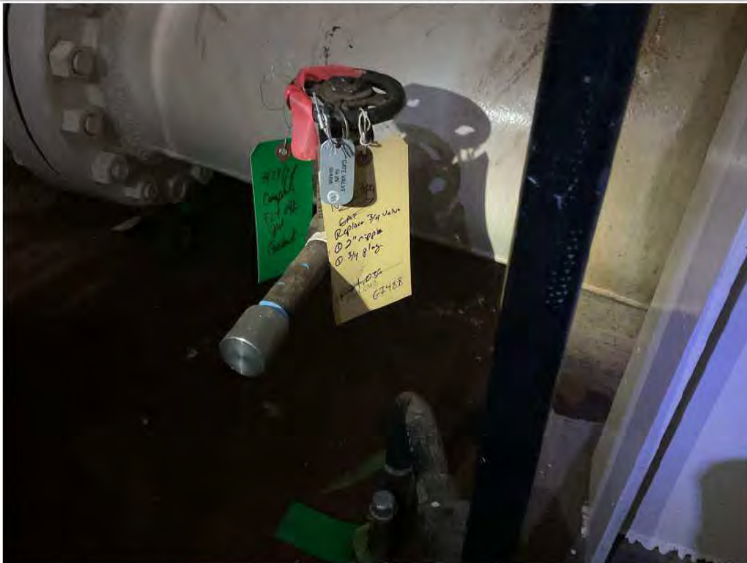
Installed threaded cap on pipeline nipple to prevent accidental discharge.
