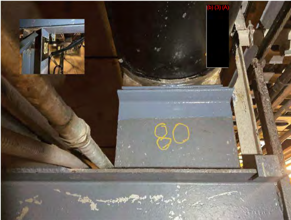
Re-seated and shimmed line at PS-80.
