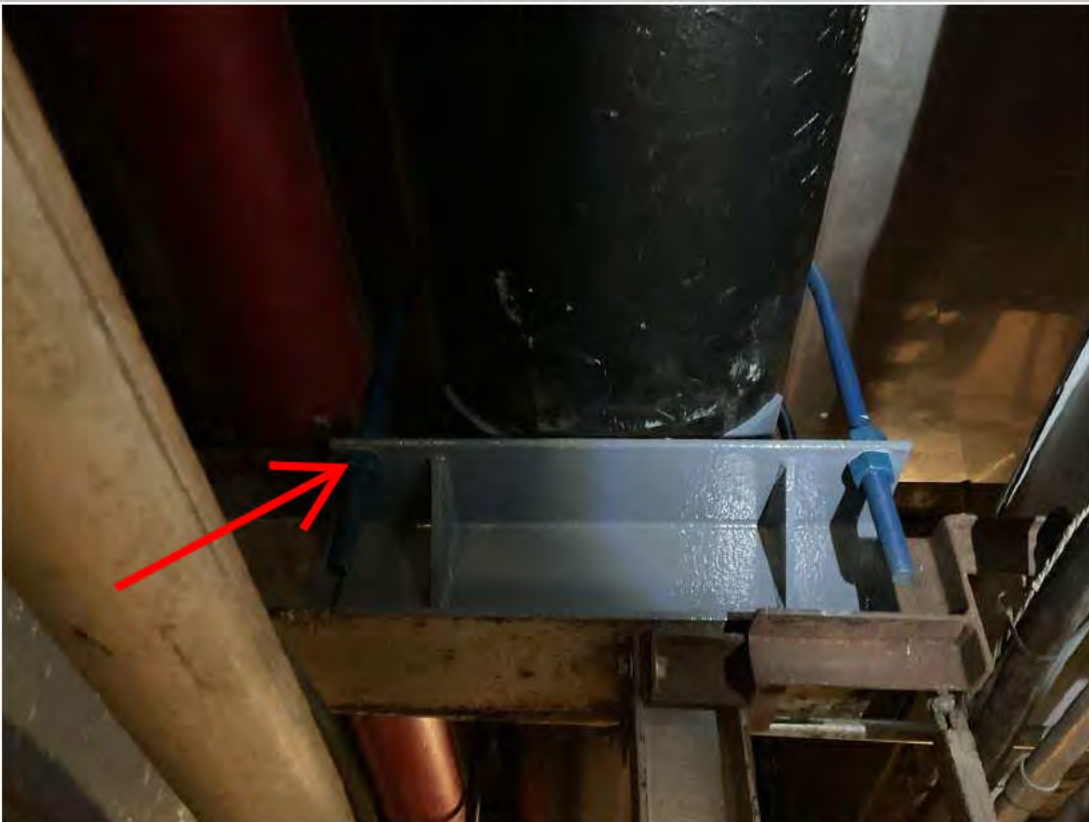
New welded bracket and U-bolt restraints existing Pipe Support 18.
