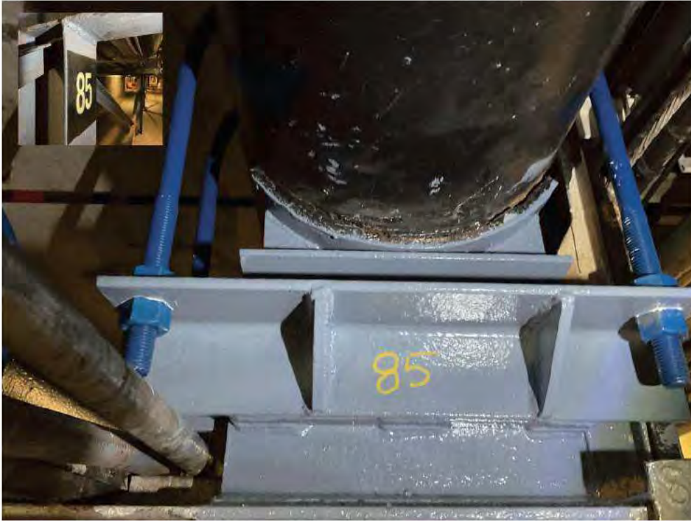
Re-seated and shimmed line at PS-85.
