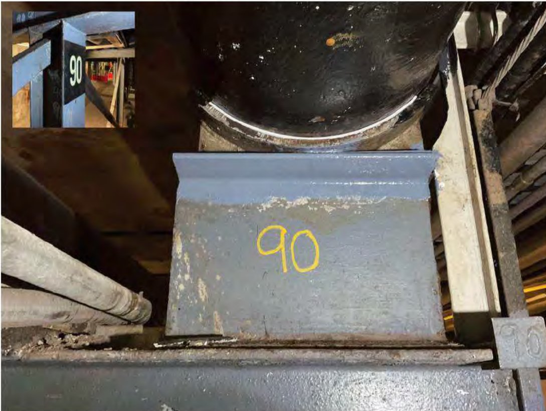
Re-seated and shimmed line at PS-90.
