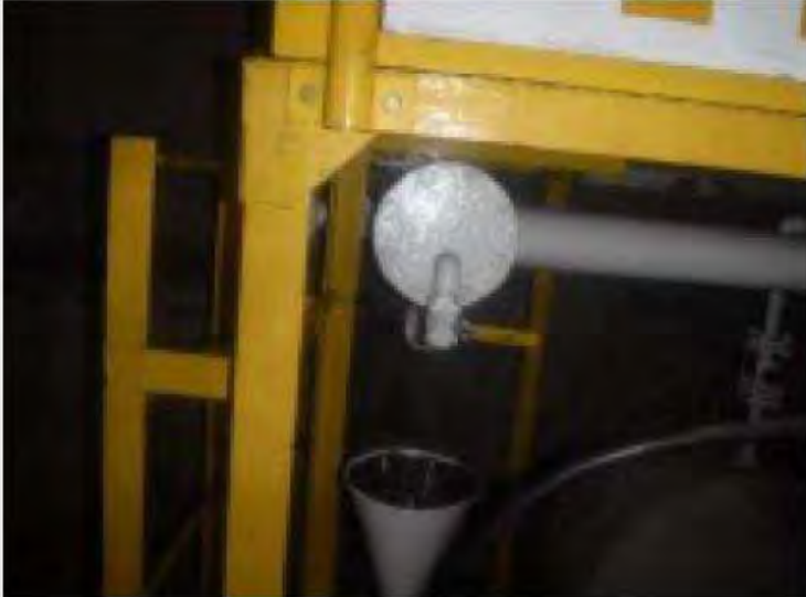
Existing condition (b) (3) (A) ball valve on FOR line without plug at Surge Tank 4.
