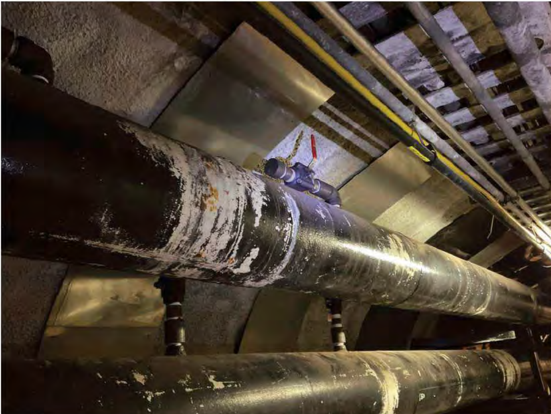
Replaced threaded component assembly at PS 595 (2 of 2).
