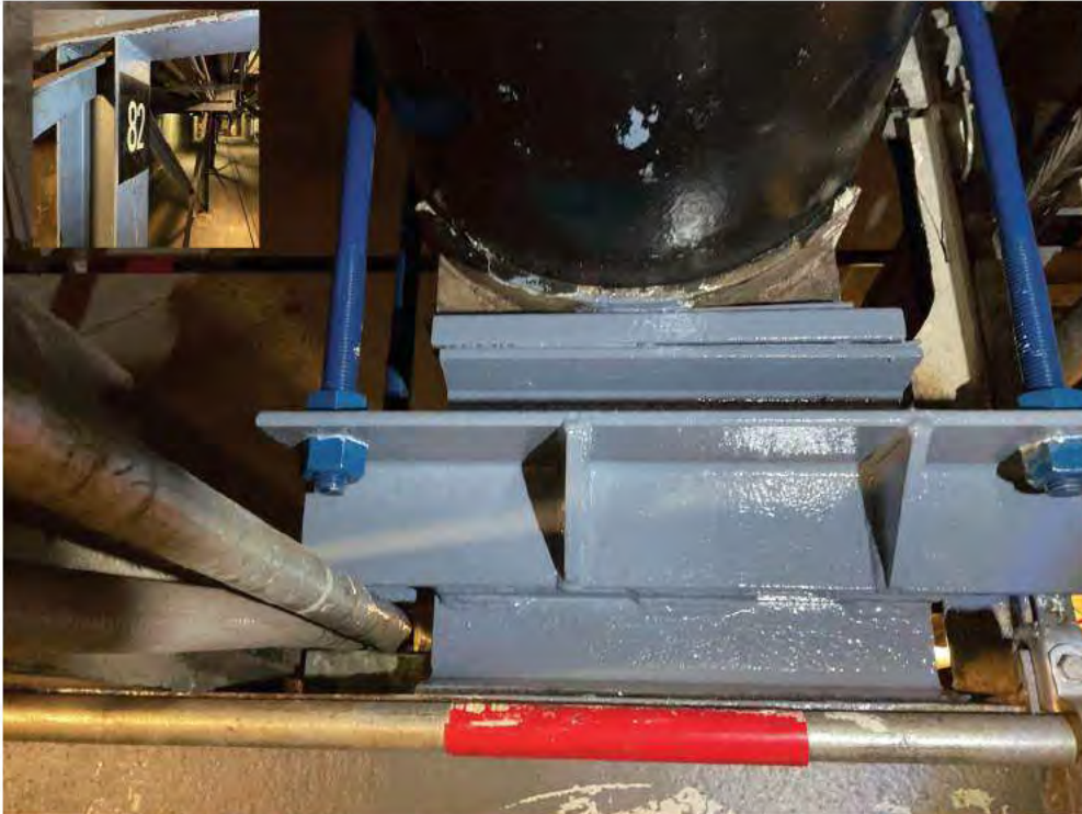
Re-seated and shimmed line at PS-82.
