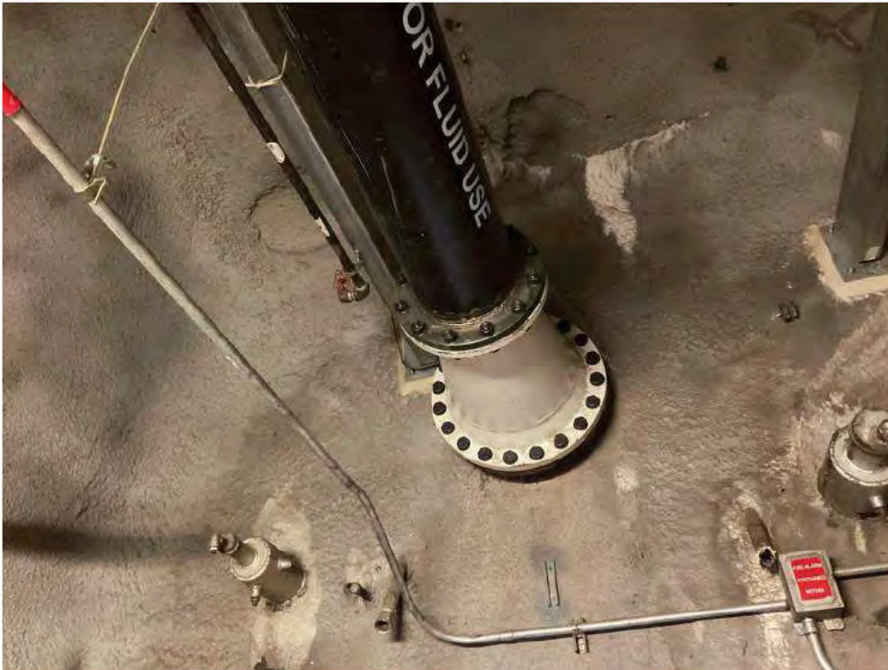
Deadleg installed between Tank 18 and main header for lateral restraint.
