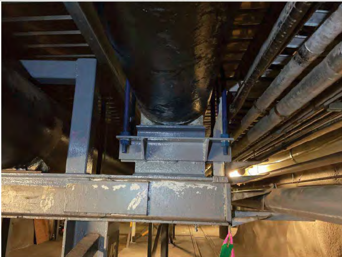
New welded bracket and U-bolt restraints at Pipe Support 45.
