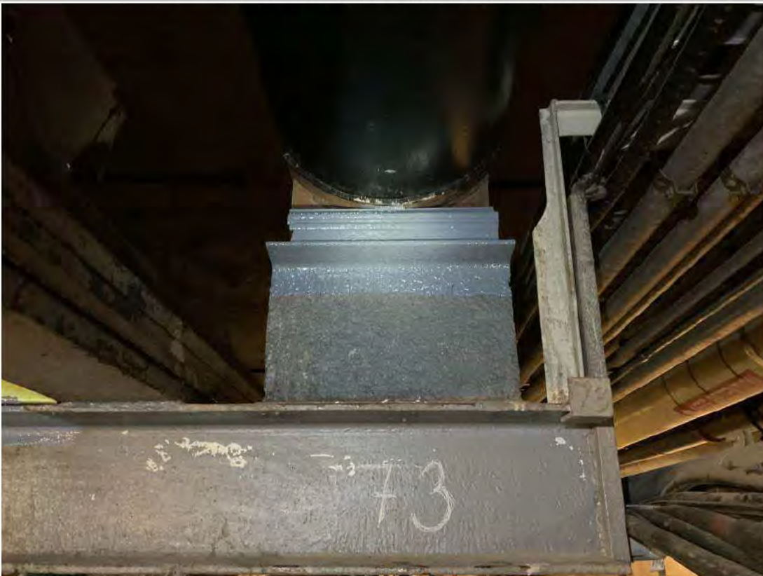
Reseated line with shims and re-oriented pipe cradle at Pipe Support 73.
