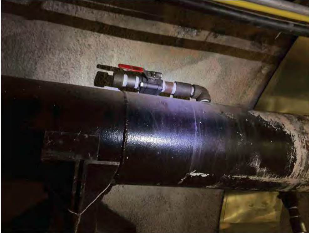
Replaced threaded component assembly at PS 595 (1 of 2).
