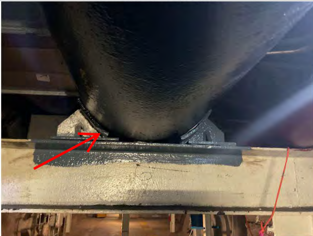
Replaced missing cradle (right) at Pipe Support 6.
