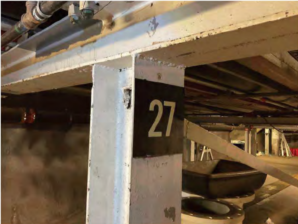
Existing Pipe Support 27.
