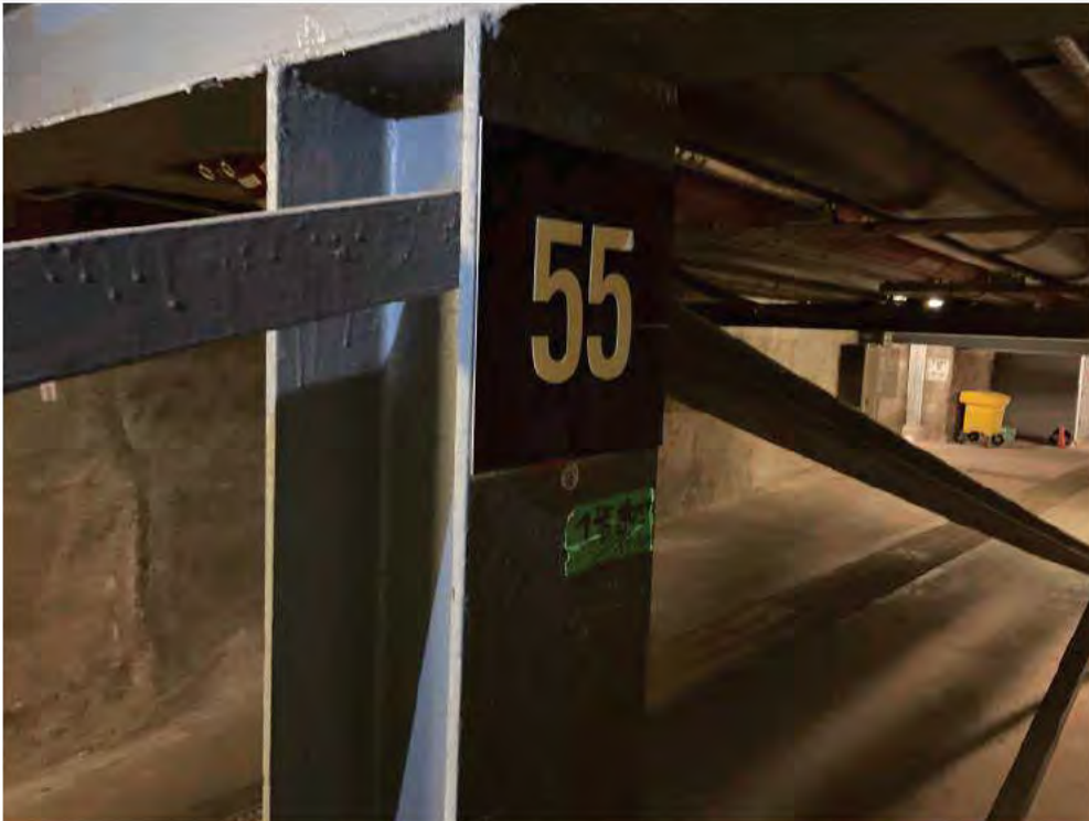
Existing Pipe Support 55.
