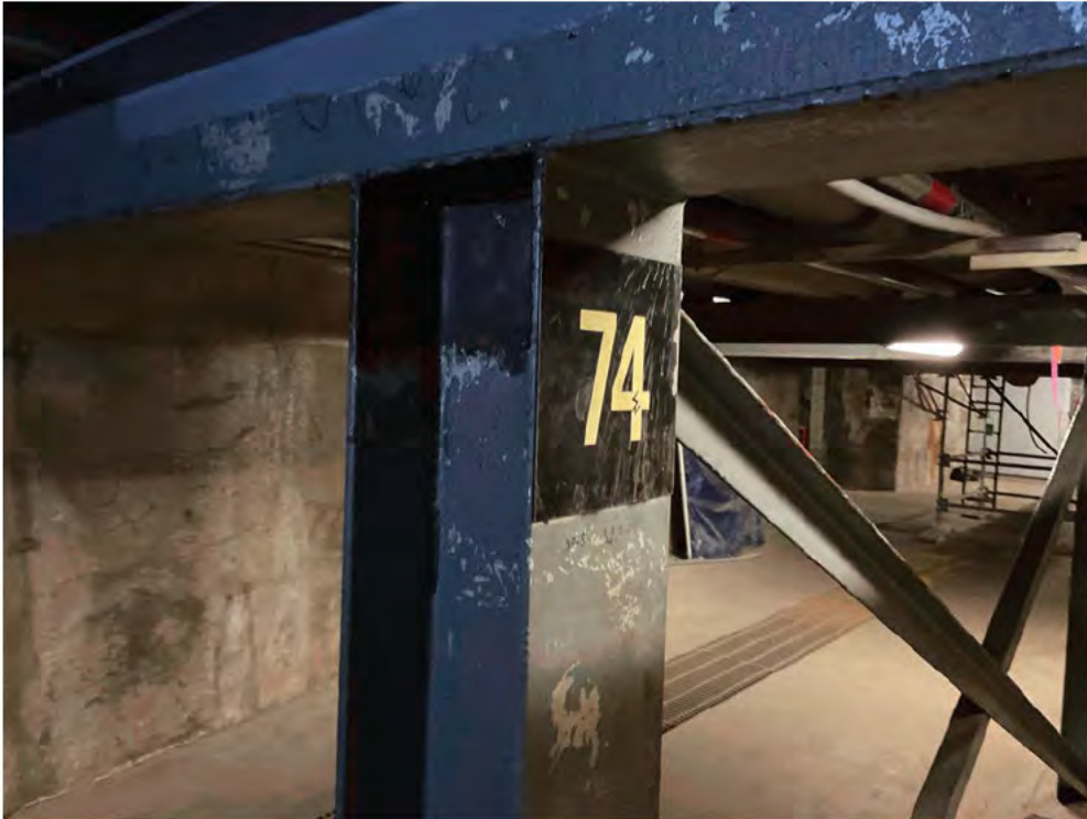
Existing Pipe Support 74.
