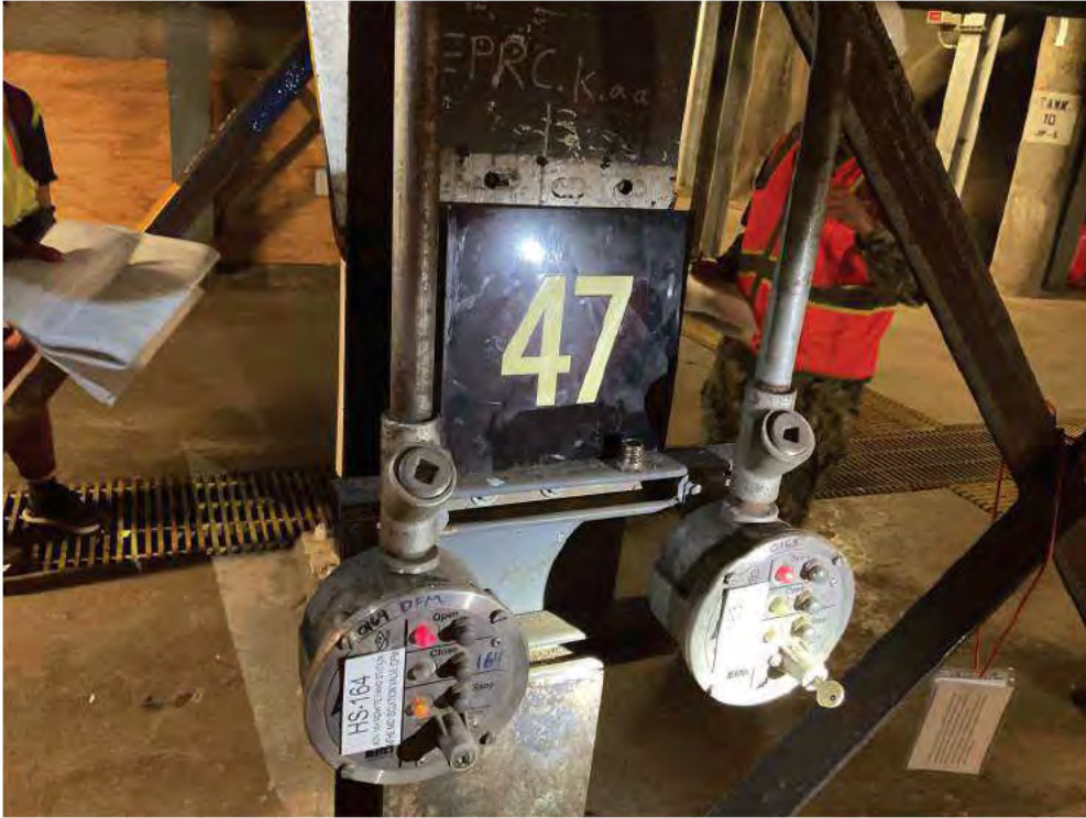
Existing Pipe Support 47.
