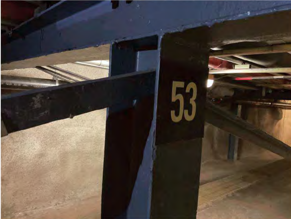
Existing Pipe Support 53.
