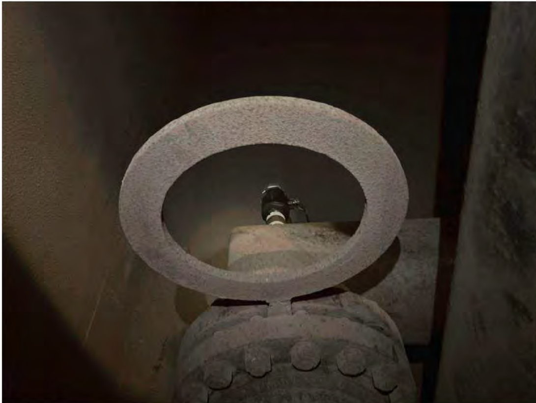
Threaded assembly replaced at PS 206.
