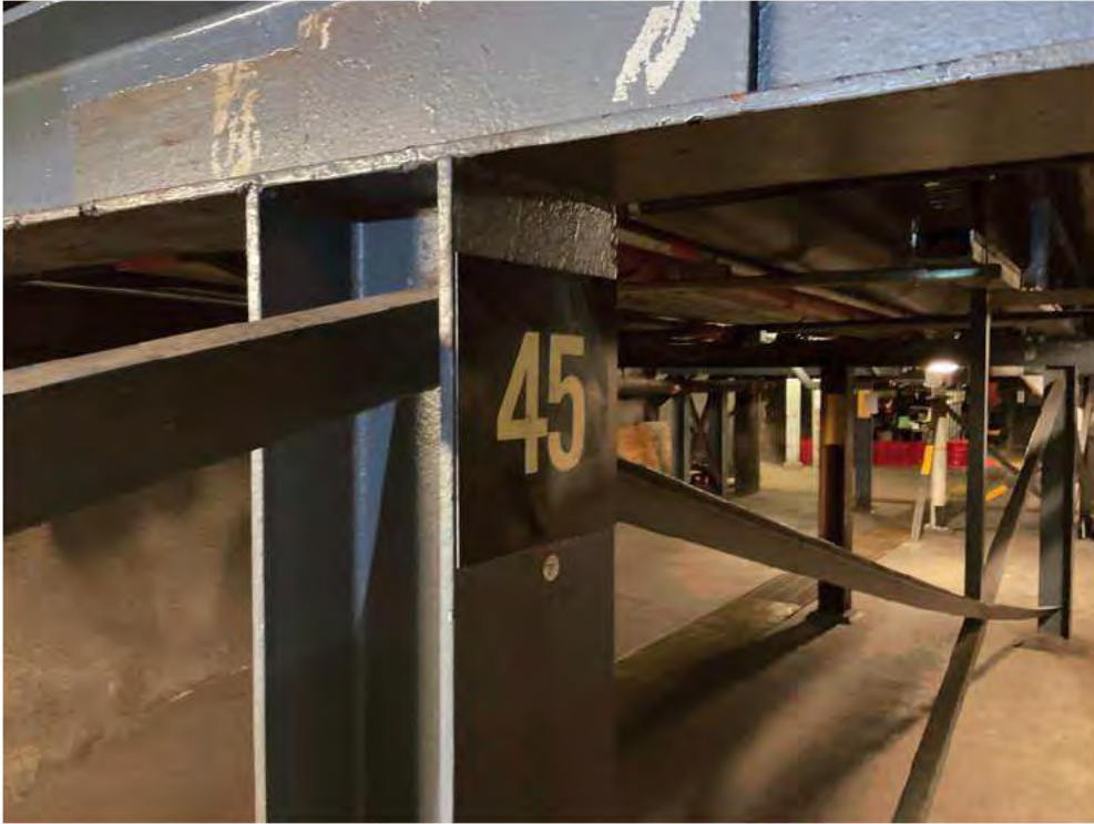
Existing Pipe Support 45.
