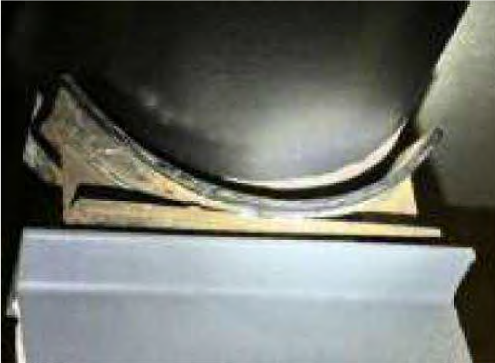
Existing condition at Pipe Support 73 prior to repair.
