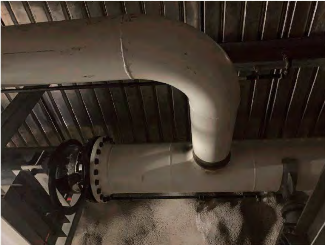
Deadleg installed between Tank 14 and main header for lateral restraint.
