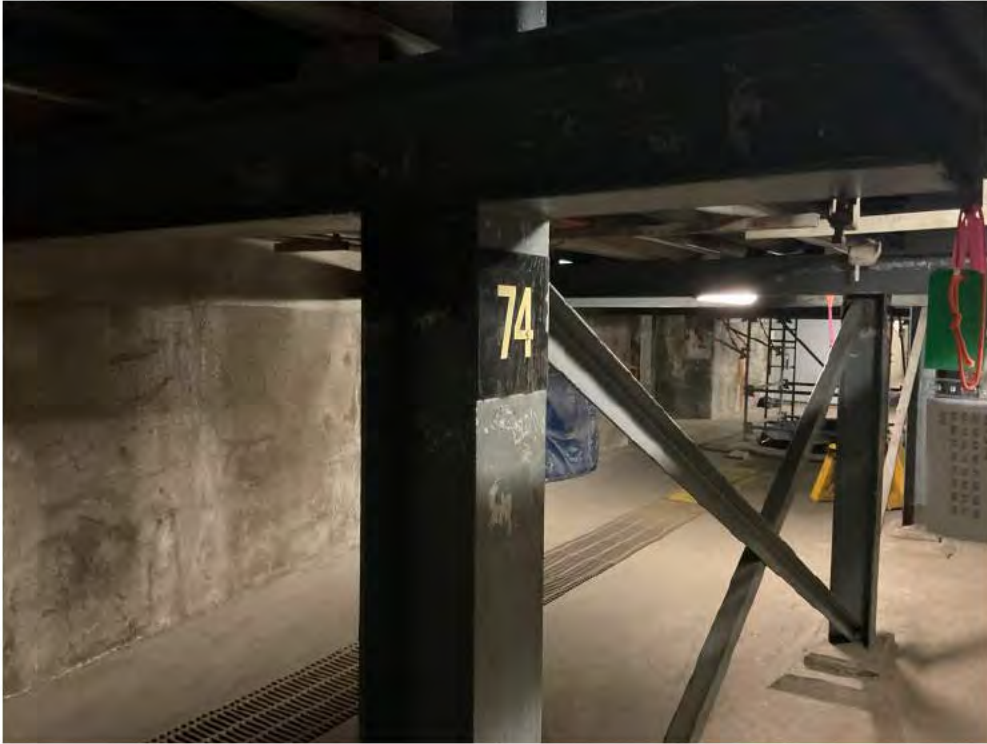
Existing Pipe Support 74.
