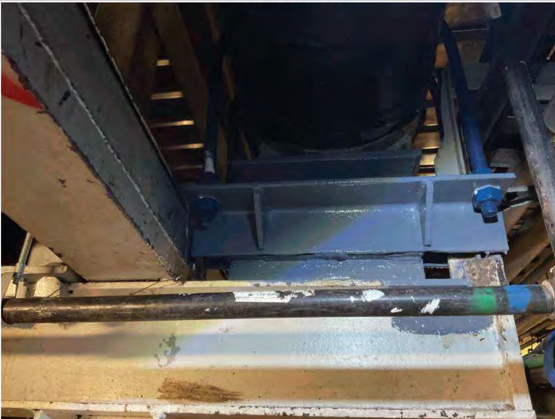
New welded bracket and U-bolt restraints existing Pipe Support 27.
