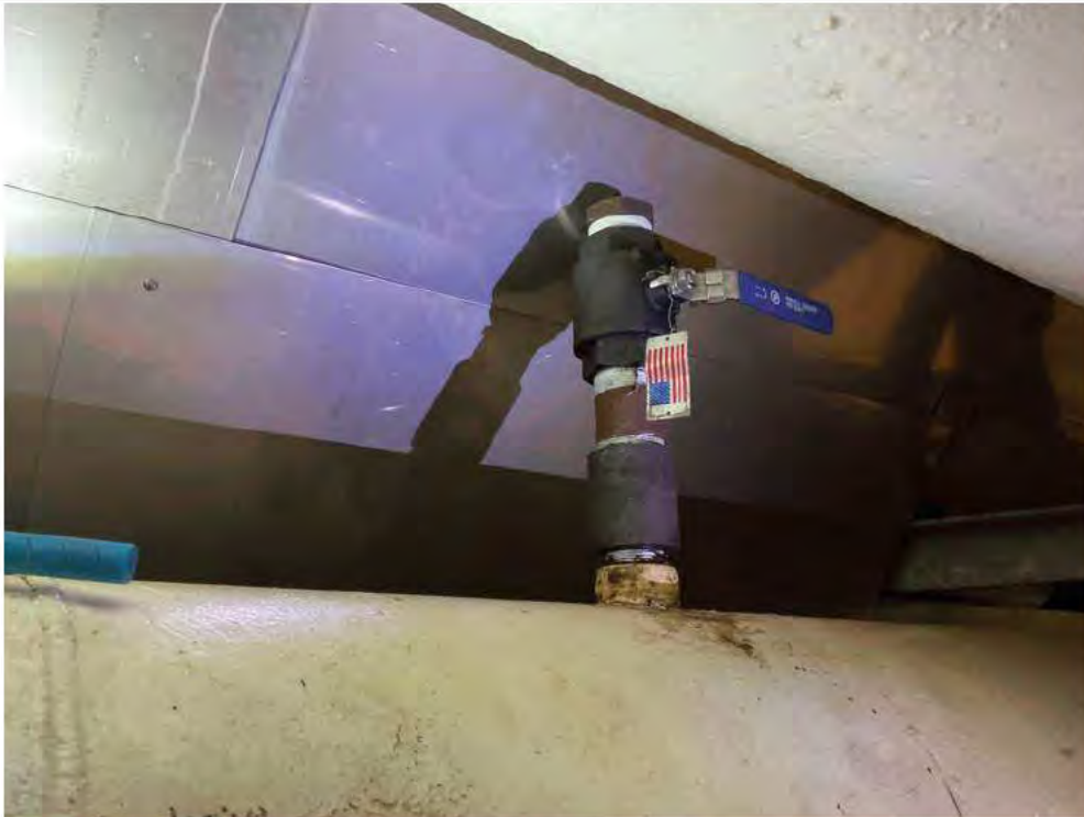
Threaded assembly replaced at PS 474.
