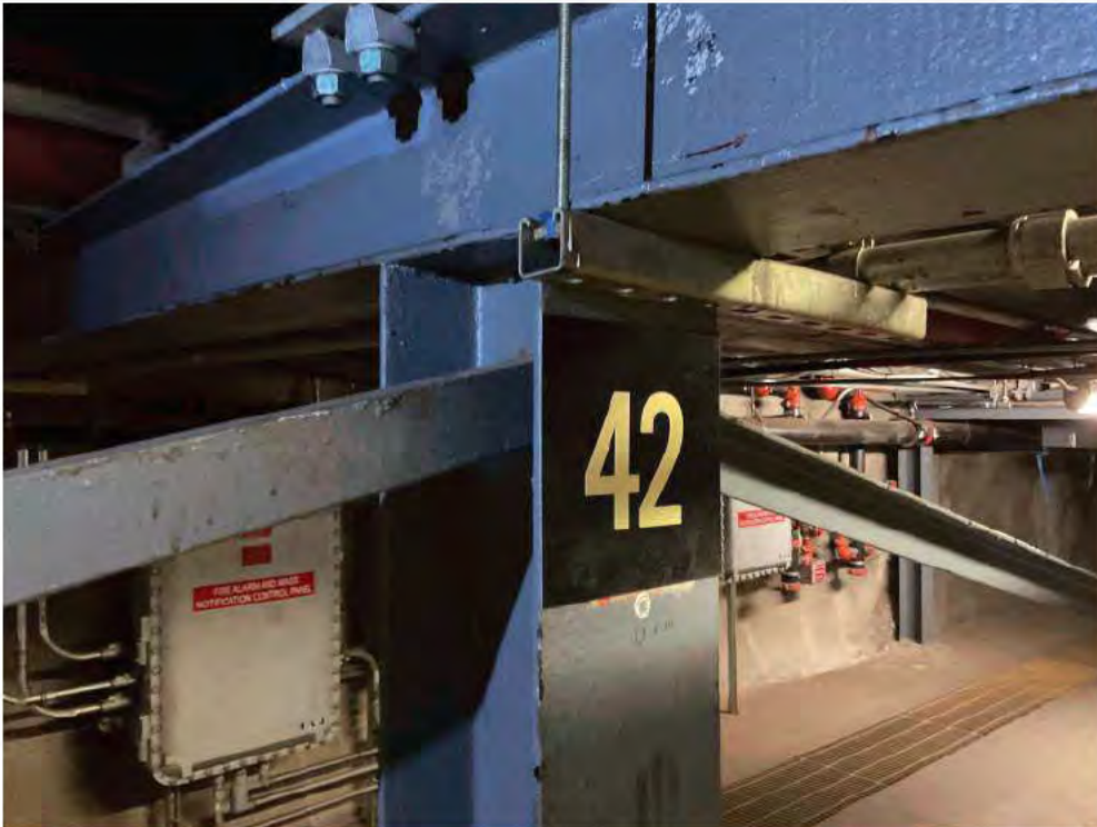
Existing Pipe Support 42.
