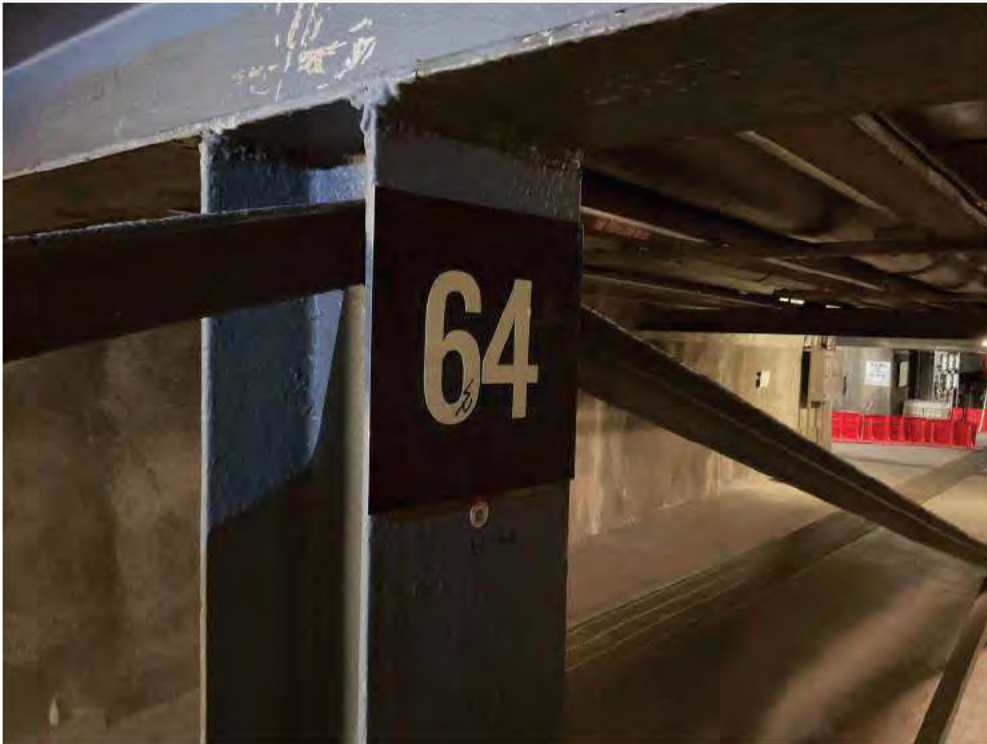
Existing Pipe Support 64.
