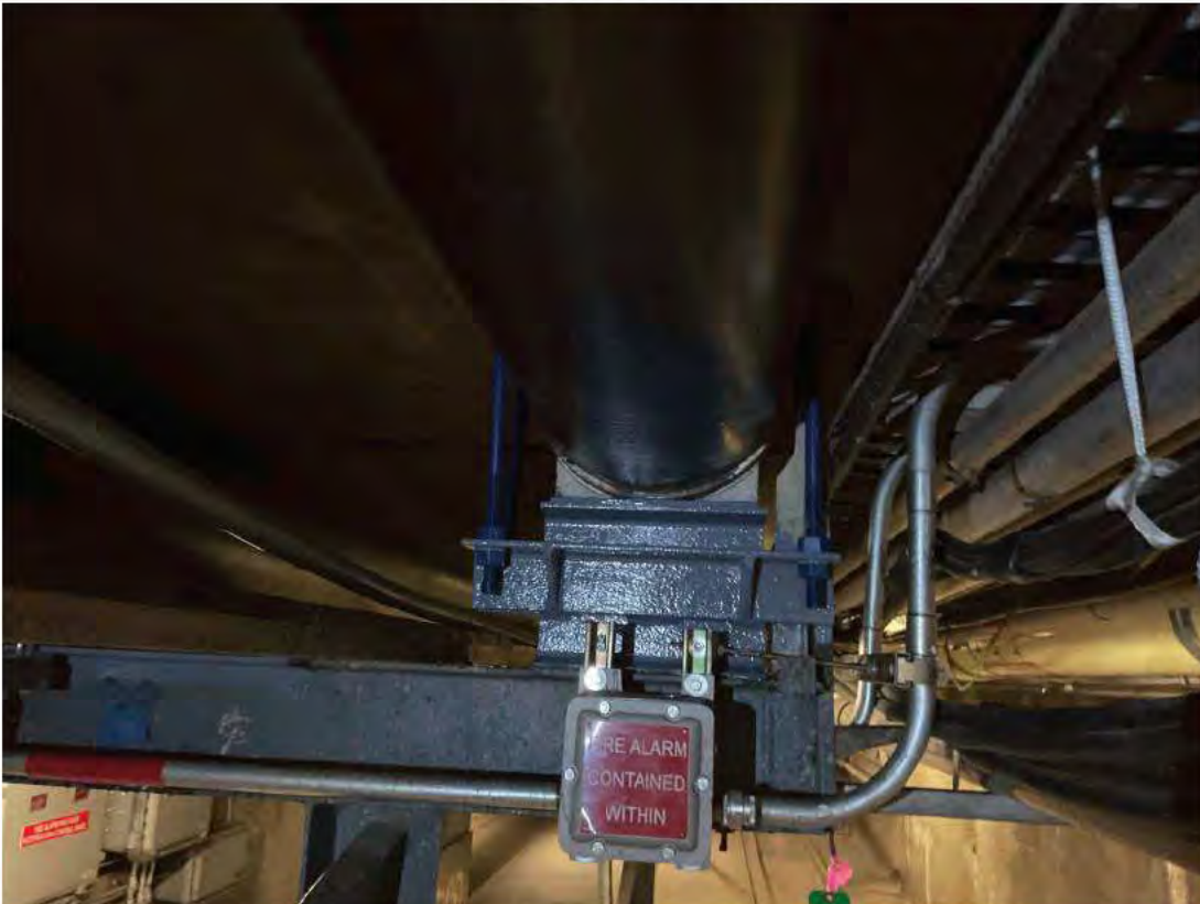
New welded bracket and U-bolt restraints at Pipe Support 60.
