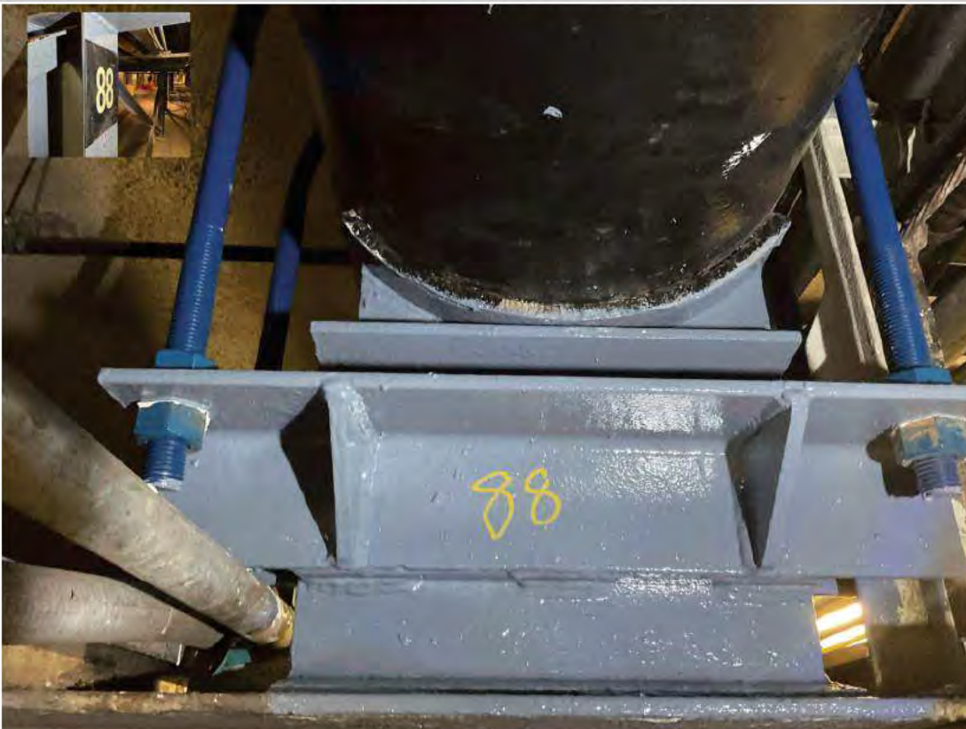
Re-seated and shimmed line at PS-88.
