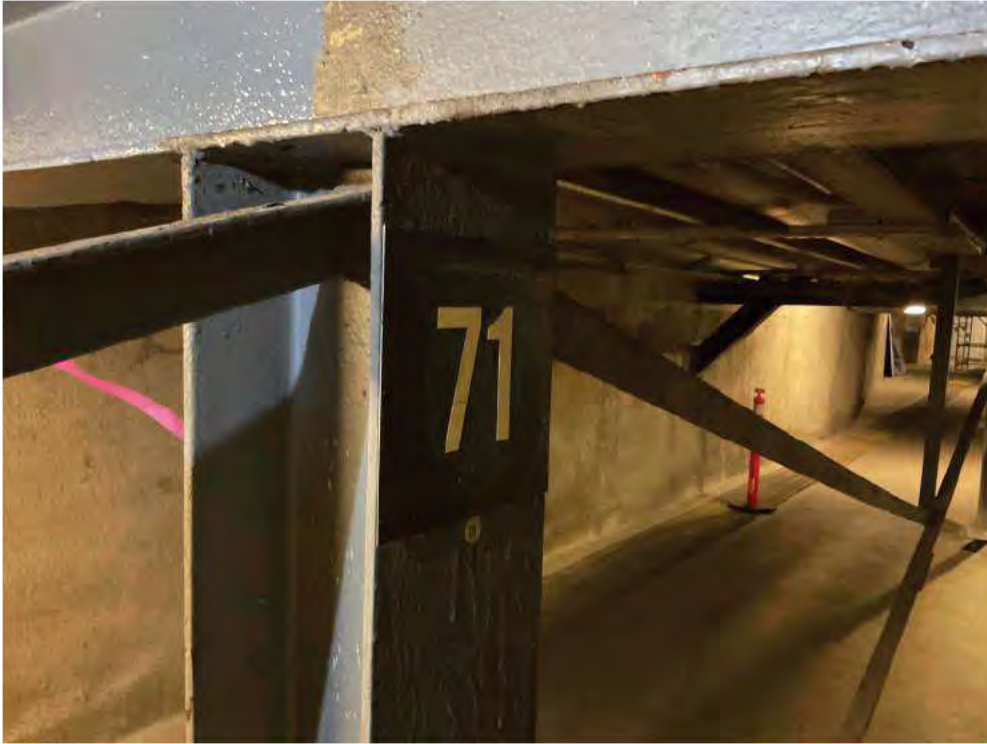
Existing Pipe Support 71.
