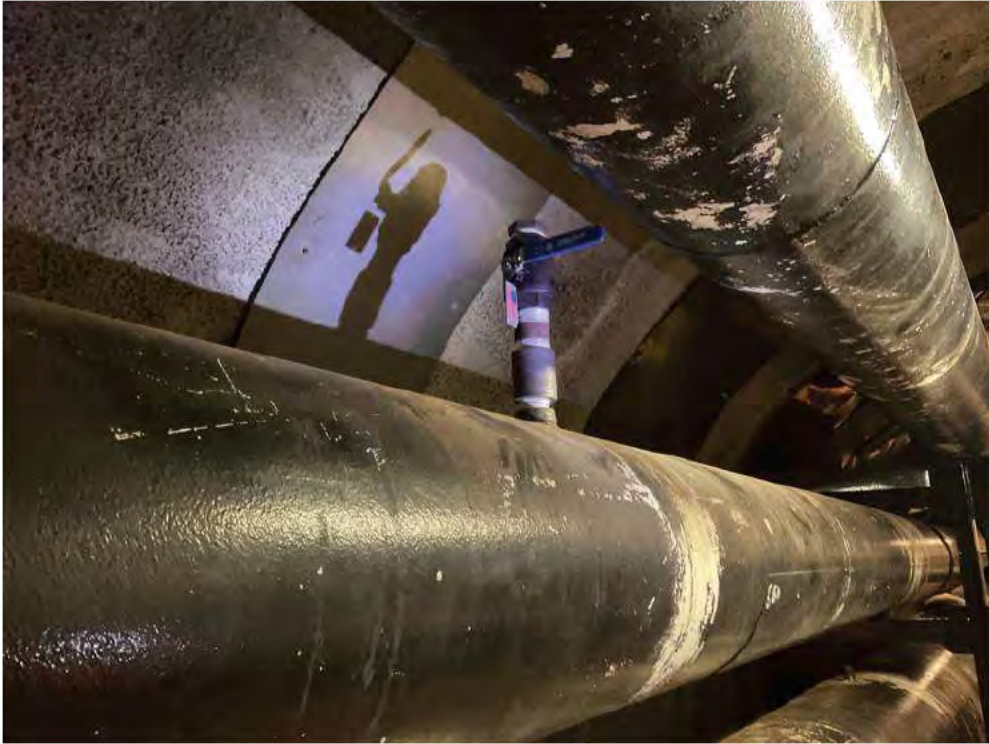
Threaded assembly replaced at PS 595 (2 of 2).
