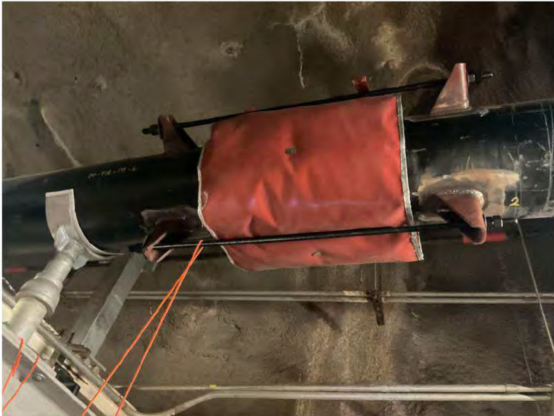
Repaired, reinstalled and re-wrapped Dresser coupling at Tank 18.
