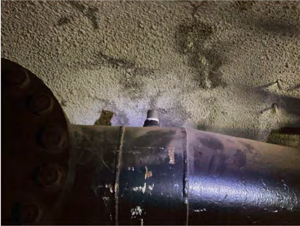
Replaced threaded plug at PS 650.
