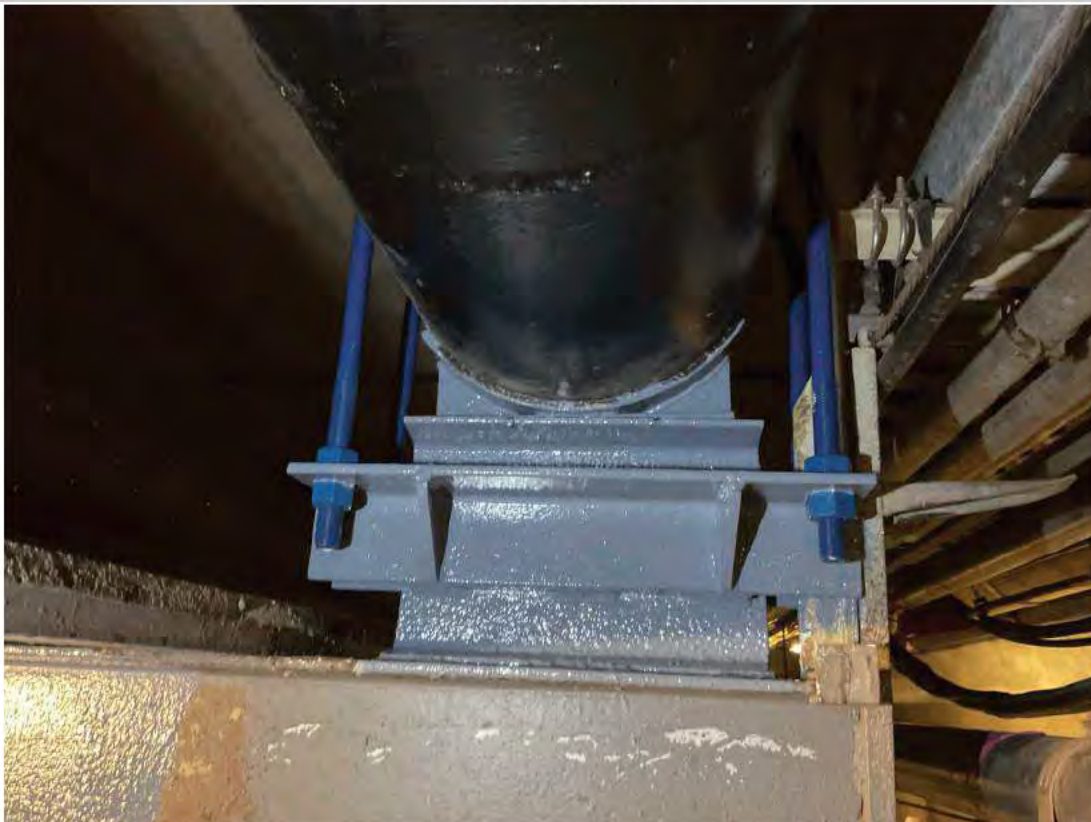
New welded bracket and U-bolt restraints at Pipe Support 71.
