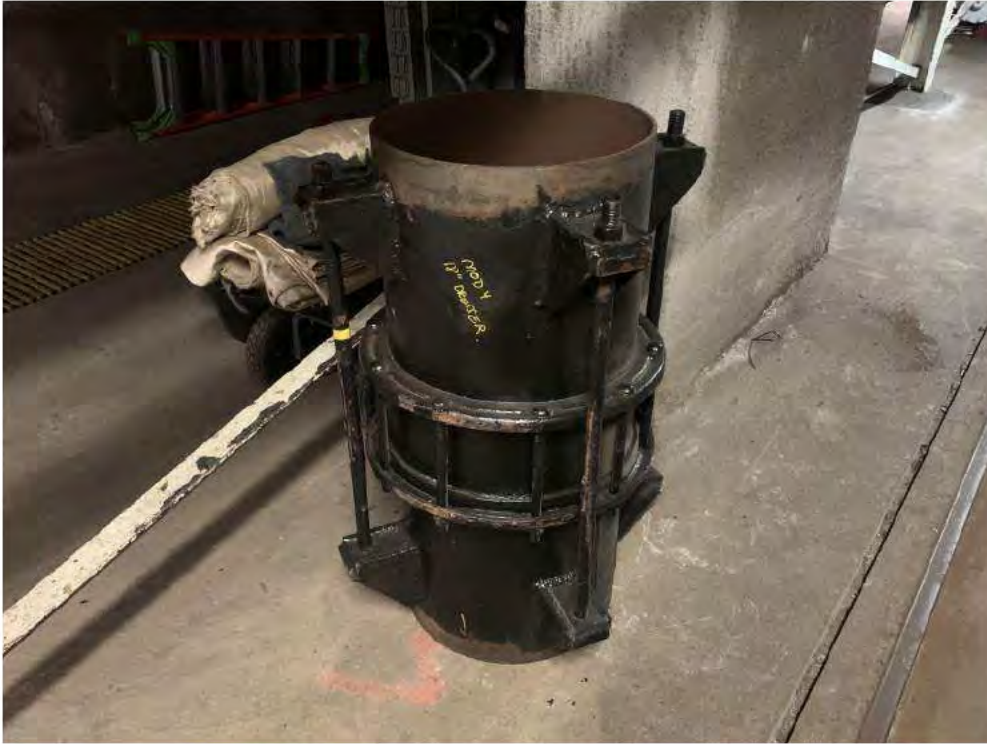
Mainline pipe compression sleeve coupling removed.
