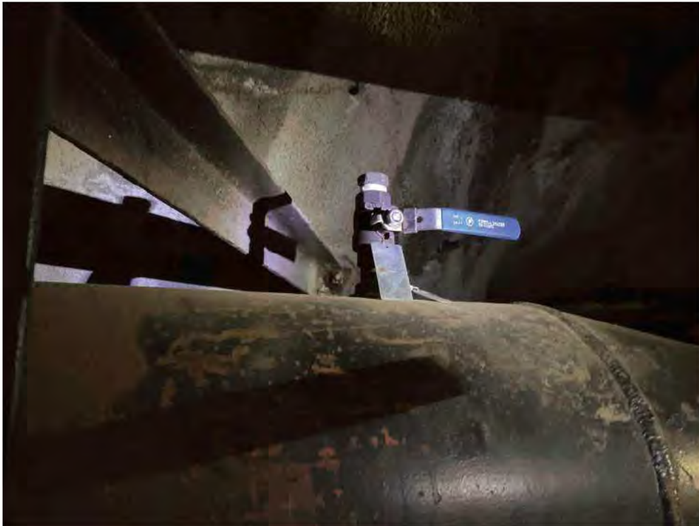
Threaded assembly replaced at PS 650.
