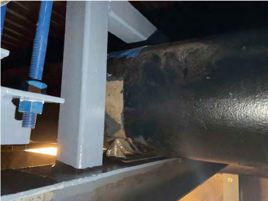
New welded bracket to prevent "escape" at existing Pipe Support 45.
