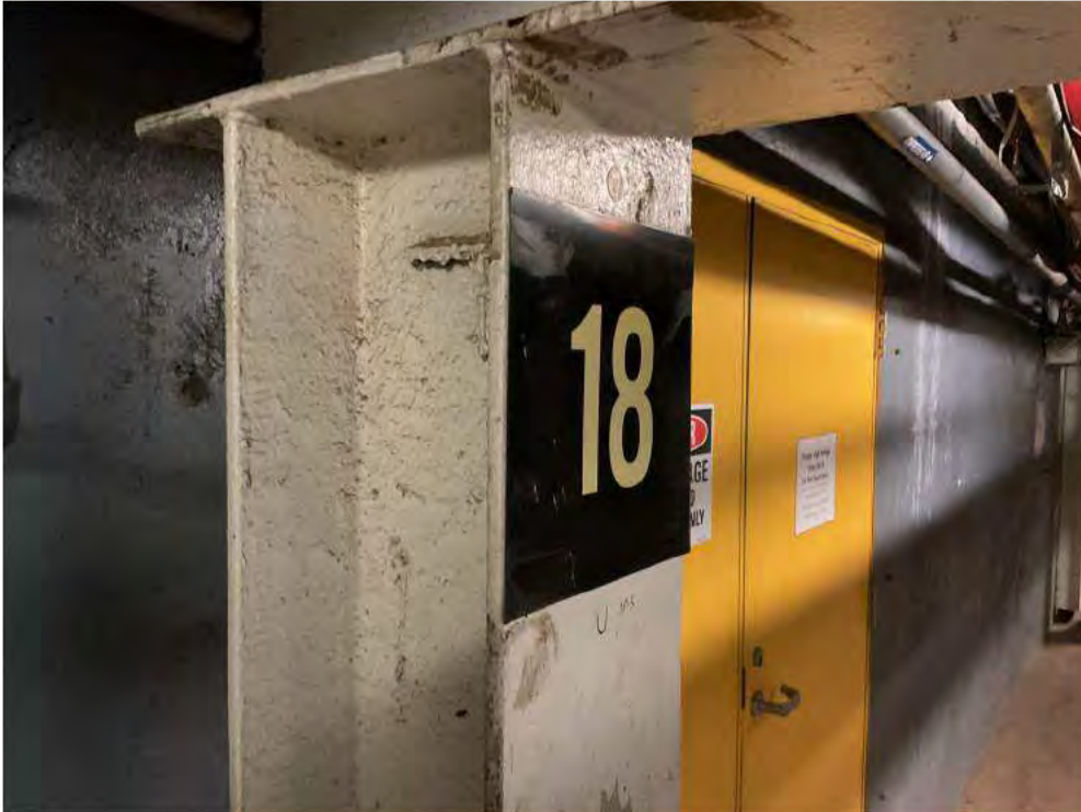
Existing Pipe Support 18.
