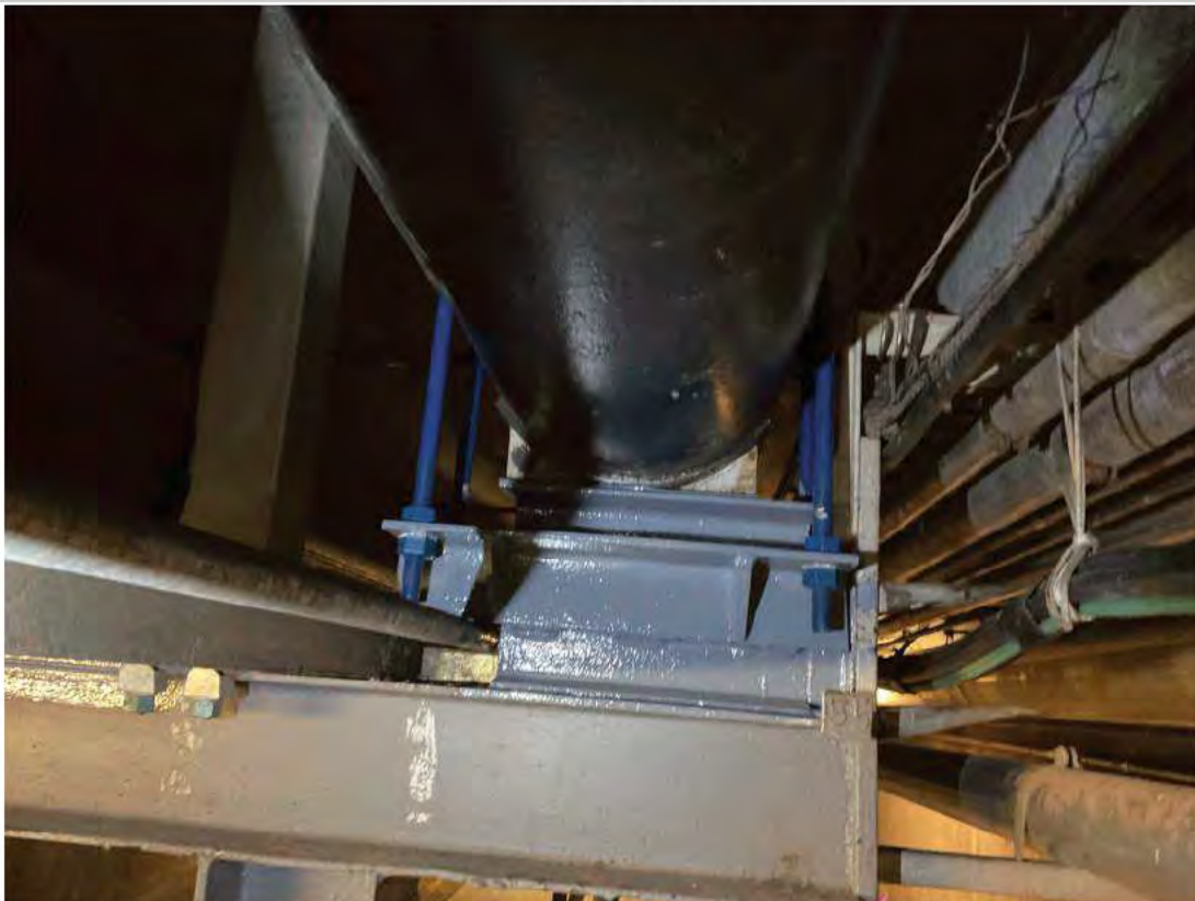
New welded bracket and U-bolt restraints at Pipe Support 55.
