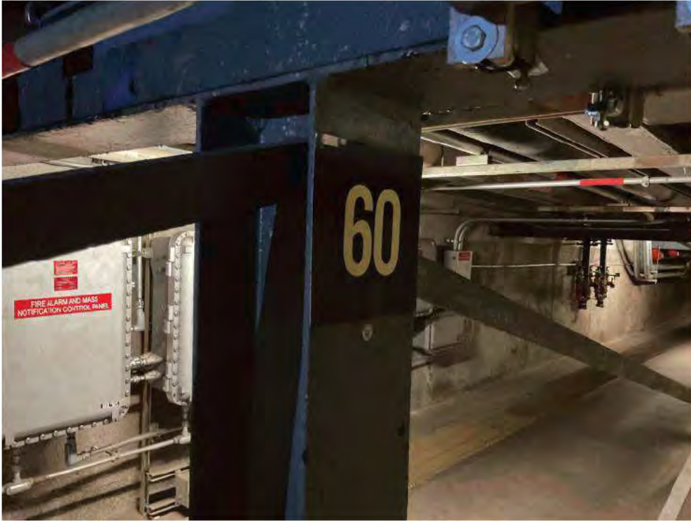
Existing Pipe Support 60.
