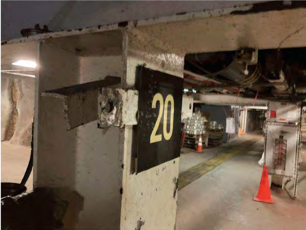
Existing Pipe Support 20.
