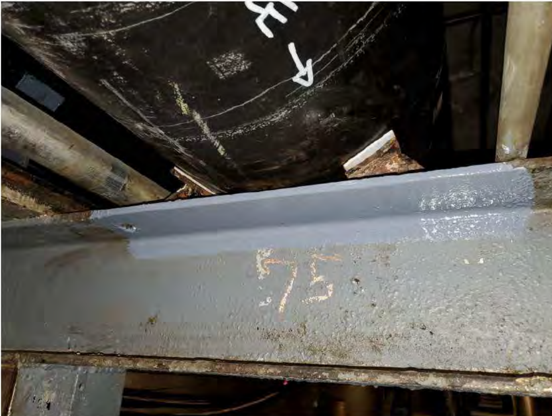
Repaired pipe cradle at Pipe Support 75.
