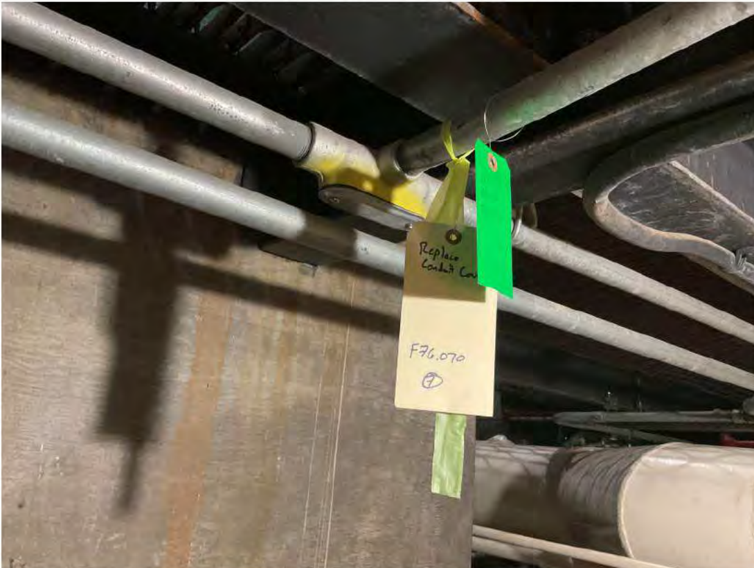
Form 5 conduit cover installation (typical) with QA tags.
