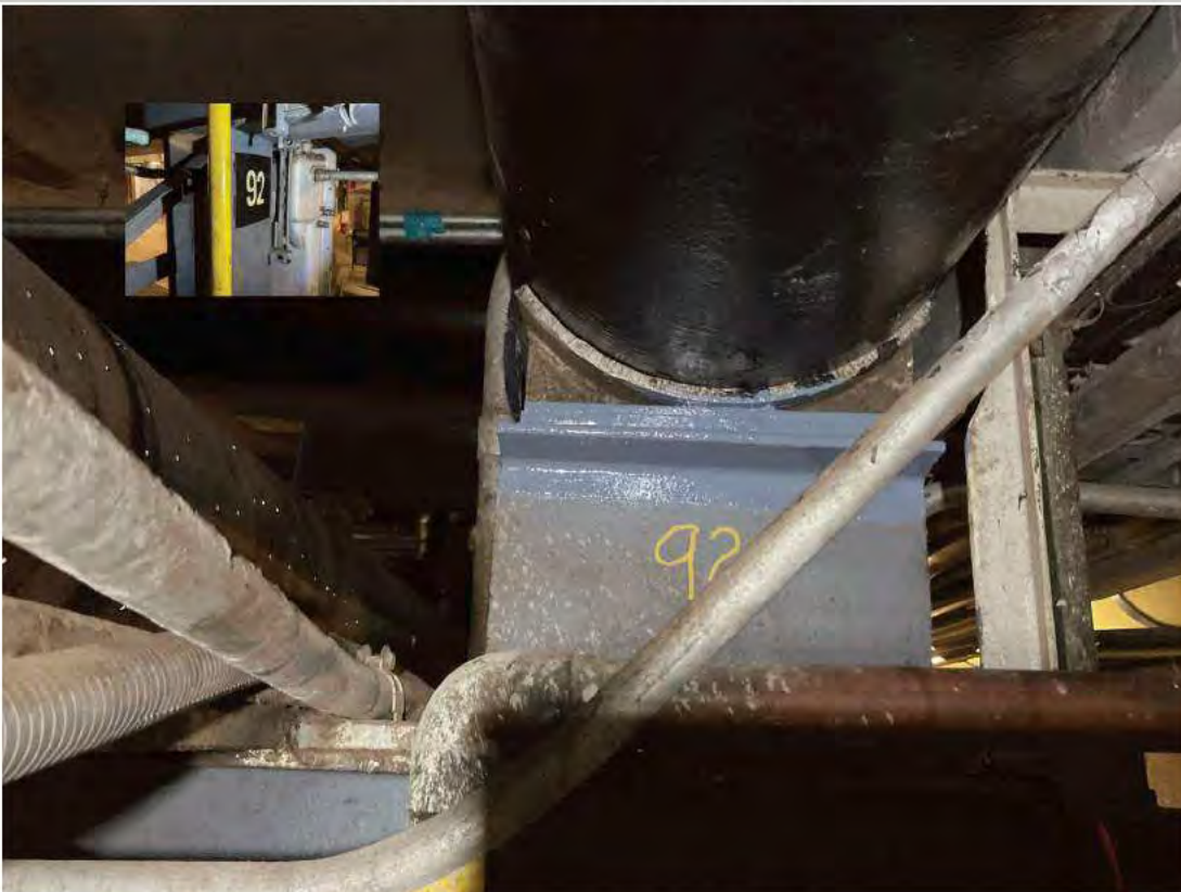
Re-seated and shimmed line at PS-92.
