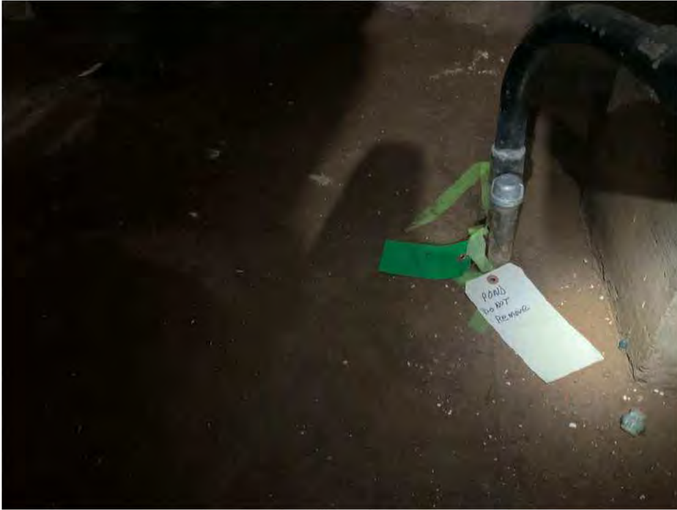
Cast iron round cap installation (typical) with QA tags.
