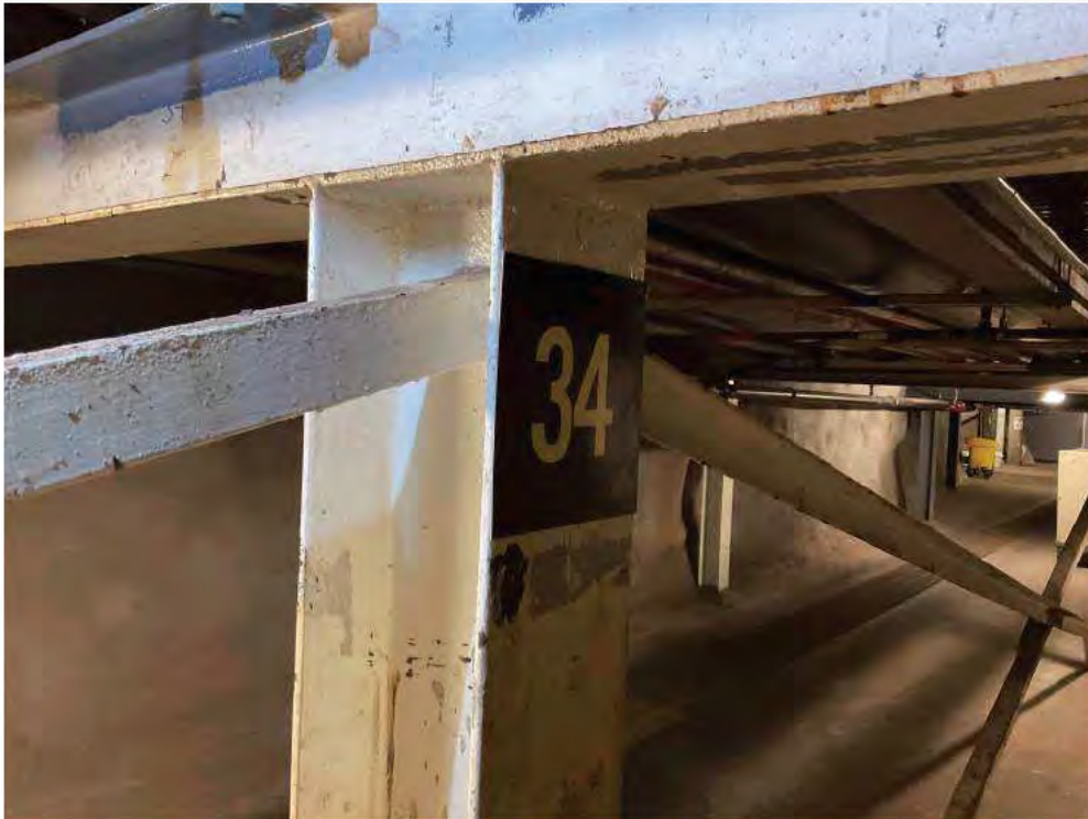
Existing Pipe Support 34.
