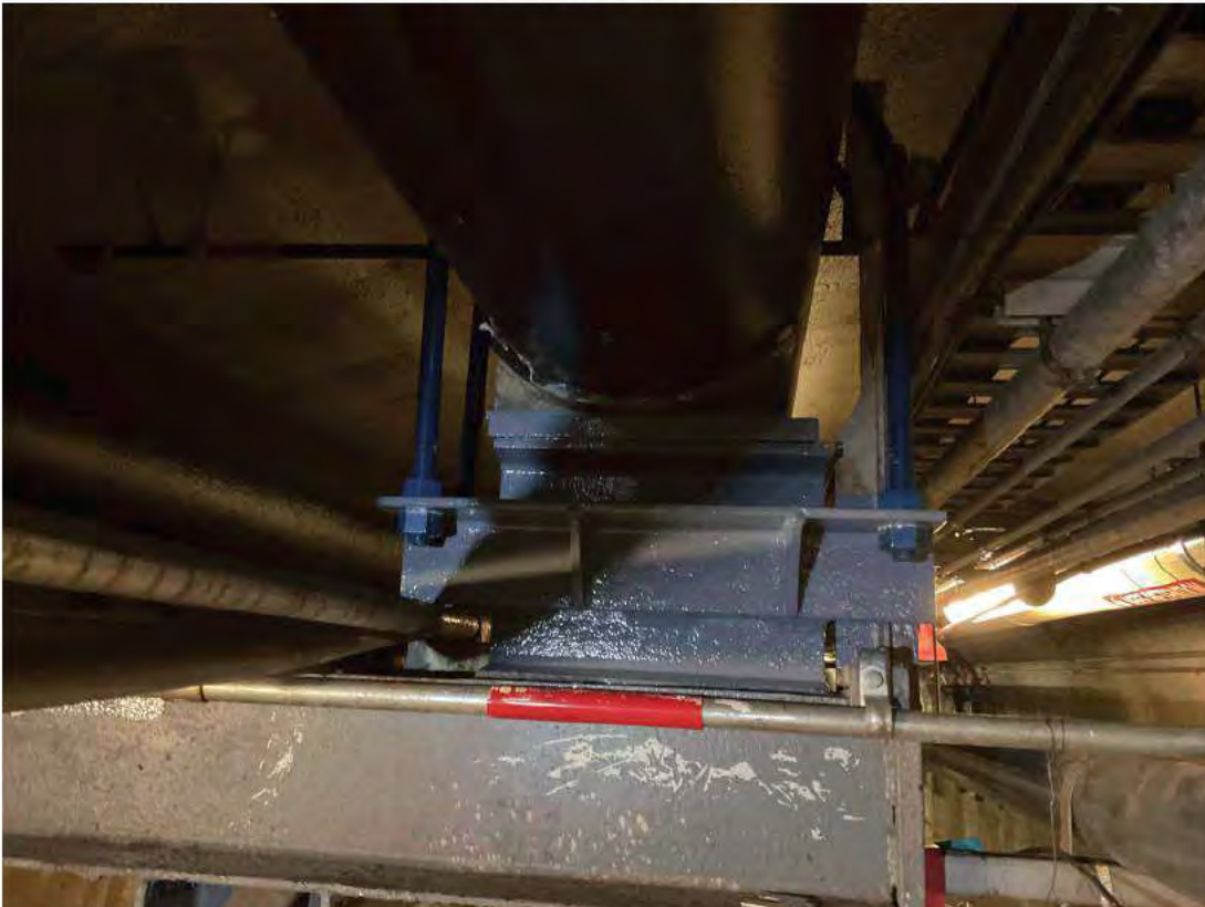
New welded bracket and U-bolt restraints existing Pipe Support 85.
