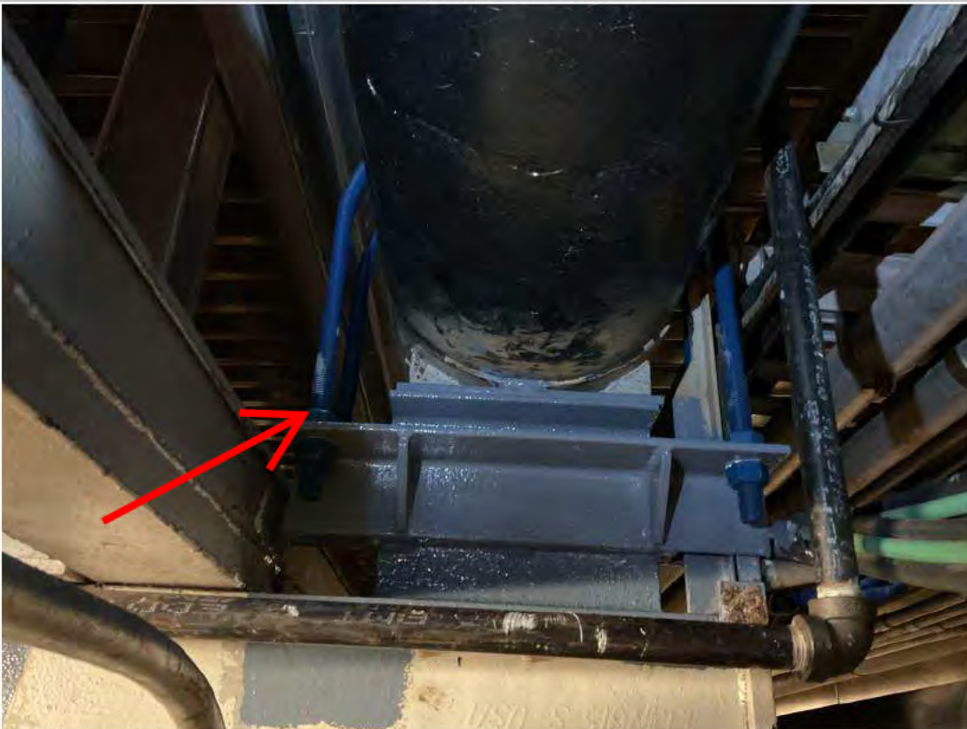
New welded bracket and U-bolt restraints existing Pipe Support 23.
