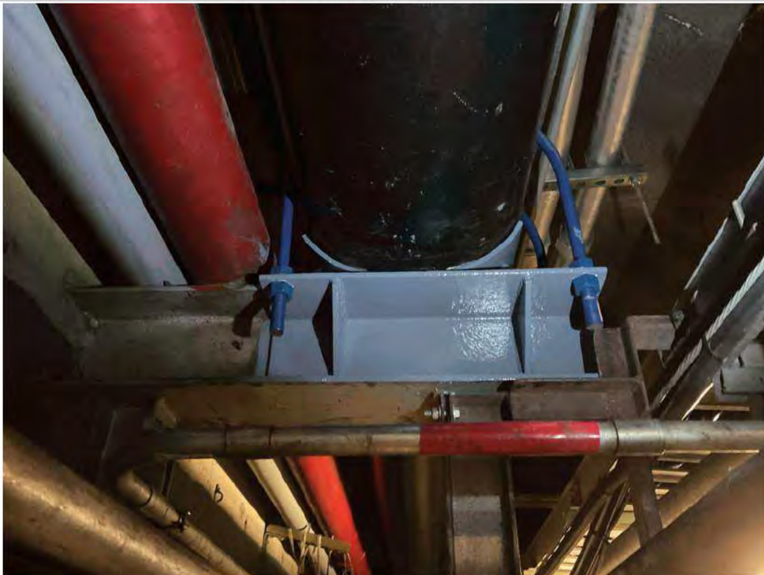
New welded bracket and U-bolt restraints existing Pipe Support 19.
