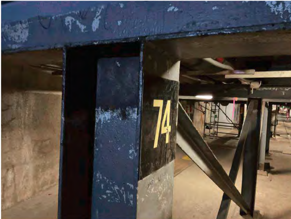
Existing Pipe Support 74.
