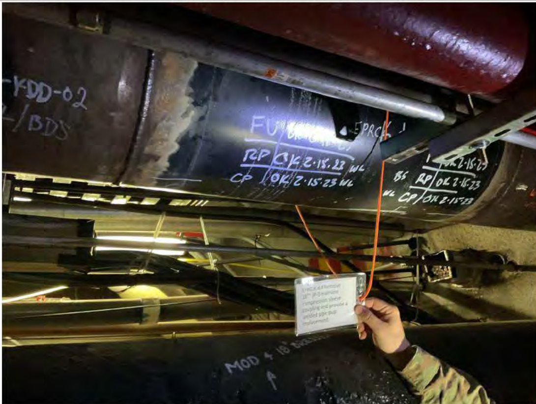
Welded pup segment installed in place of pipe compression sleeve coupling.
